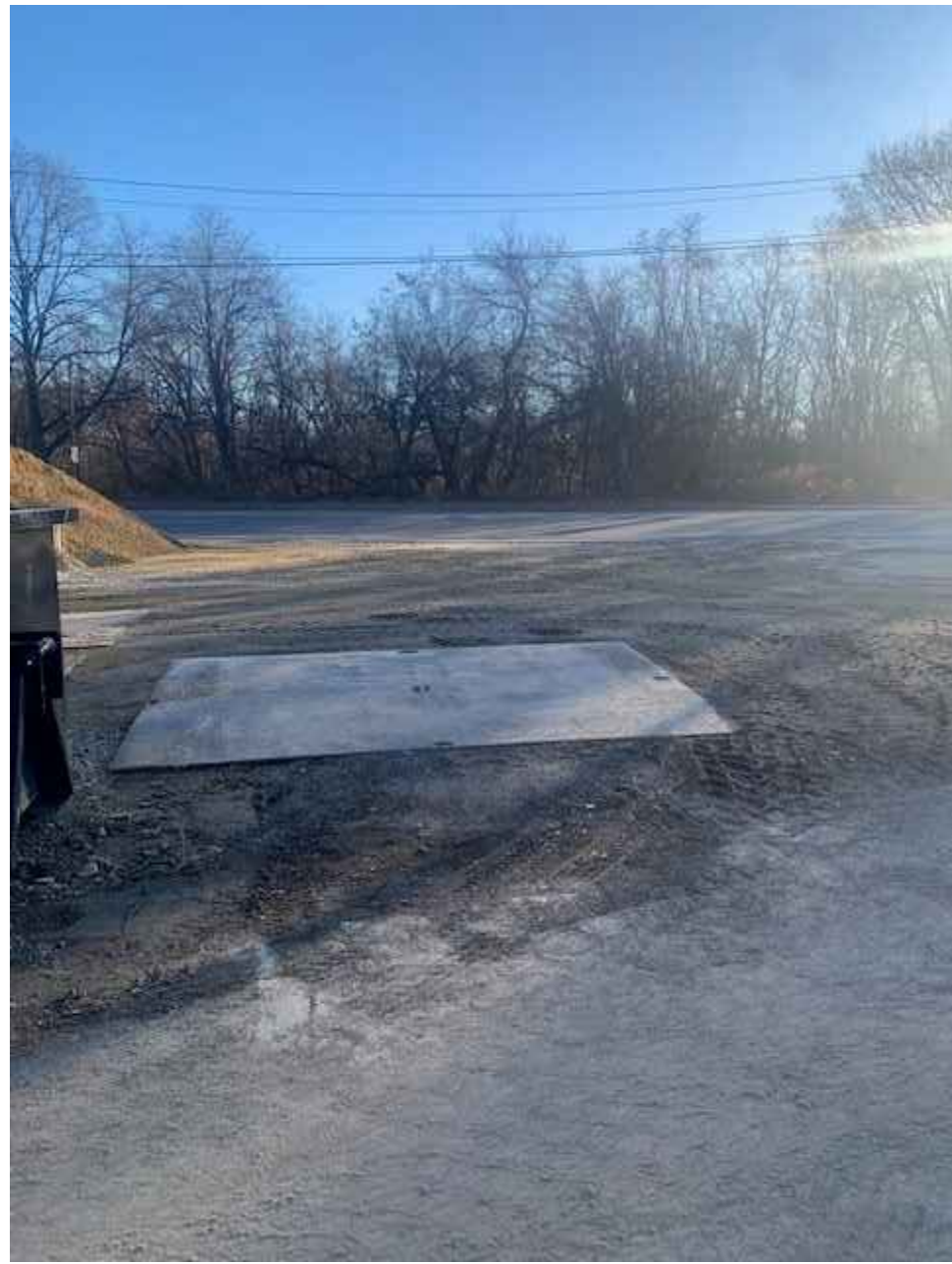
PHOTO 5: TAKEN FROM SOUTHERN PORTION OF BIKE PATH LOOKING SOUTH
