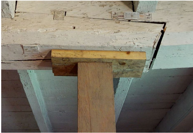
Support and crack monitor
