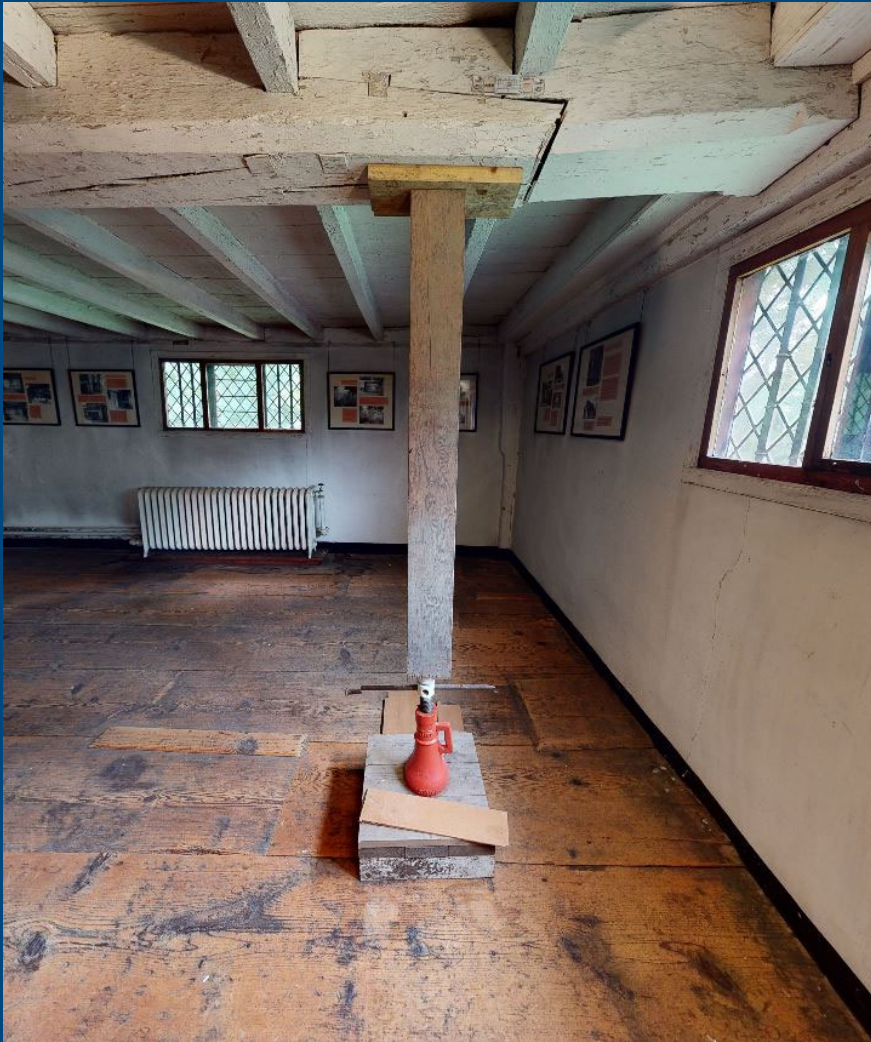
Temporary post shore on the second floor
