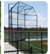
Renovated Baseball Backstop
