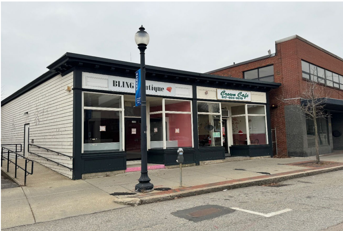
3. 104-106 Main Street north (facade) elevation. Facing west.
