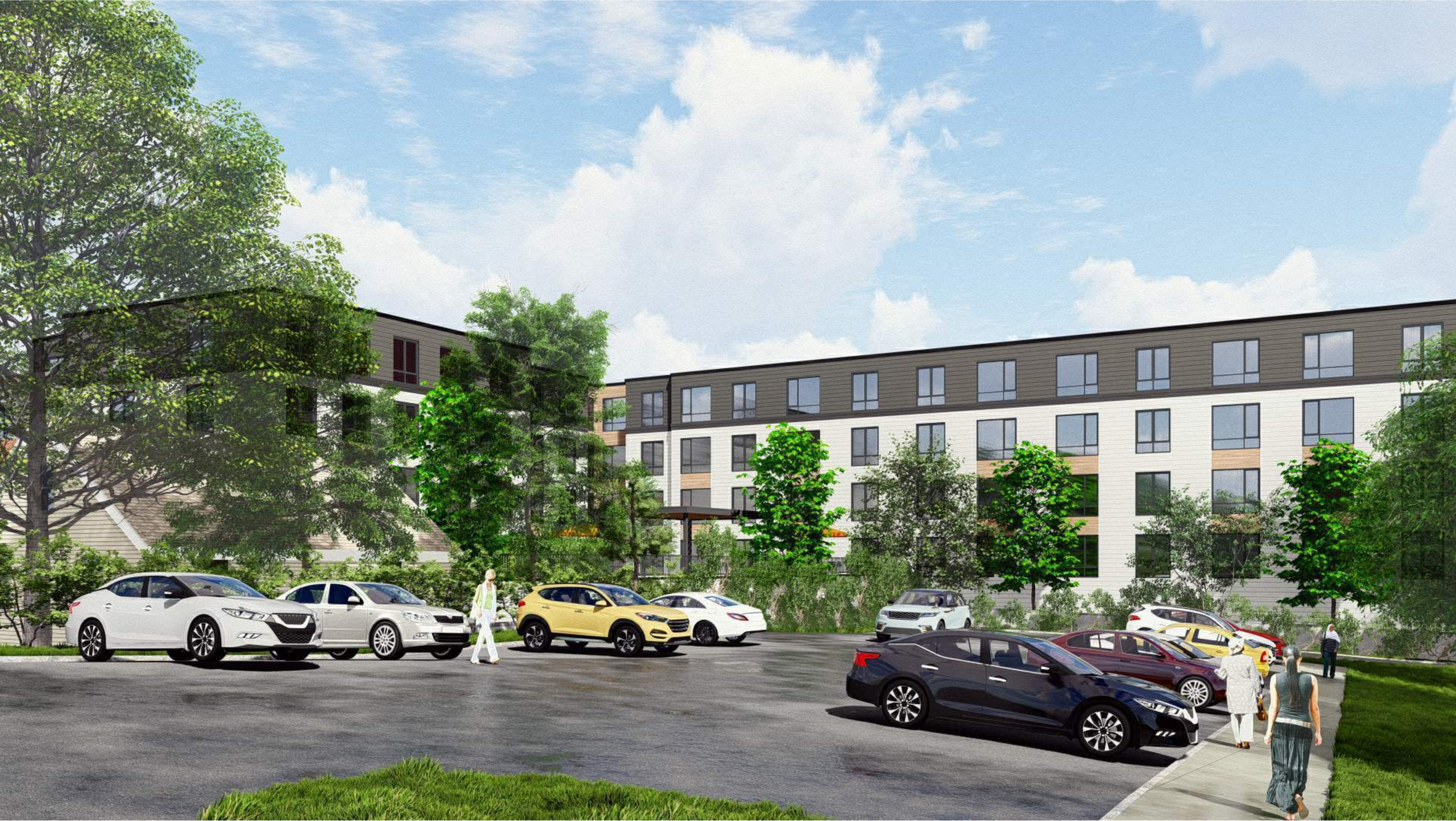
VIEW ALONG CHURCH HILL ST.
