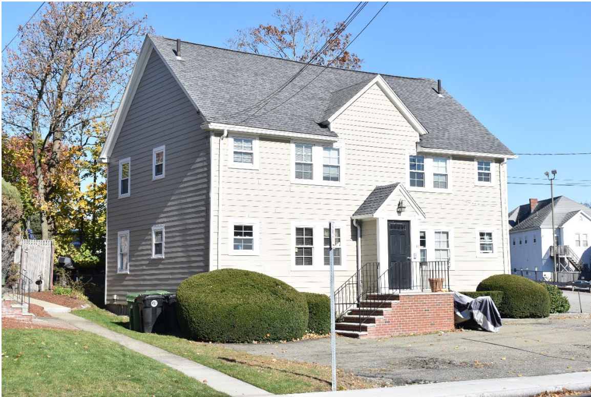
1. 53 Pleasant Street, west and south (facade) elevations. Facing northwest
