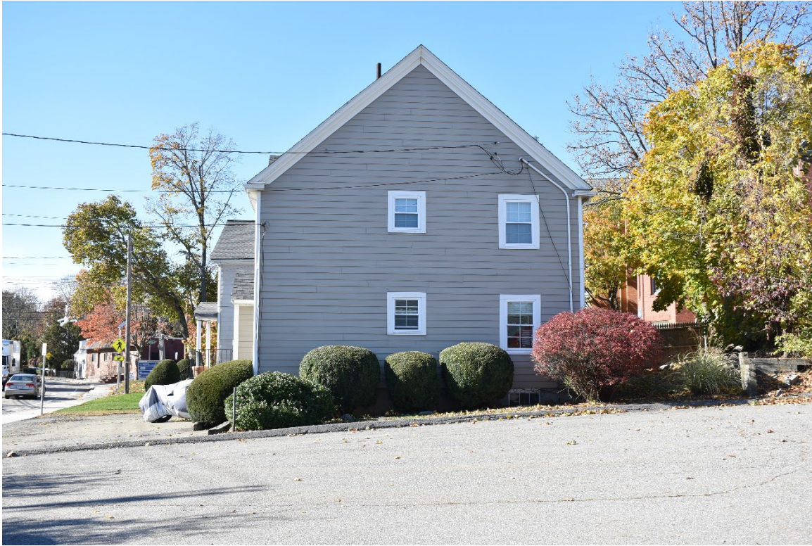
3. 53 Pleasant Street, east side elevation. Facing west.
