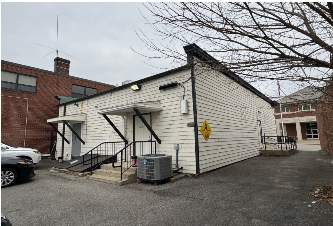
4. Rear (south) and side (east) elevation of 104-106 Main Street from parking lot. Facing north.
