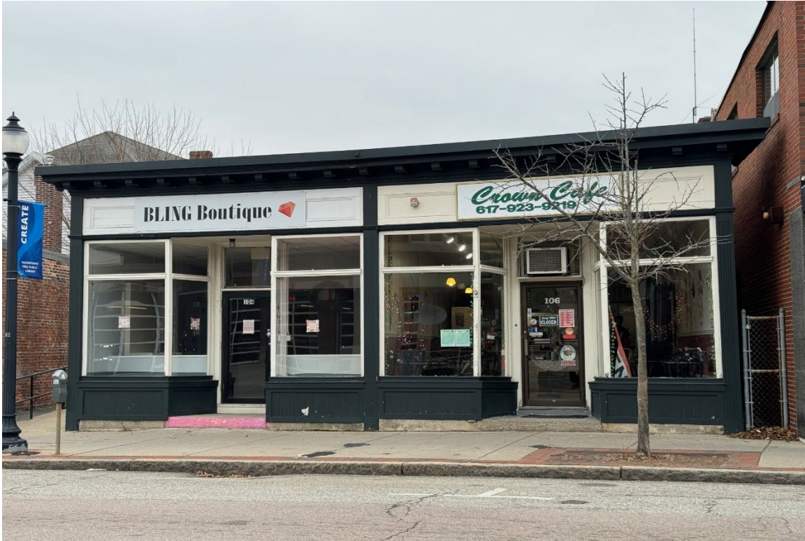
1. 104-106 Main Street north (facade) elevation. Facing southwest.
