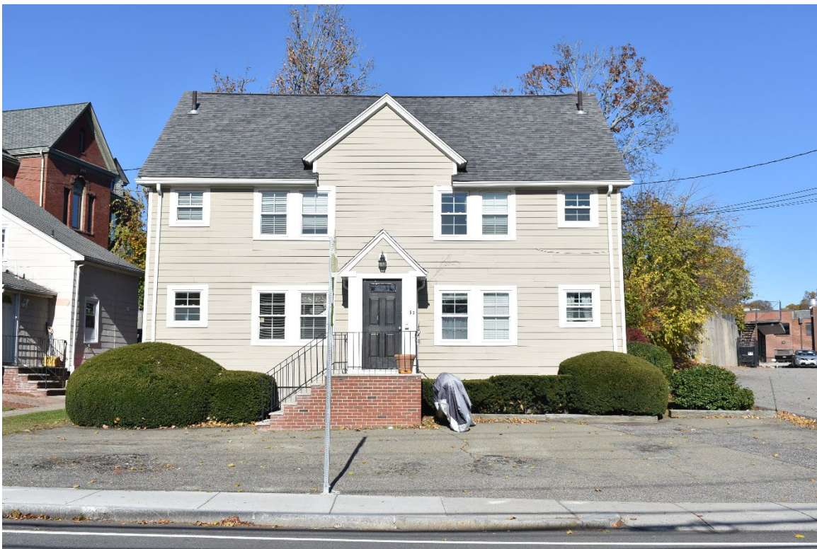
2. 53 Pleasant Street, south (facade) elevation. Facing north.
