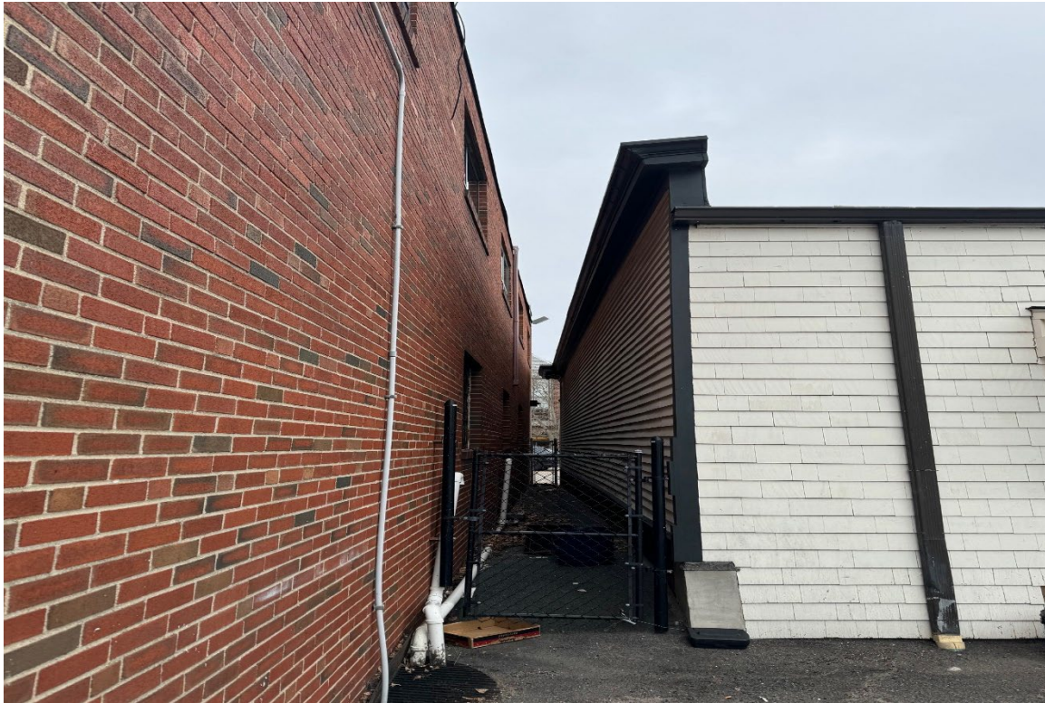
5. Side (west) elevation of 104-106 Main Street. Facing northeast.
