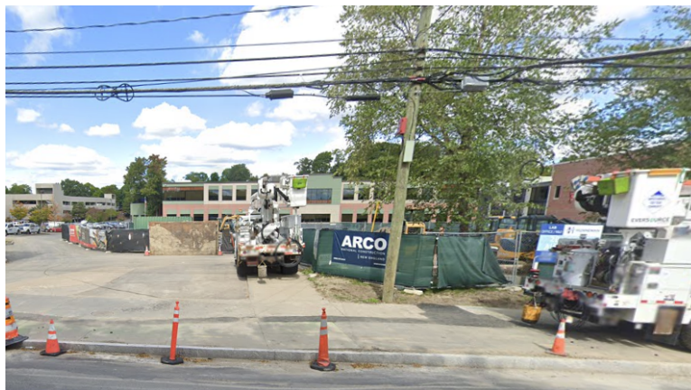
View of UP#5/46 on Arsenal Street at the property line of 101 Walnut Street where conduit is proposed.
