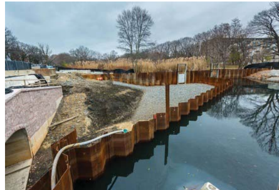
During construction - in-water cofferdam allows fish bypass.
