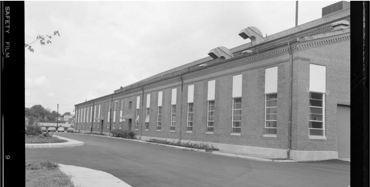
EXTERIOR VIEW FROM SOUTH-EAST - CA. 1967–1984
