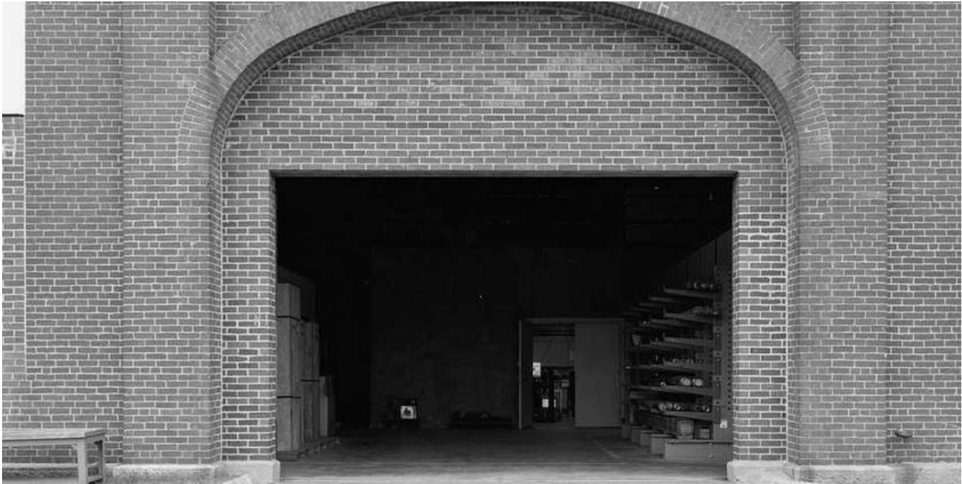
EXTERIOR VIEW FROM NORTH ARC ENTRYWAY CA. 1967-1984
