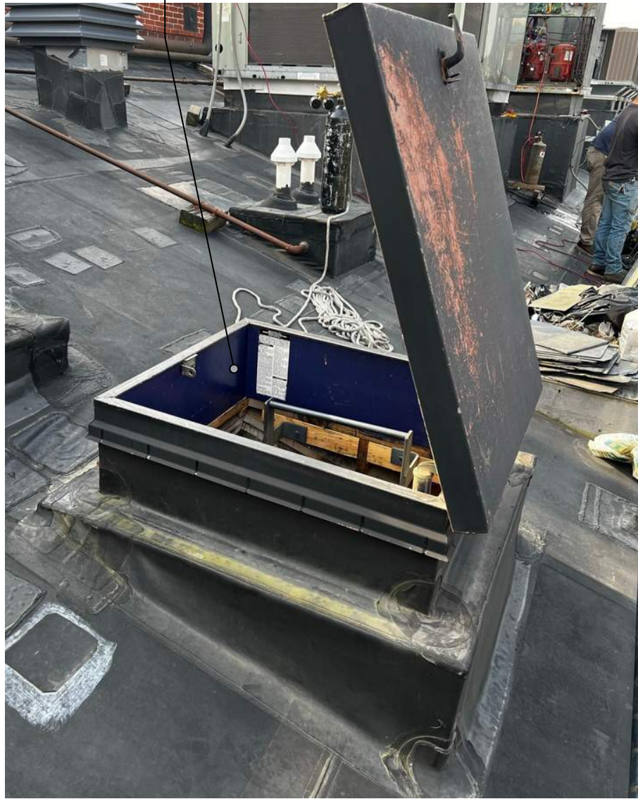
B) EXISTING SHIPS LADDER HATCH
