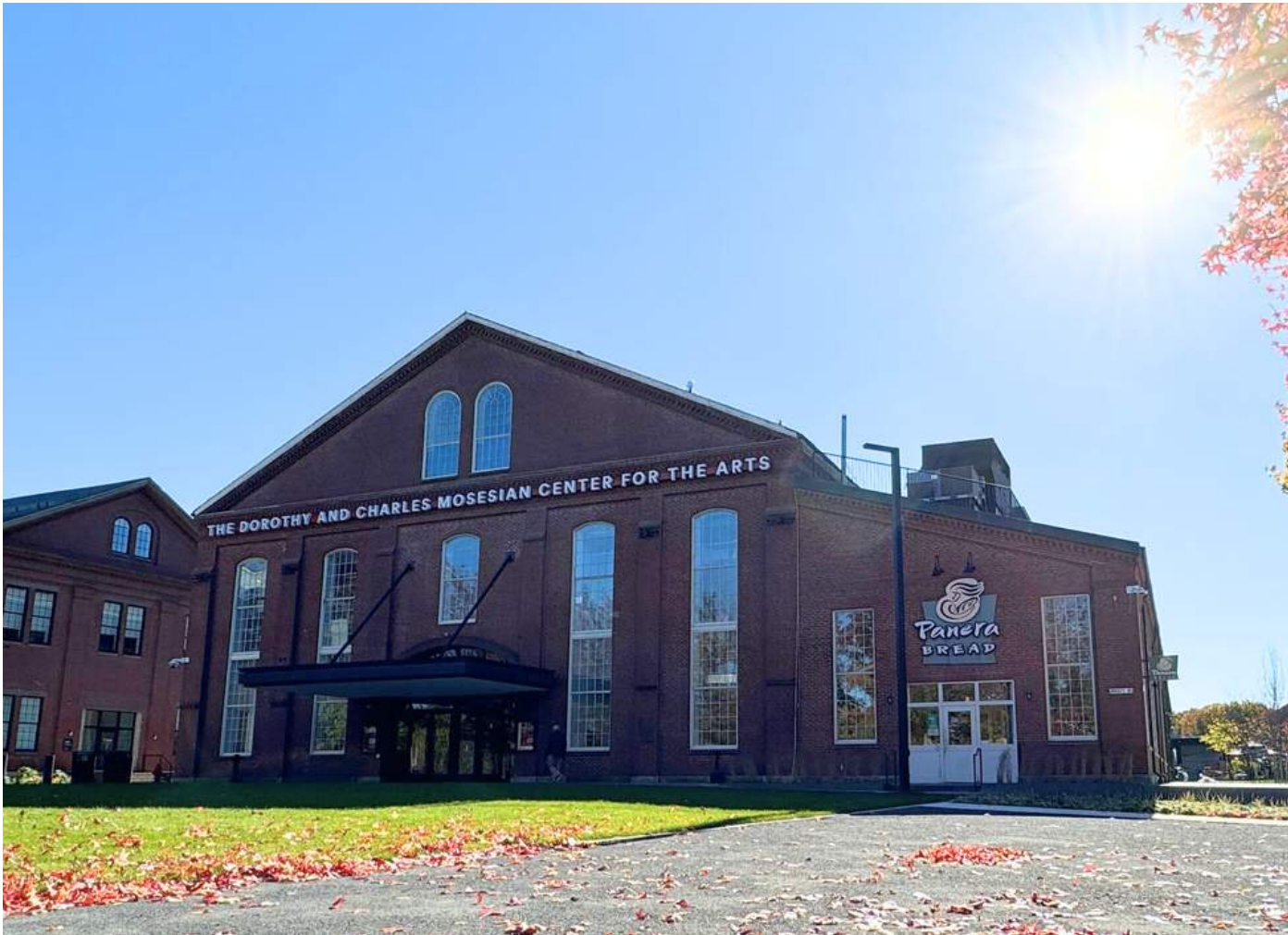
A| VIEW FROM NORTH
