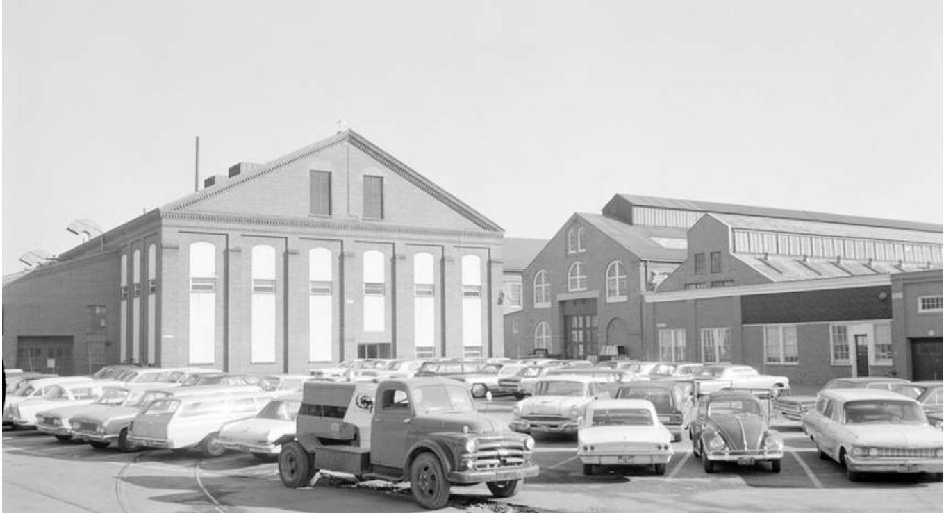
EXTERIOR VIEW FROM SOUTH - CA. 1967-1984
