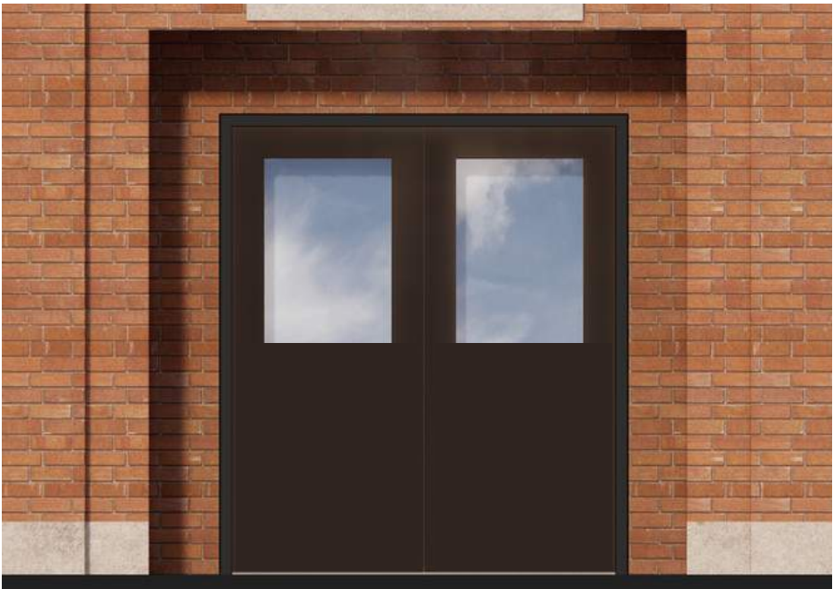
SOUTH FACADE NEW DOOR
