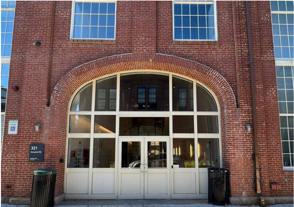
ARC ENTRYWAY EAST FACADE - EXISTING
