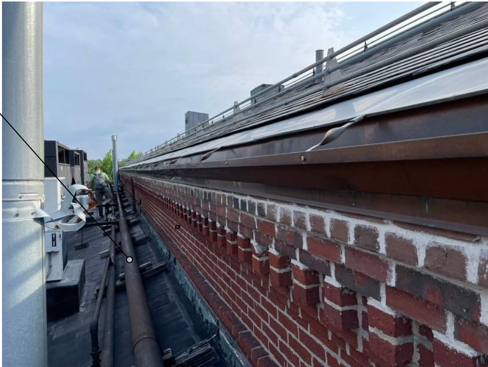
C) EXISTING PIPING UPPER SIDE ROOF
