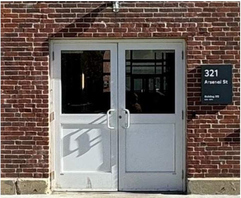
WEST FACADE DOOR- EXISTING
