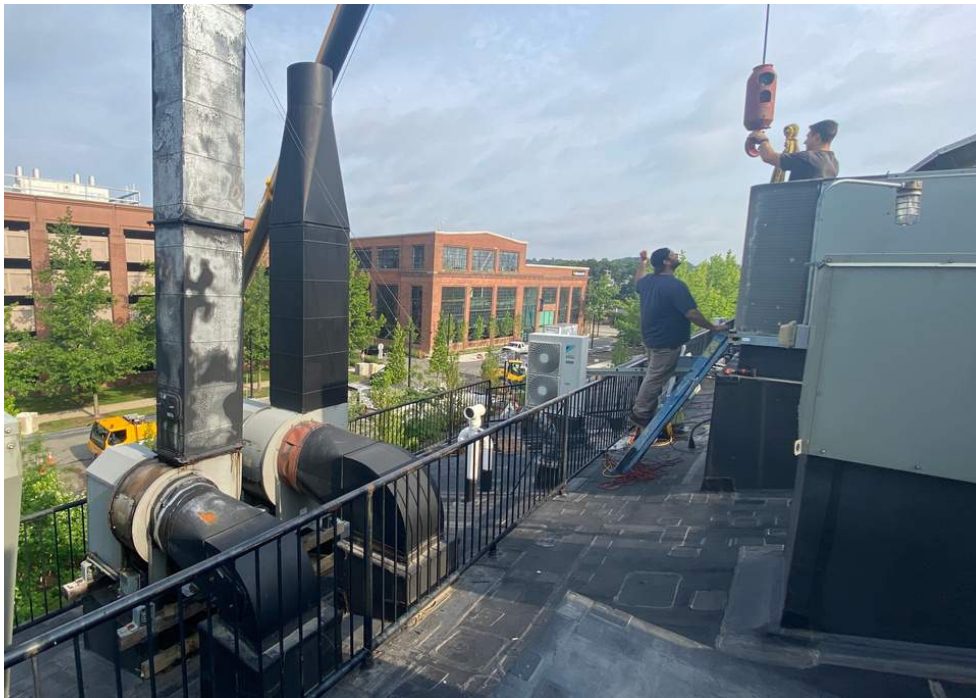
D) EXISTING ROOF CONDITIONS
