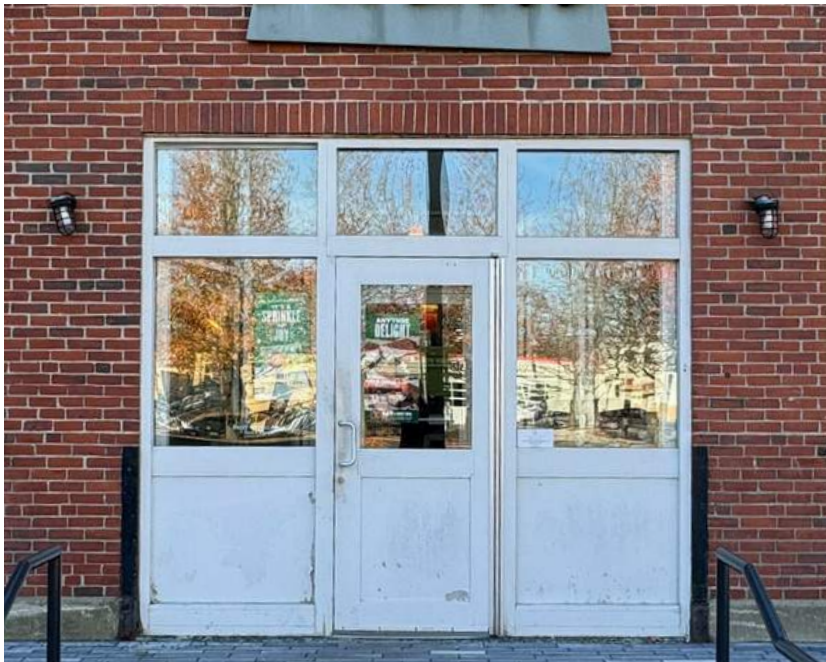
A1) NORTH ENTRYWAY - EXISTING
