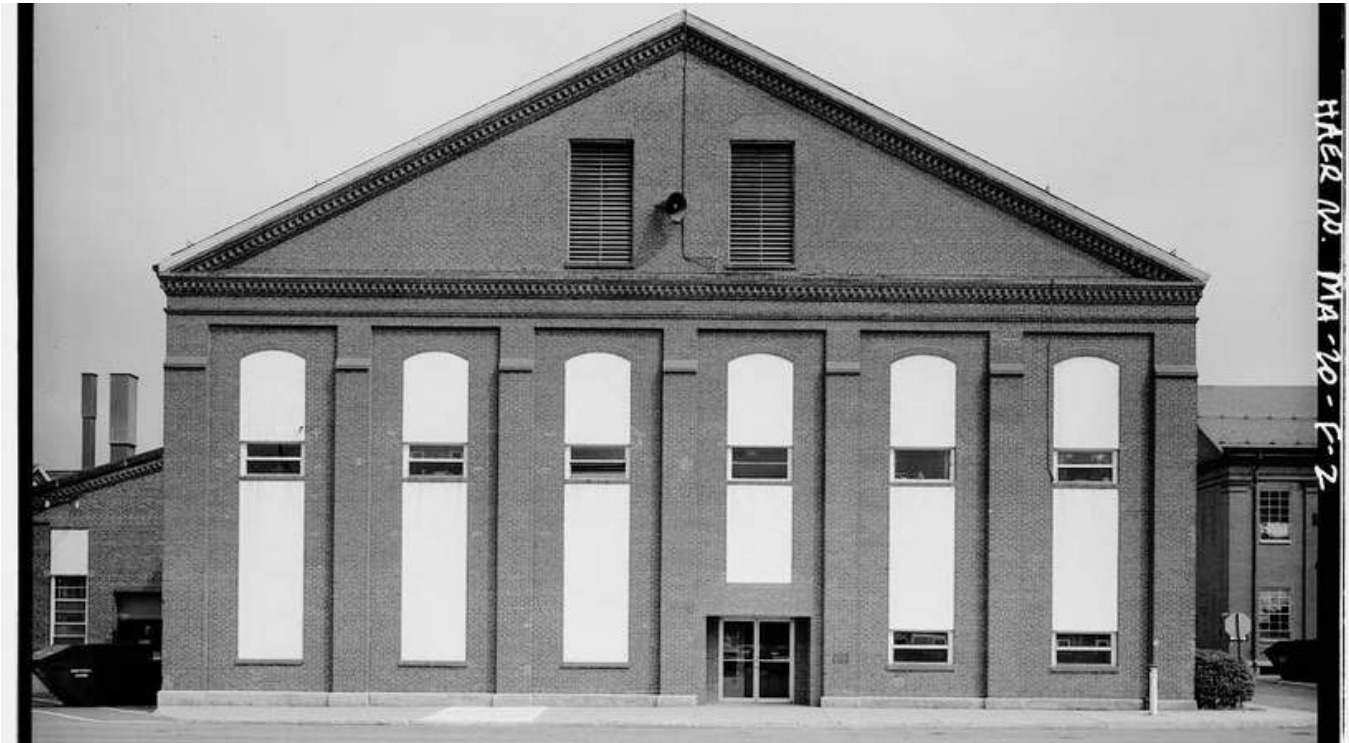
EXTERIOR VIEW FROM SOUTH - CA. 1967–1984
