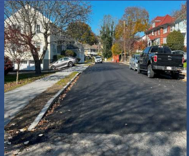
East Bates Road - After
