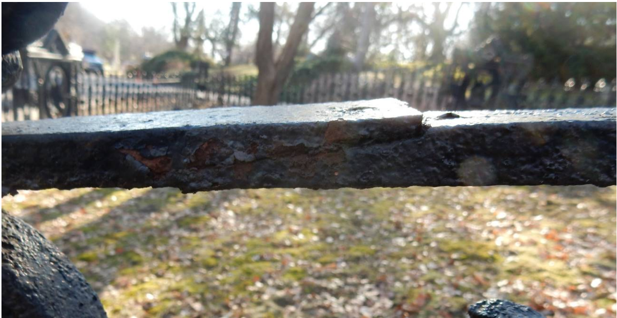
Photo 19 (Example of top rail splice)
