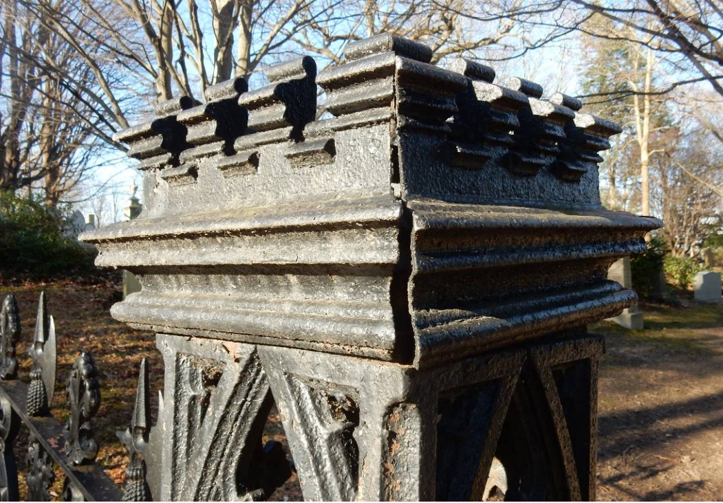
Photo 52 (Post C, example of separated cast iron elements and elements out of alignment)
