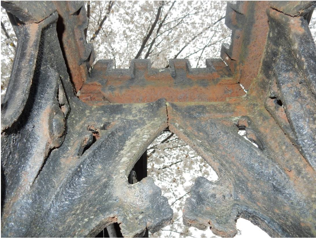
Photo 40 (Example of rust damage)
