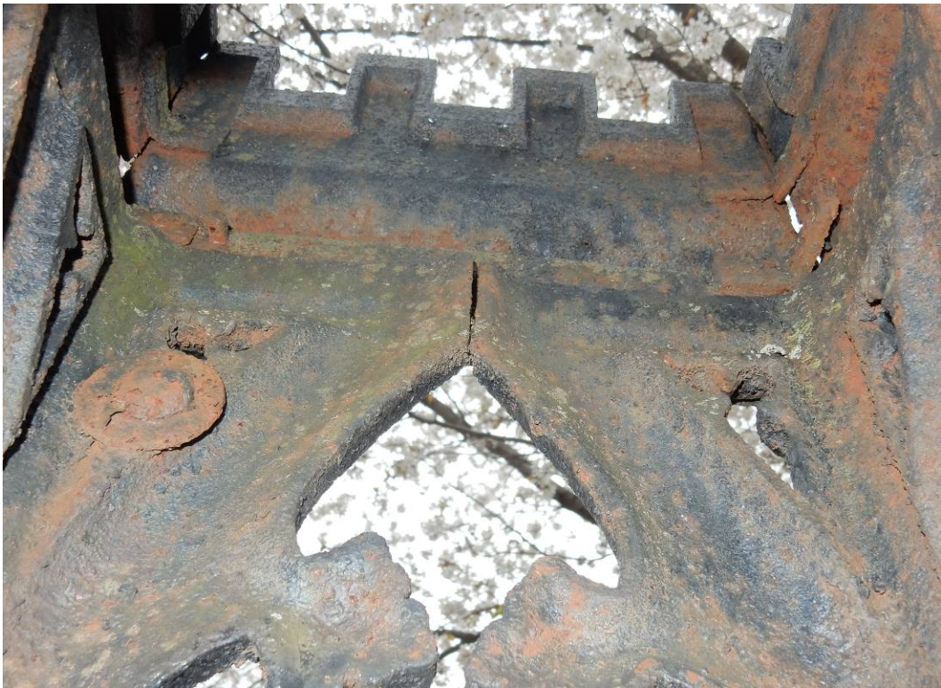
Photo 42 (Example of rust and rust damage)
