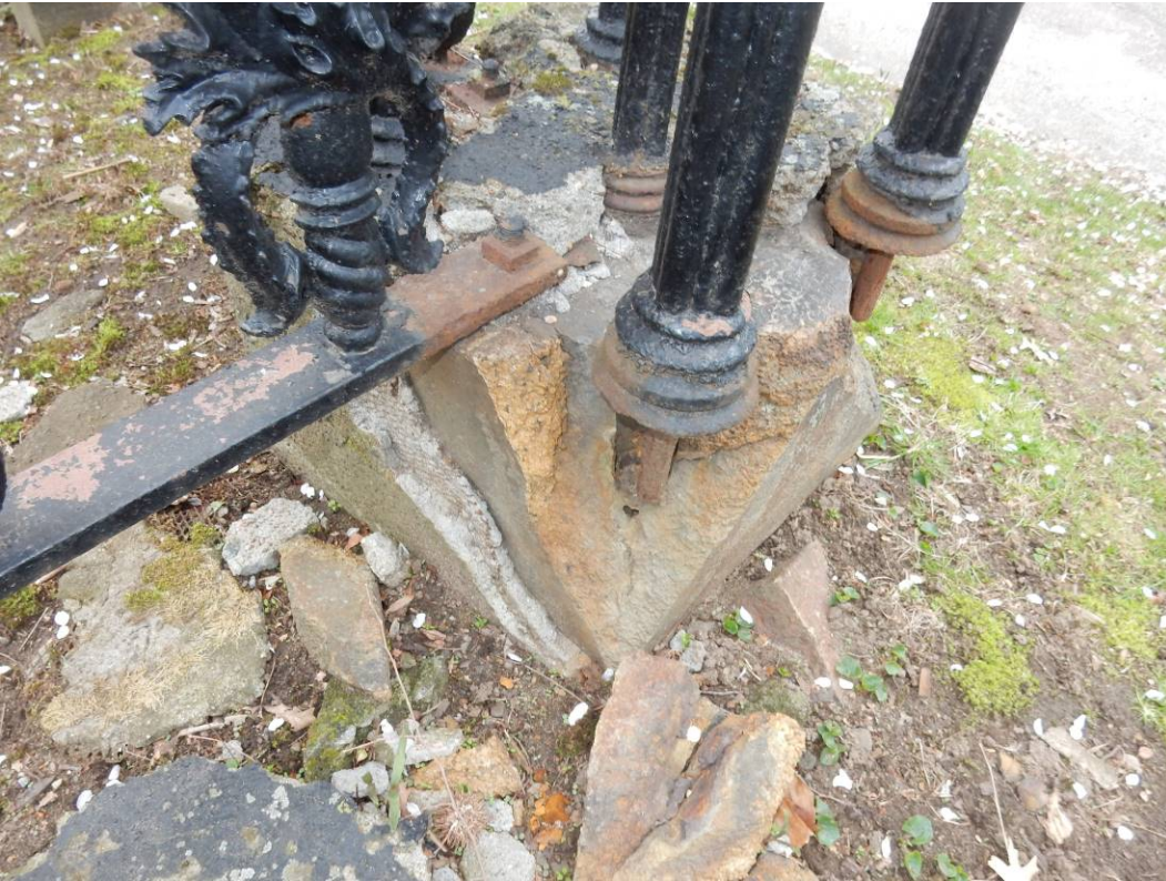
Photo 16 (Example of damaged concrete base, labeled “A” on Site Plan)
