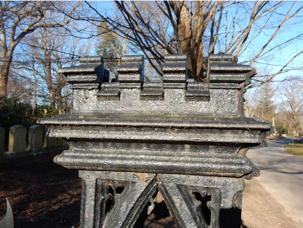
Photo 52 (Post C, example of separated cast iron elements and elements out of alignment)
