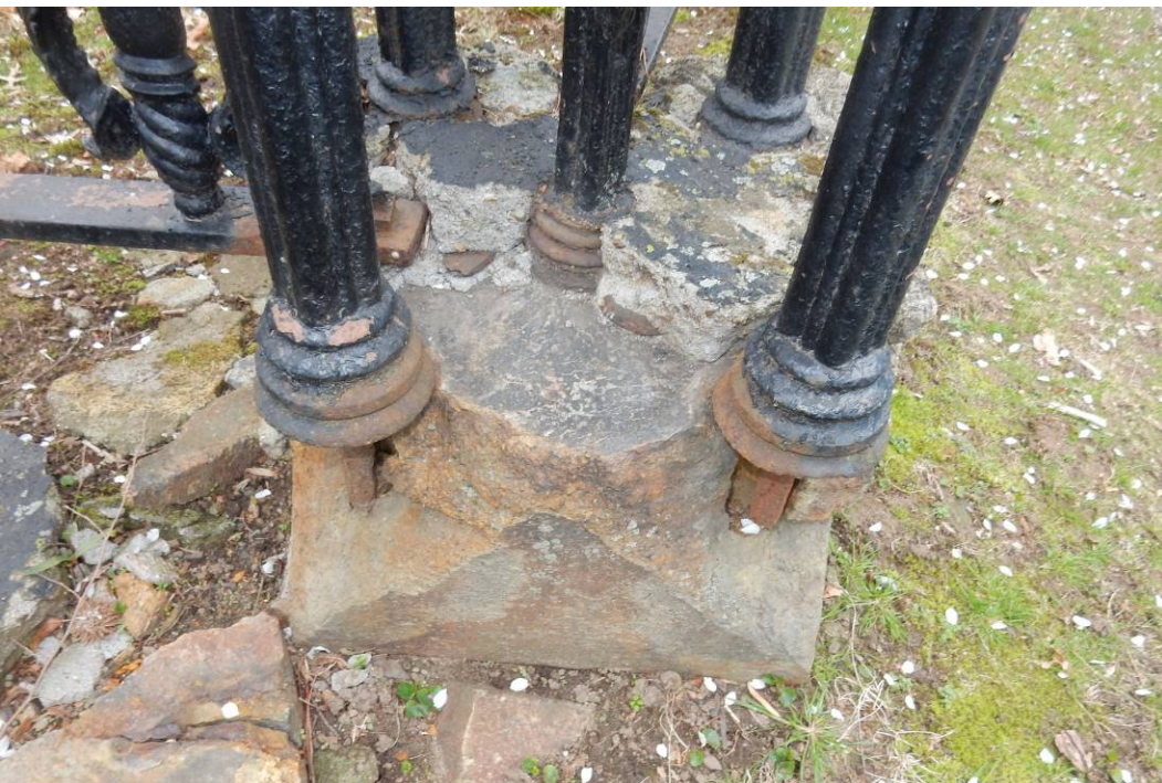
Photo 16 (Example of damaged concrete base, labeled “A” on Site Plan)
