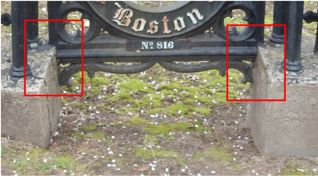
Photo 38 (Lower gate elements embedded / hidden in retrofit concrete cap)
