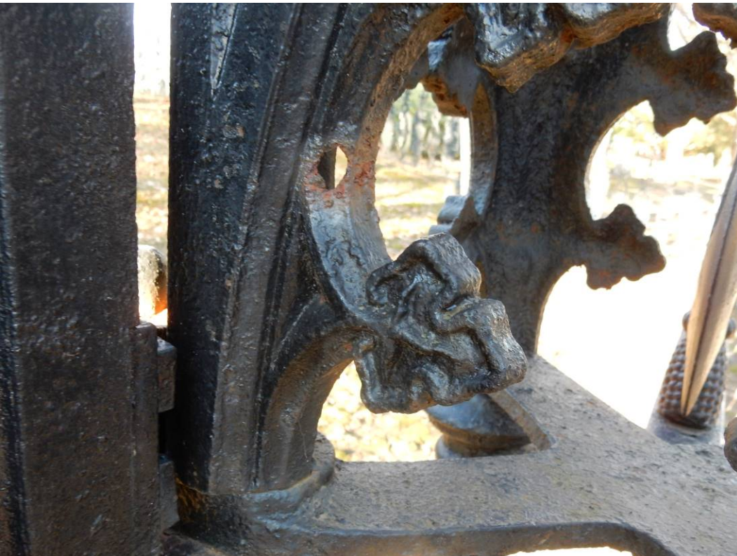
Photo 34 (Example of rust damage)
