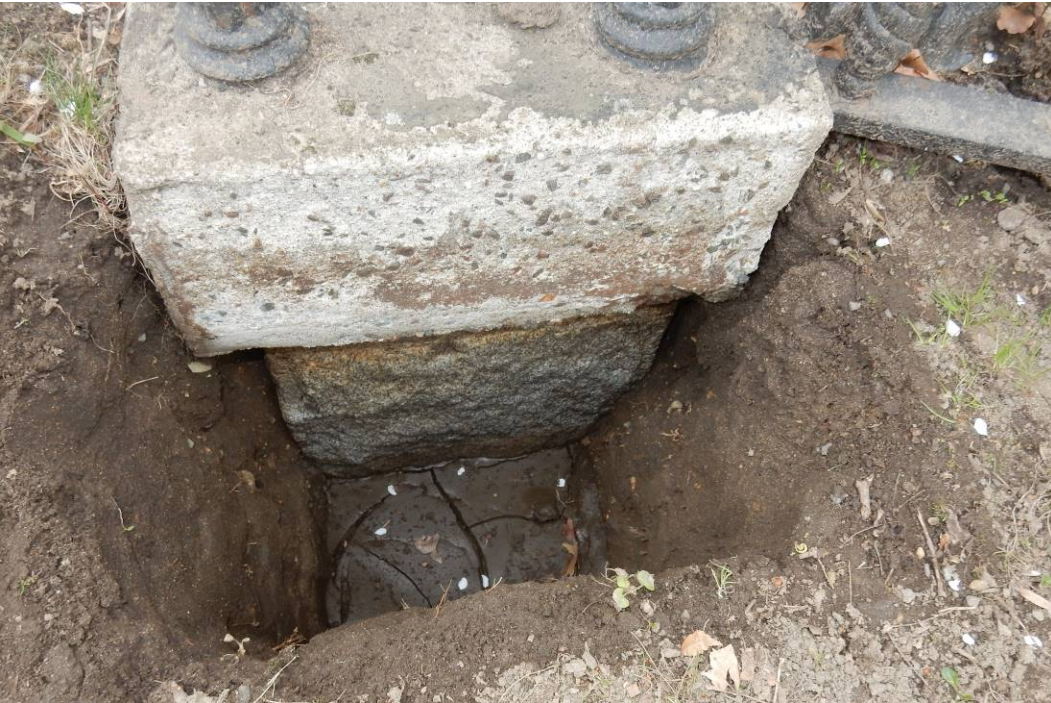
Photo 11 (Example of exposed granite base post at corner, location “F” on Site Plan)
