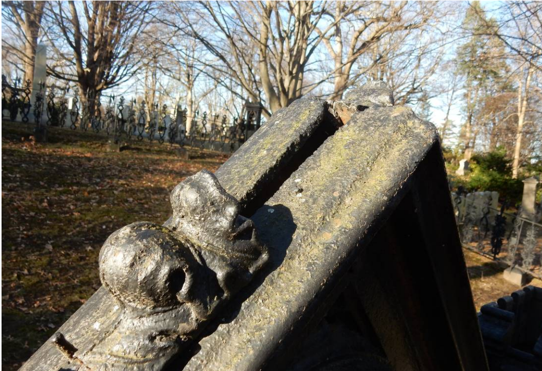
Photo 32 (Example of separated cast iron elements)
