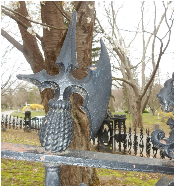
Photo 26 (Example of top decorative cast iron element out of plumb, #F13 on East Elevation)
