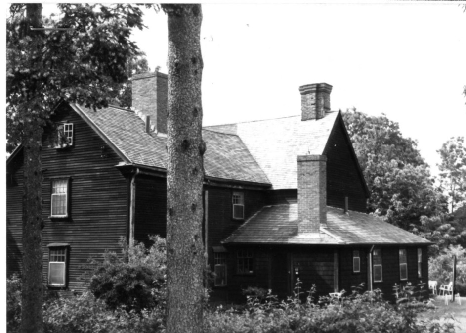
18 th c. addition. 1985.
