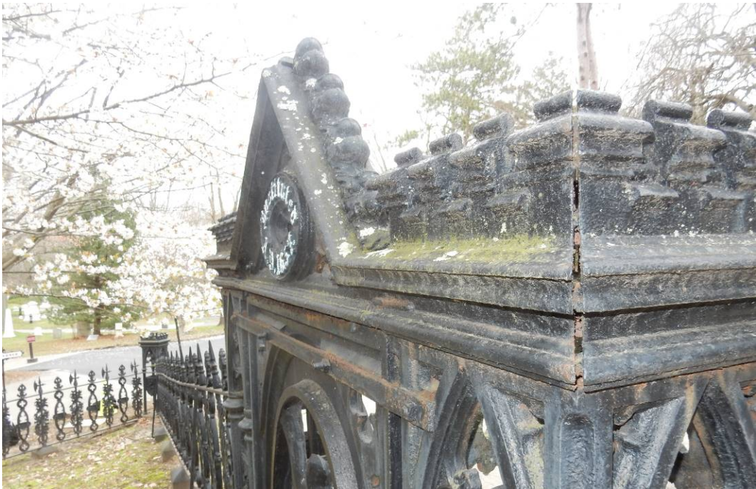
Photo 37 (Example of separated cast iron elements and biological growth)
