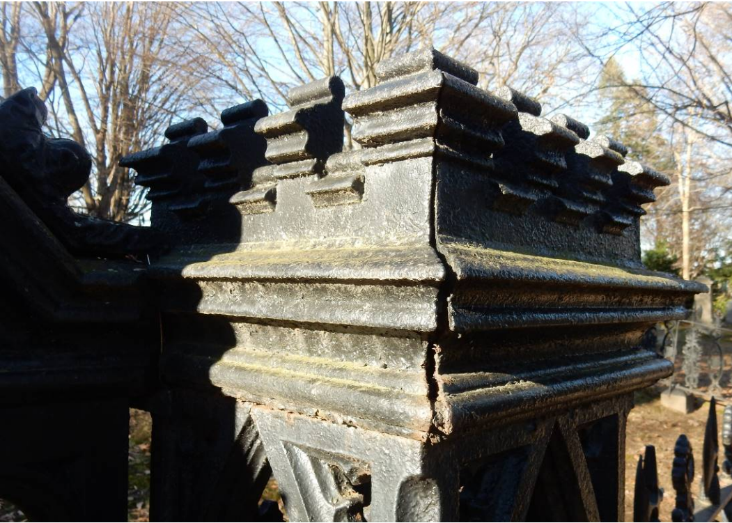
Photo 34 (Example of rust damage)
