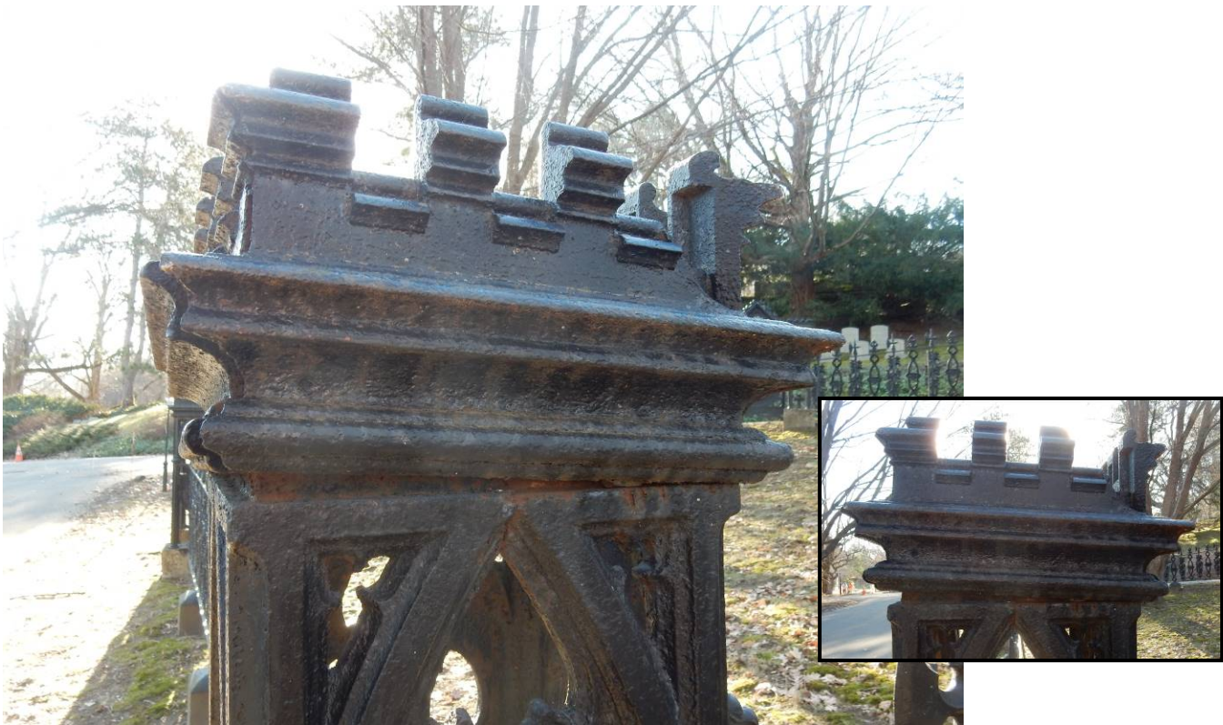
Photo 54 (Post C, example of missing cast iron element: crenellation)
