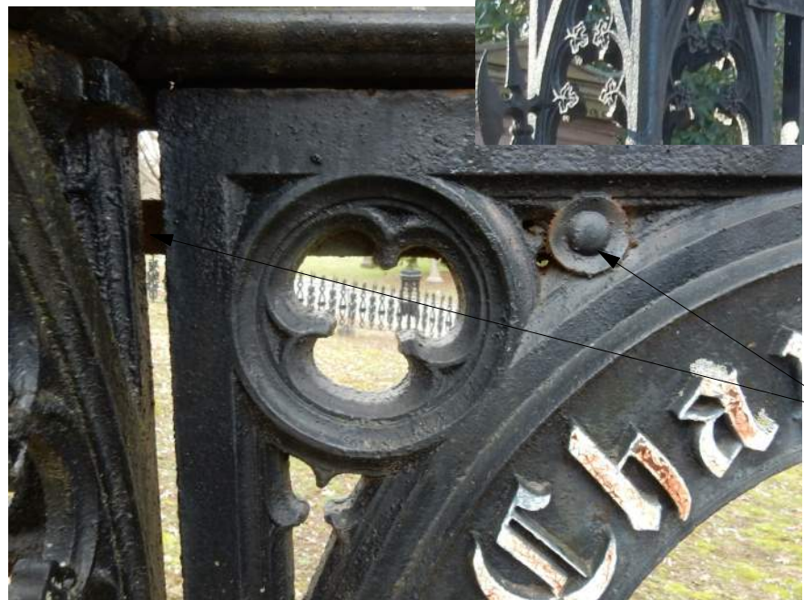
NOTE: GATE 1 IS NOT OPERABLE. NO EVIDENCE OF HINGES OR LOCK MECHANISM. GATE IS SECURED FROM THE BACK WITH A CAST IRON BAR ANCHORED WITH BOLTS AND WASHERS.
