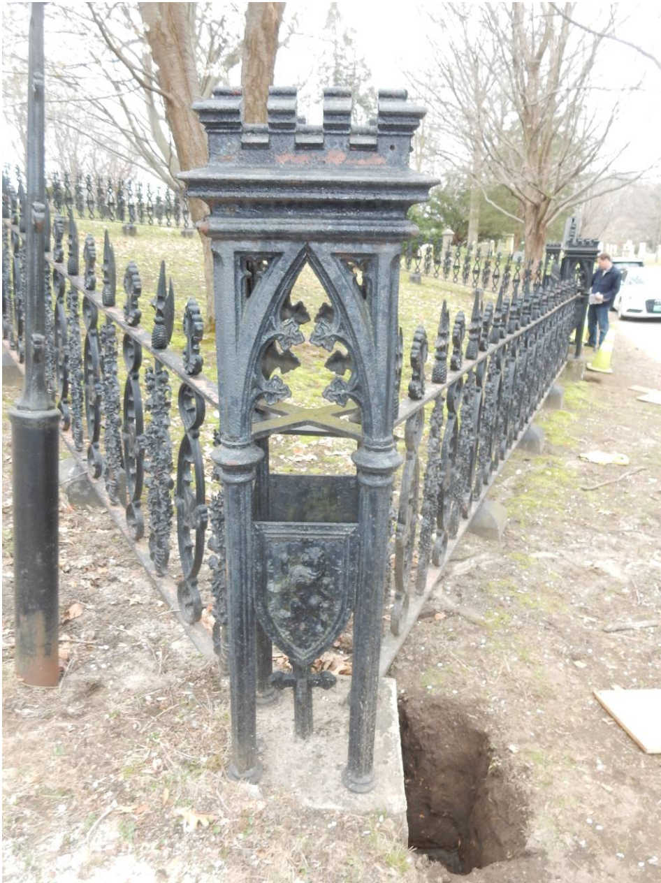
Photo 07 (Corner post, Northeast, labeled “F” on Site Plan)
