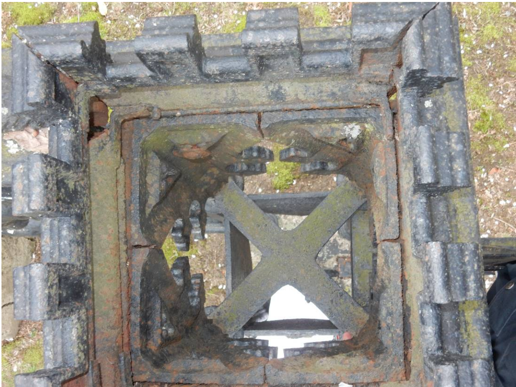
Photo 42 (Example of rust and rust damage)
