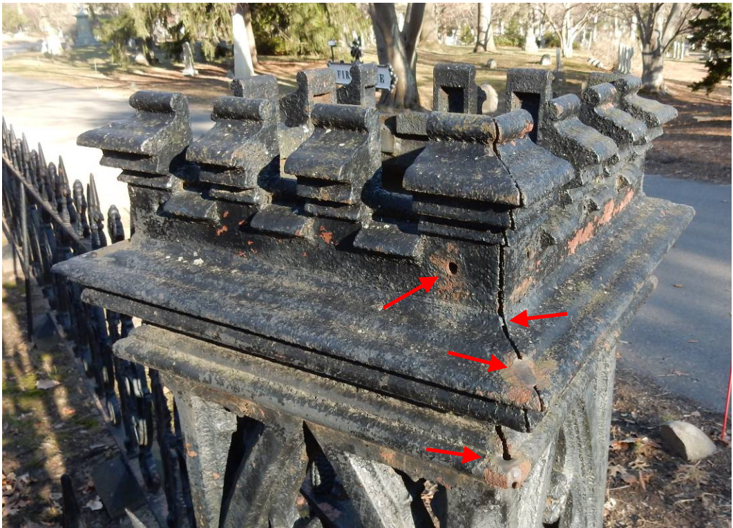
Photo 56 (Post F, example of separated cast iron elements, biological growth, missing cast iron plugs, and missing cast iron element: crenellation)
