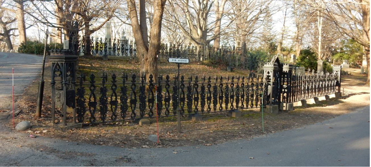
Photo 01 (Overall view, North Elevation along Fir Avenue)
