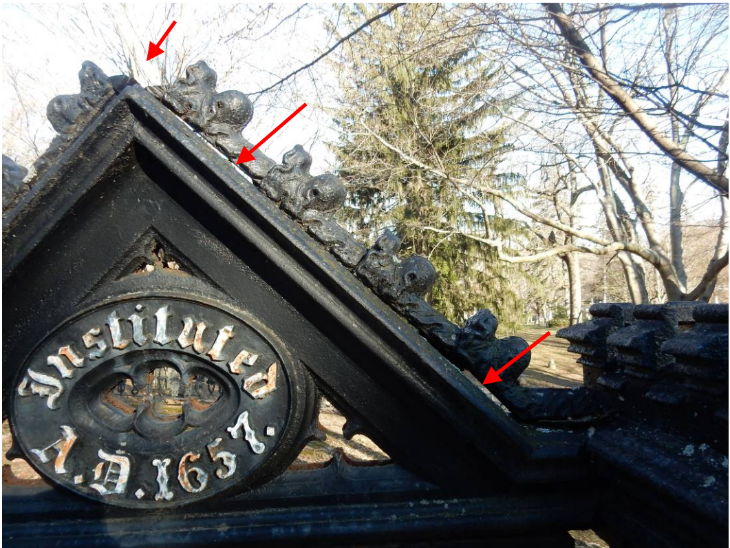
Photo 36 (Example of separated cast iron elements)
