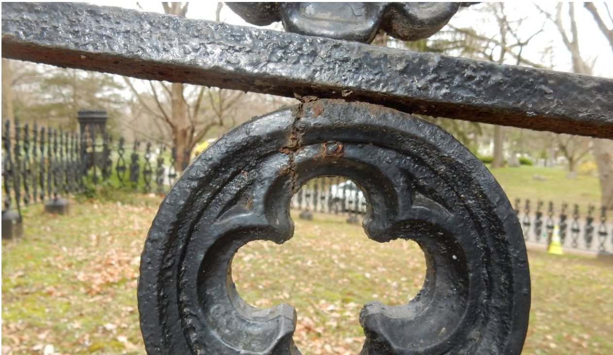
Photo 26 (Example of top decorative cast iron element out of plumb, #F13 on East Elevation)
