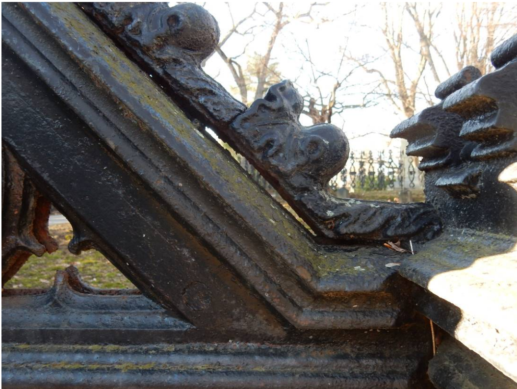
Photo 32 (Example of separated cast iron elements)
