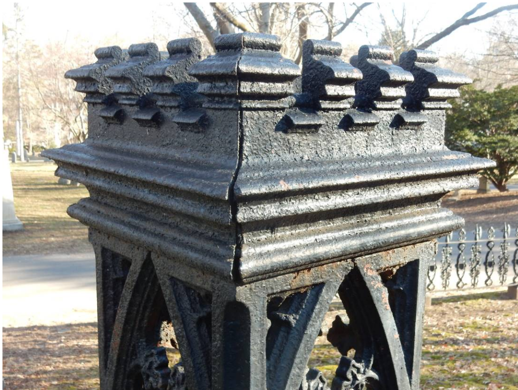
Photo 48 (Post B, example of separated elements)
