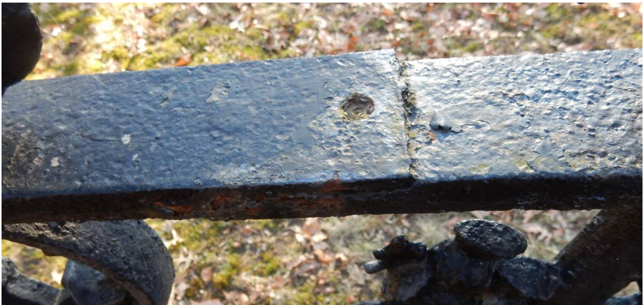
Photo 20 (Example of top rail splice)
