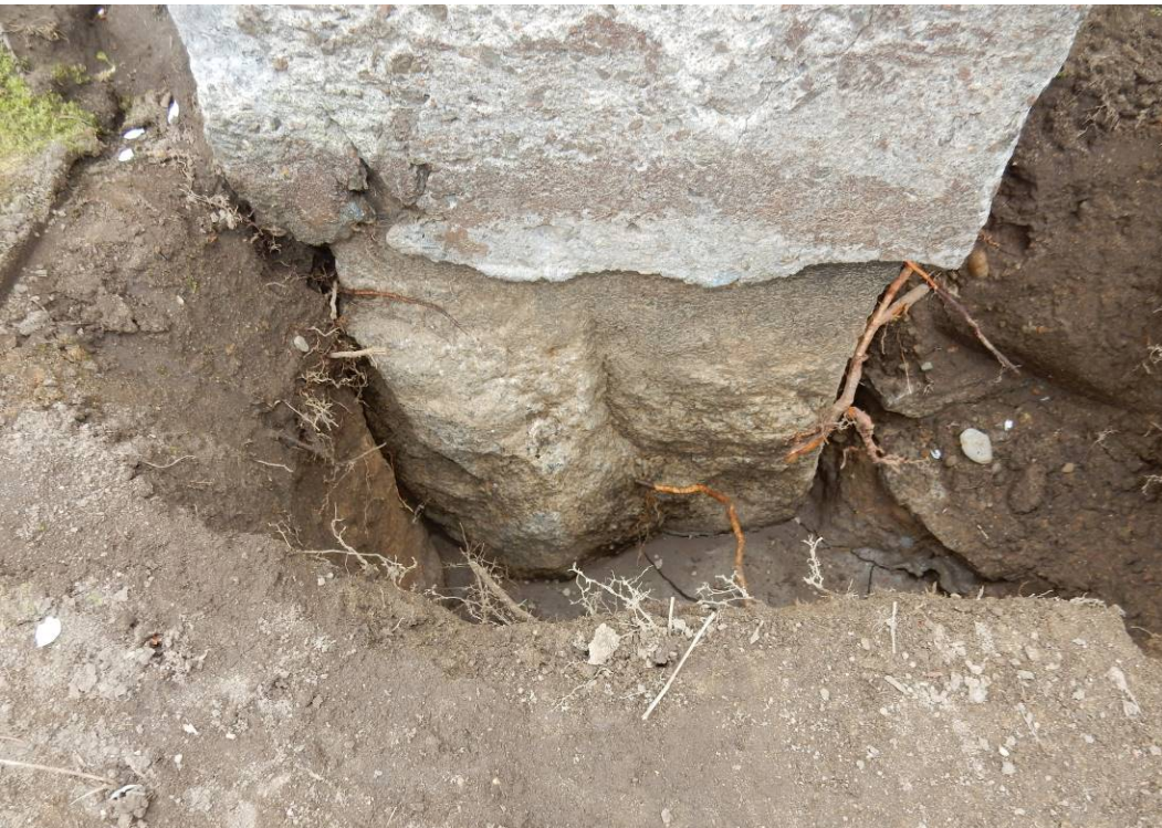
Photo 12 (Example of exposed granite base post at entrance gate, location “E” on Site Plan)
