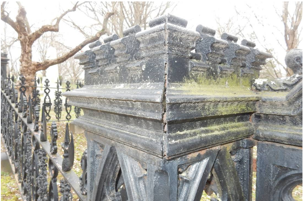
Photo 36 (Example of separated cast iron elements)
