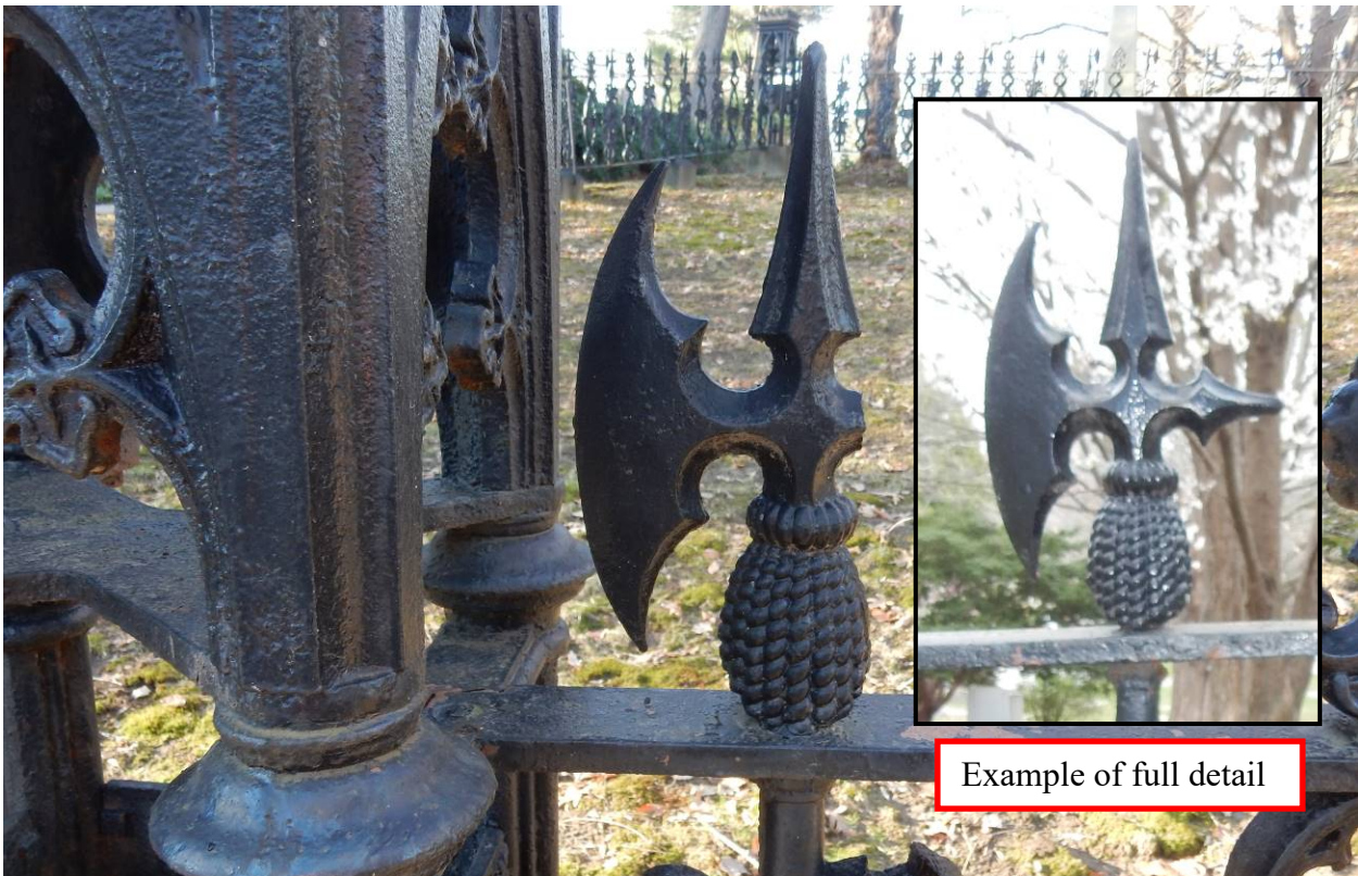
Photo 24 (Example of missing cast iron detail, #C28 on North Elevation)
