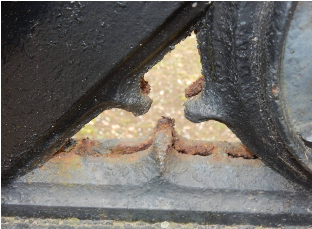
Photo 40 (Example of rust damage)
