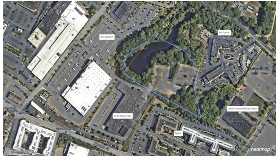
Figure 3: Aerial of Walker Pond and surrounding properties, 2023 (source: Nearmap GIS)
