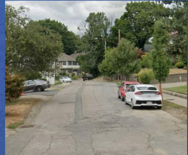
East Bates Road - Before
