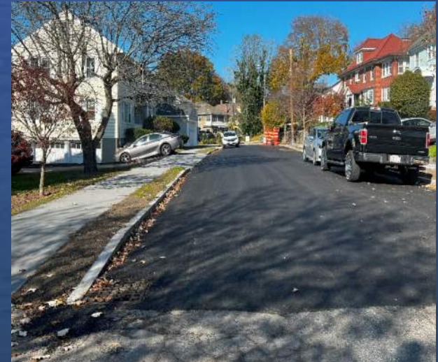
East Bates Road - After
