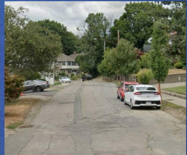
East Bates Road - Before
