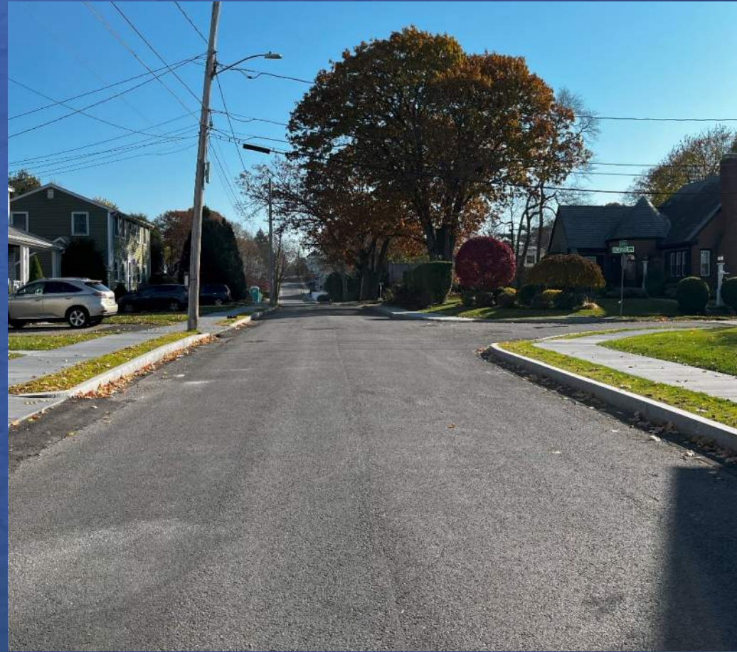
Highland Ave - After
