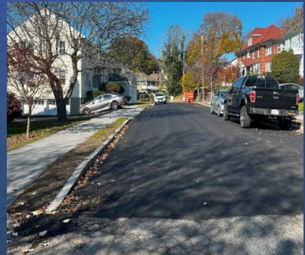
East Bates Road - After
