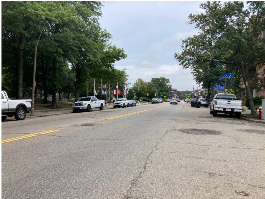
View of MH1096 and Main Street facing southeast.
