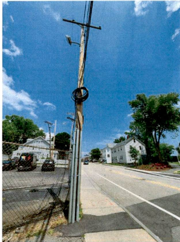
View of utility pole #225/5 on Howard Street facing the intersection between Howard Street and Acton Street.
