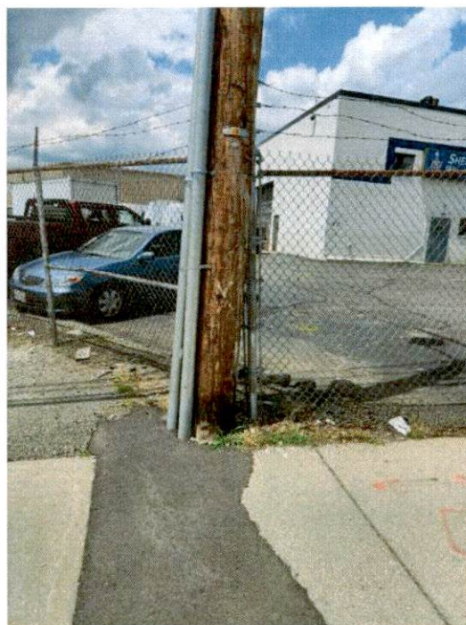
View of utility pole #225/5 on Howard Street opposite of municipal parking lot.
