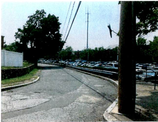
View of utility pole #6 and Winter Street facing south.
