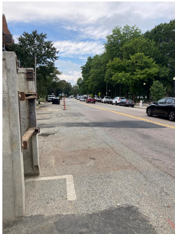
View of Main Street from service location facing northwest.
