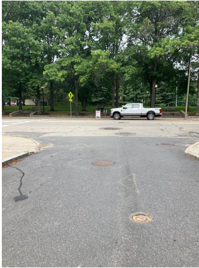
View of MH1096 at intersection of Chestnut Street and Main Street where service will be pulled from.
