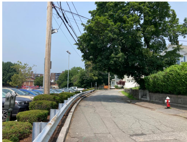
View of utility pole #5 and Winter Street facing northwest.
