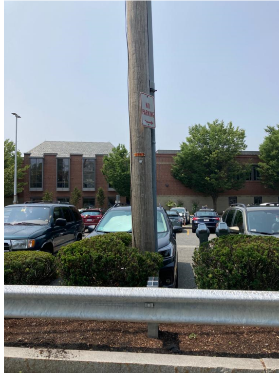
View of proposed start position of underground conduit at utility pole #5 facing southwest towards parking area.
