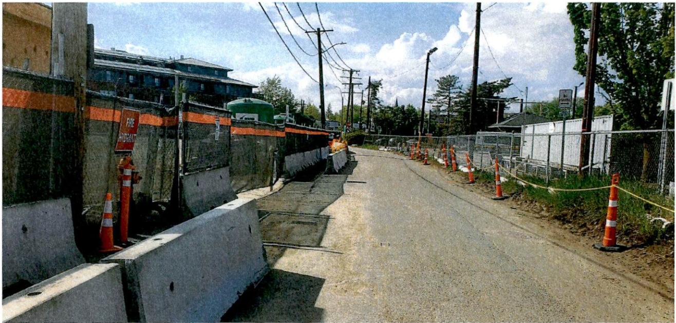
Photo 2: View of Water Street facing northwest closer to Galen Street where the connection is proposed across Water Street from 66 Galen Street.
