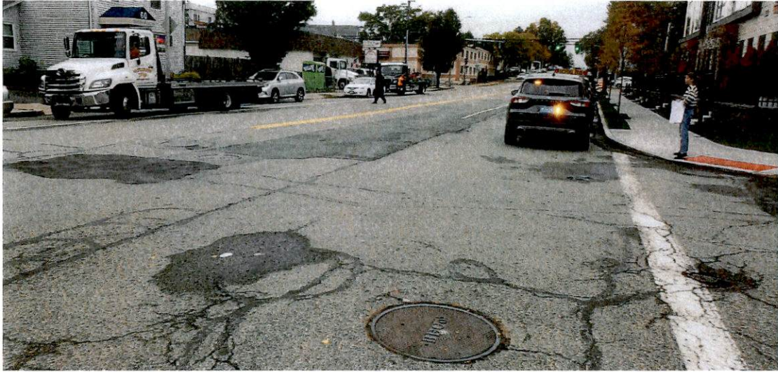
Photo 6: View of North Beacon Street facing East at Manhole #9902
