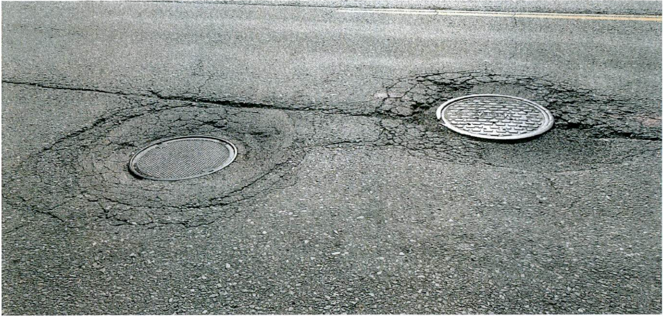
Photo 4: View of manhole MH 16/205.
