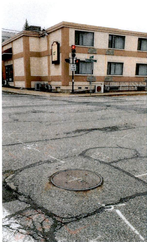
Photo 7: View of North Beacon Street and Irving Street Intersection at location of Manhole #9904
