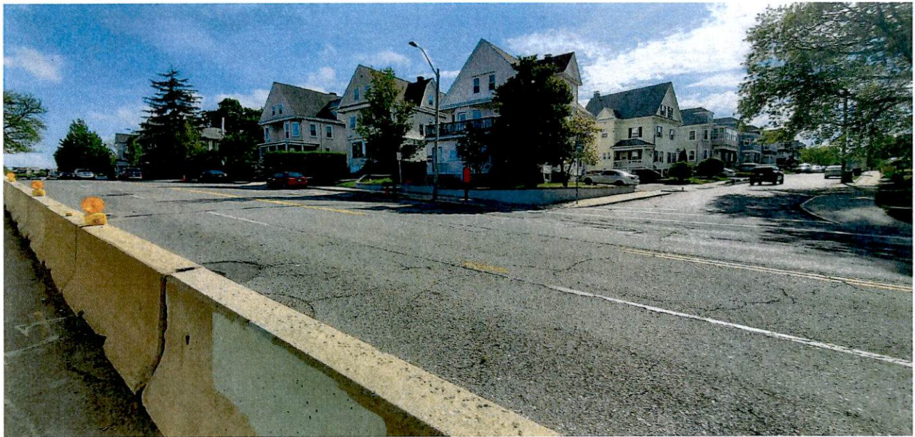
Photo 5: View of Galen Street facing South where the connection is proposed from manhole MH 16/205A to the 66 Galen Street Property.
