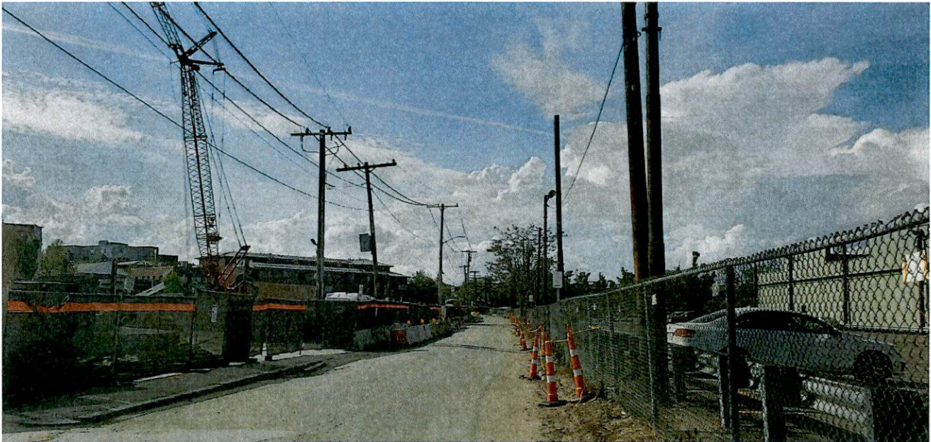
Photo 1: View of Water Street facing northwest where the connection is proposed across Water Street from 66 Galen Street.
