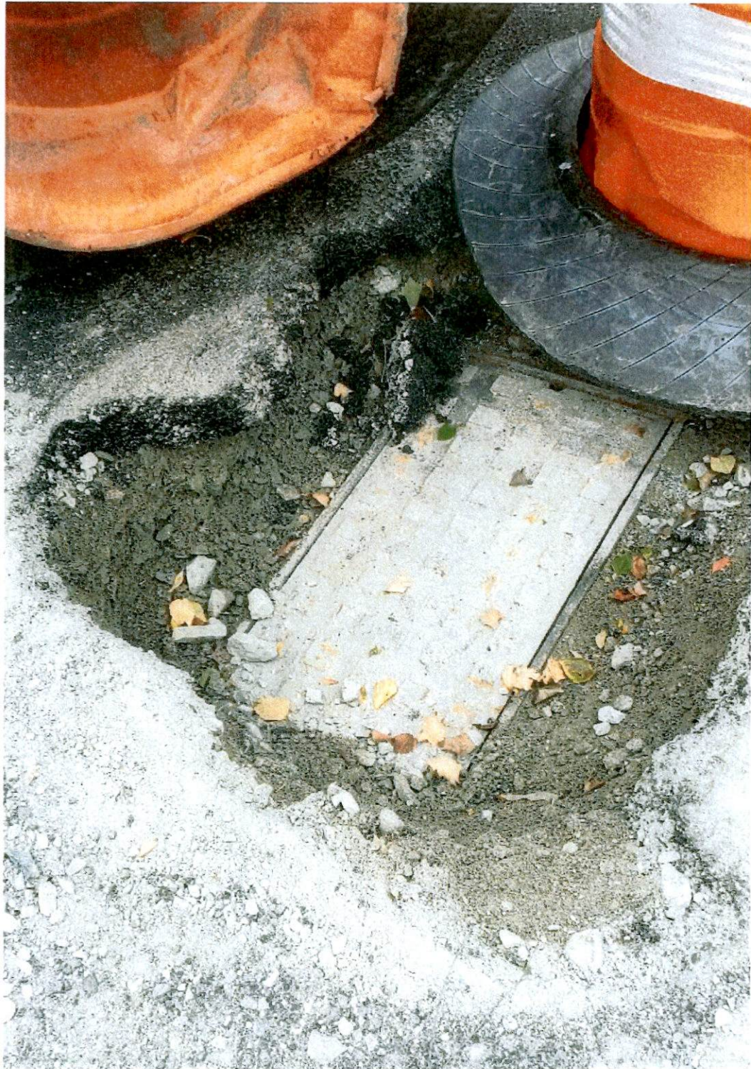
Photo 1: View of pull box on Arsenal Street where the service connection is proposed.
