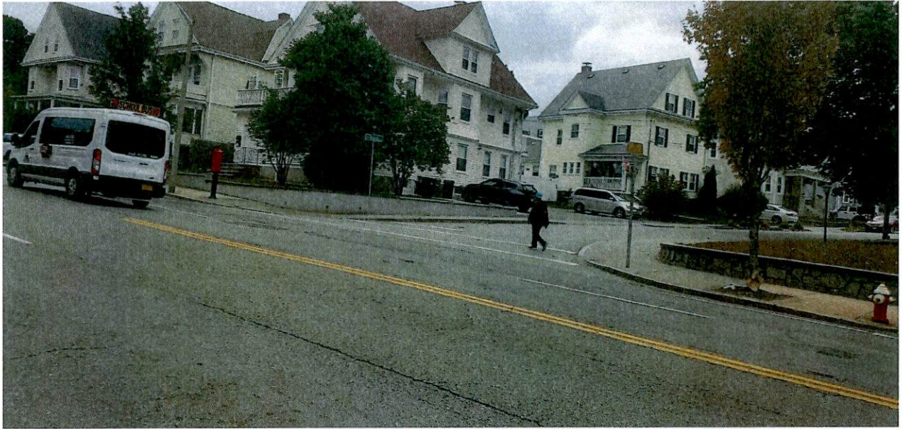
Photo 3: View of connection point on Union Street facing West
