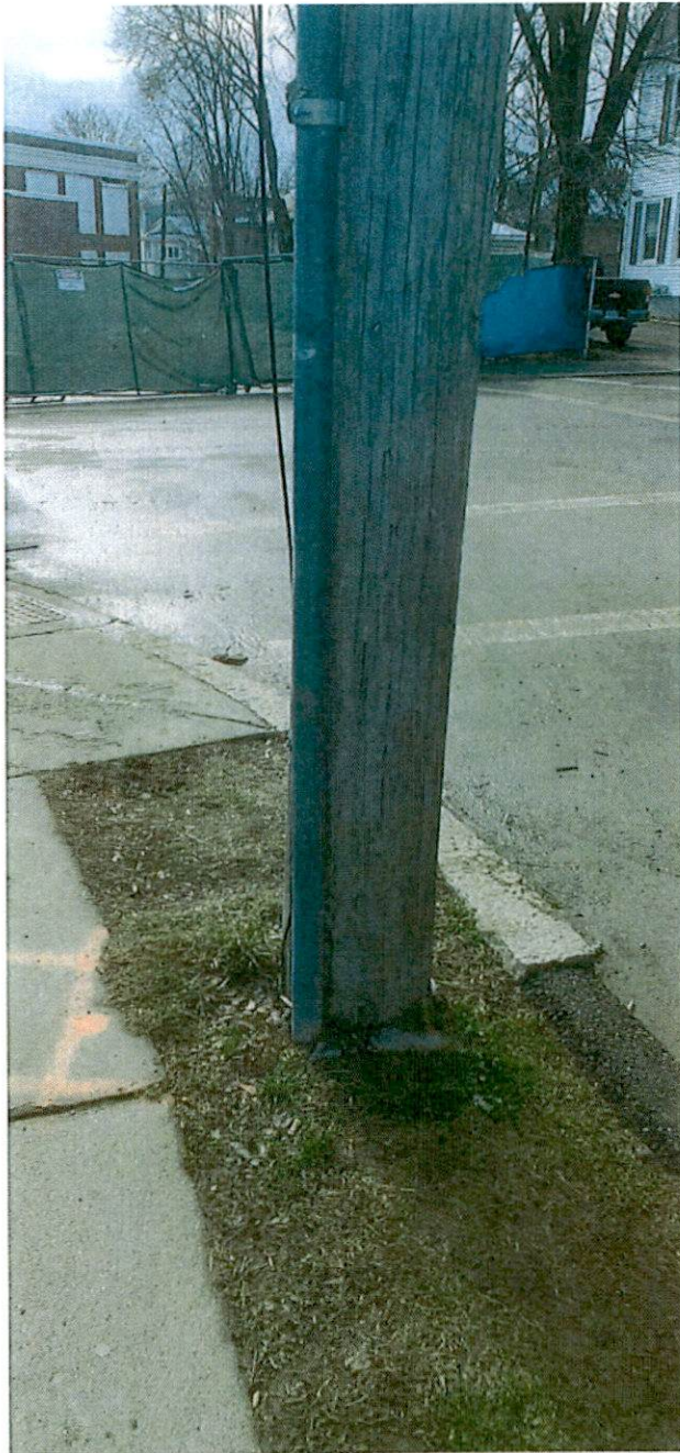
View of Utility Pole 193/10 and associated riser depicting the existing electrical run east and proposed work zone.
