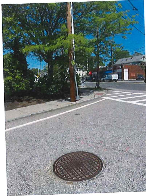
View of MH10703 and utility pole #225/0 on Howard Street facing Main Street.
