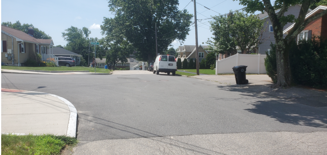
View of Nyack Street and Tappan Avenue facing southwest at the location where the new gas main will be installed to extend the existing main towards Madison Avenue.
