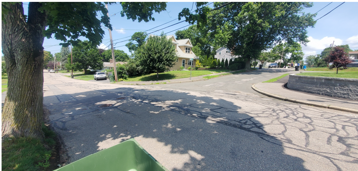
View of the end connection of the new gas main at the intersection of Nyack Street and Madison Avenue.
