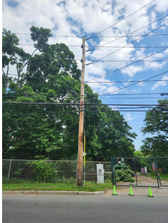
View of Mount Auburn Cemetery and utility pole #63/16 on Grove Street.
