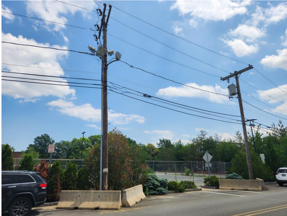
View of utility pole #16/68-2 and utility pole #16/68-2A 2A on Pleasant Street opposite of Paramount Place.
