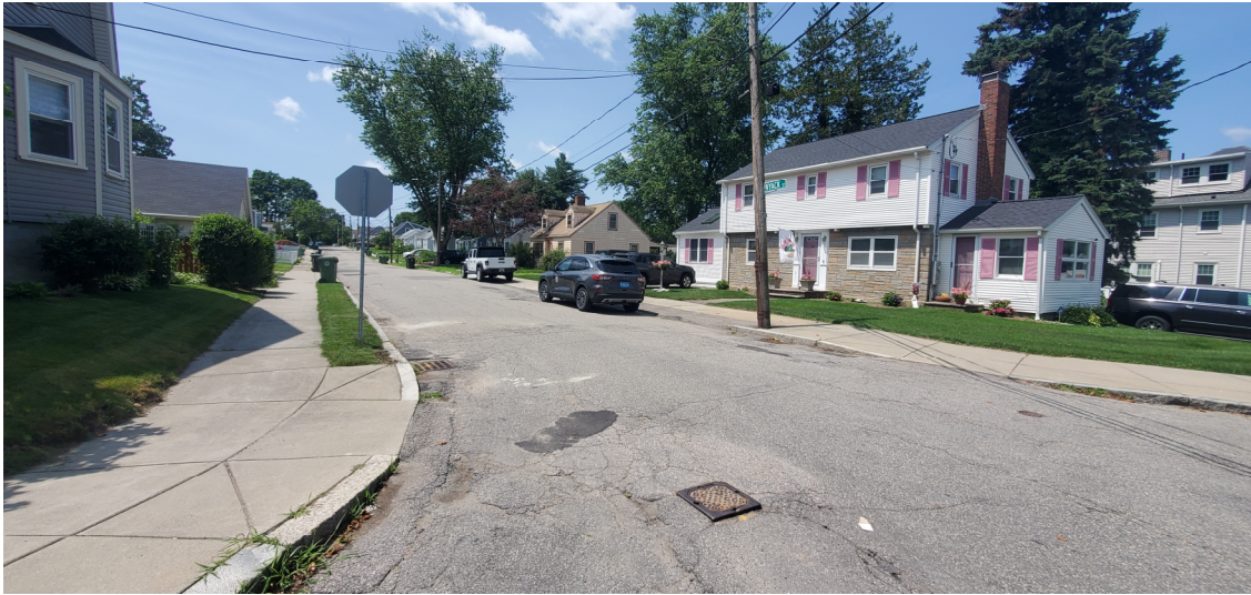
View of Nyack Street and Belmont Street where existing gas man is to be replaced facing southwest.
