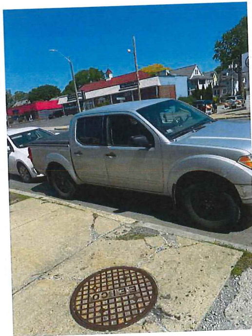
View of MH11286 facing towards Westminster Avenue.
