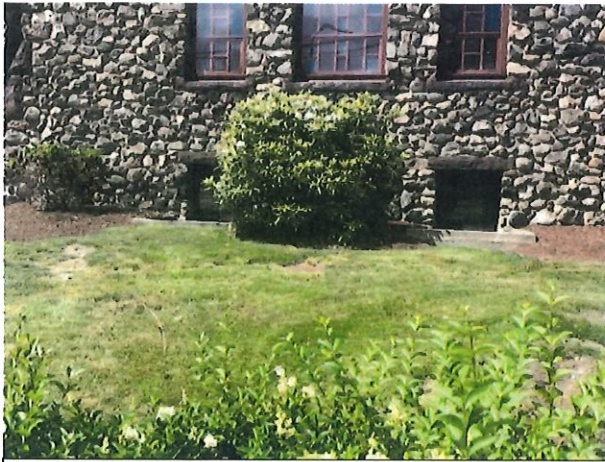
View of two basement windows on south side from Mt. Auburn St. sidewalk.
