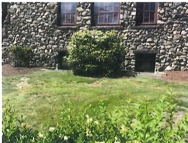
View of two basement windows on south side from Mt. Auburn St. sidewalk.
