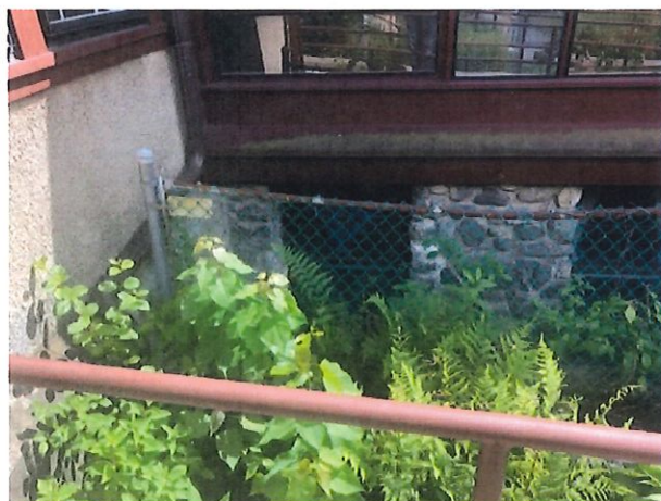
View of one window on north side, from ramp to parish house entrance.
