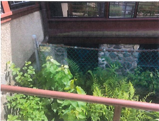
View of one window on north side, from ramp to parish house entrance.
