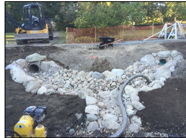
Figure B-4. Stormwater improvement following stone placement (October 2015).
