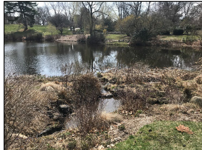
Figure B-12. Improvement as seen during maintenance visit March 2021.
