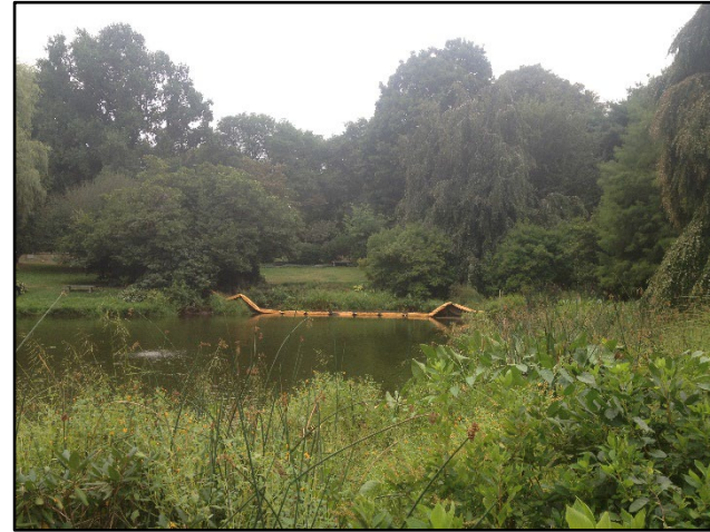
Figure B-2. Installation of floating silt fence (September 2015).
