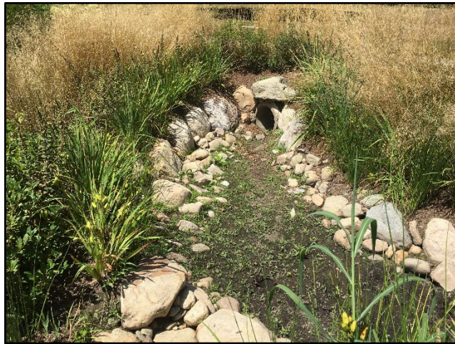
Figure B-11. Sediment accumulation in improvement fall 2016.
