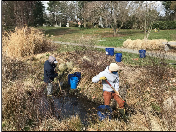
Figure B-13. Sediment removal in stormwater improvement area (March 2021).
