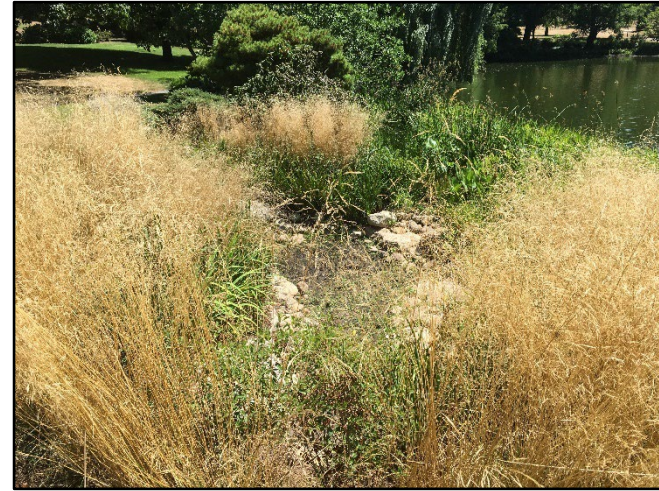
Figure B-10. Accumulated sediment in improvement prior to maintenance 2016.
