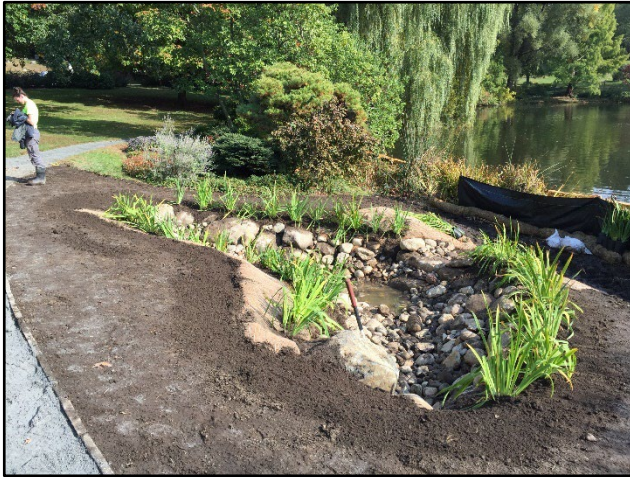
Figure B-5. Installation of plantings (October 2015).
