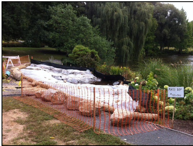
Figure B-3. Construction of the stormwater improvement (October 2015).
