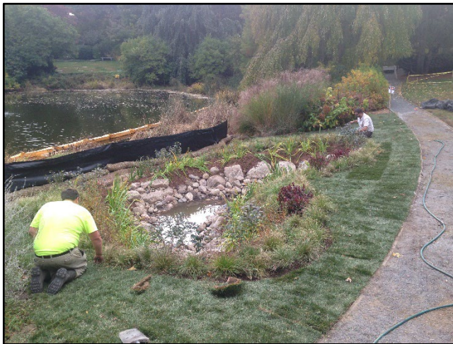
Figure B-7. Final planting and sod placement. (Oct. 2015)
