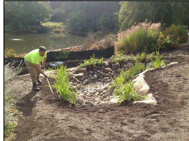
Figure B-6. Preparation of sod bed prior to installation (October 2015).
