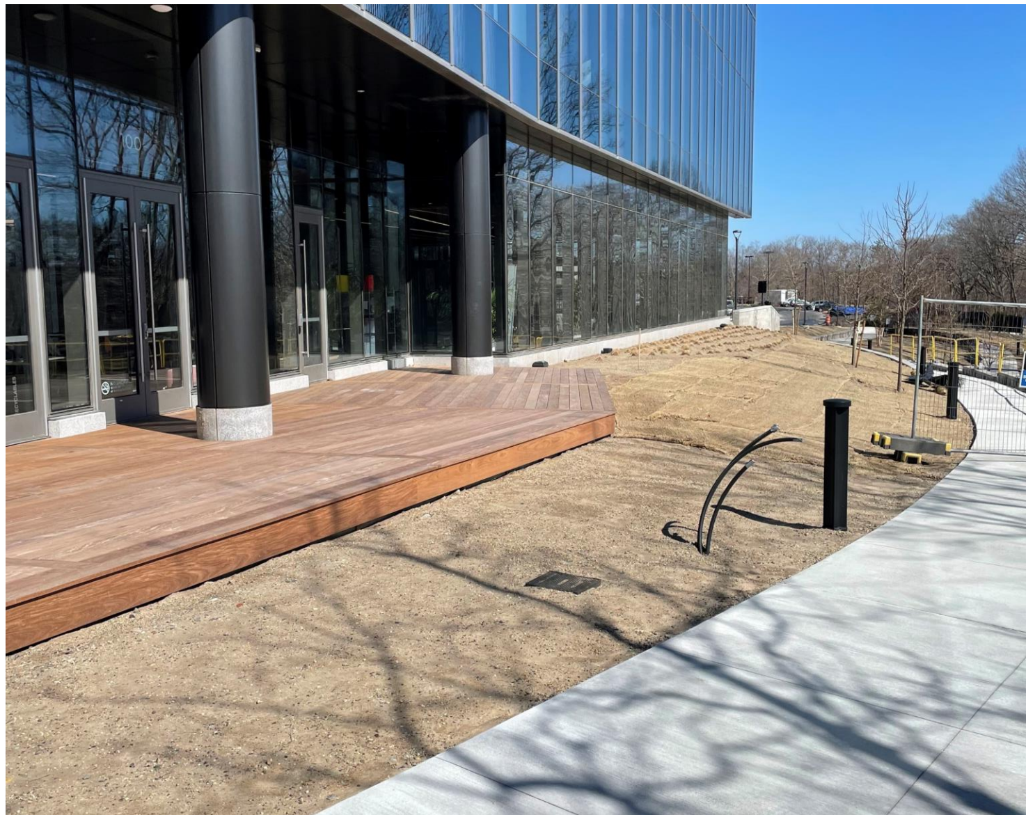
Exterior deck at 100 Forge
