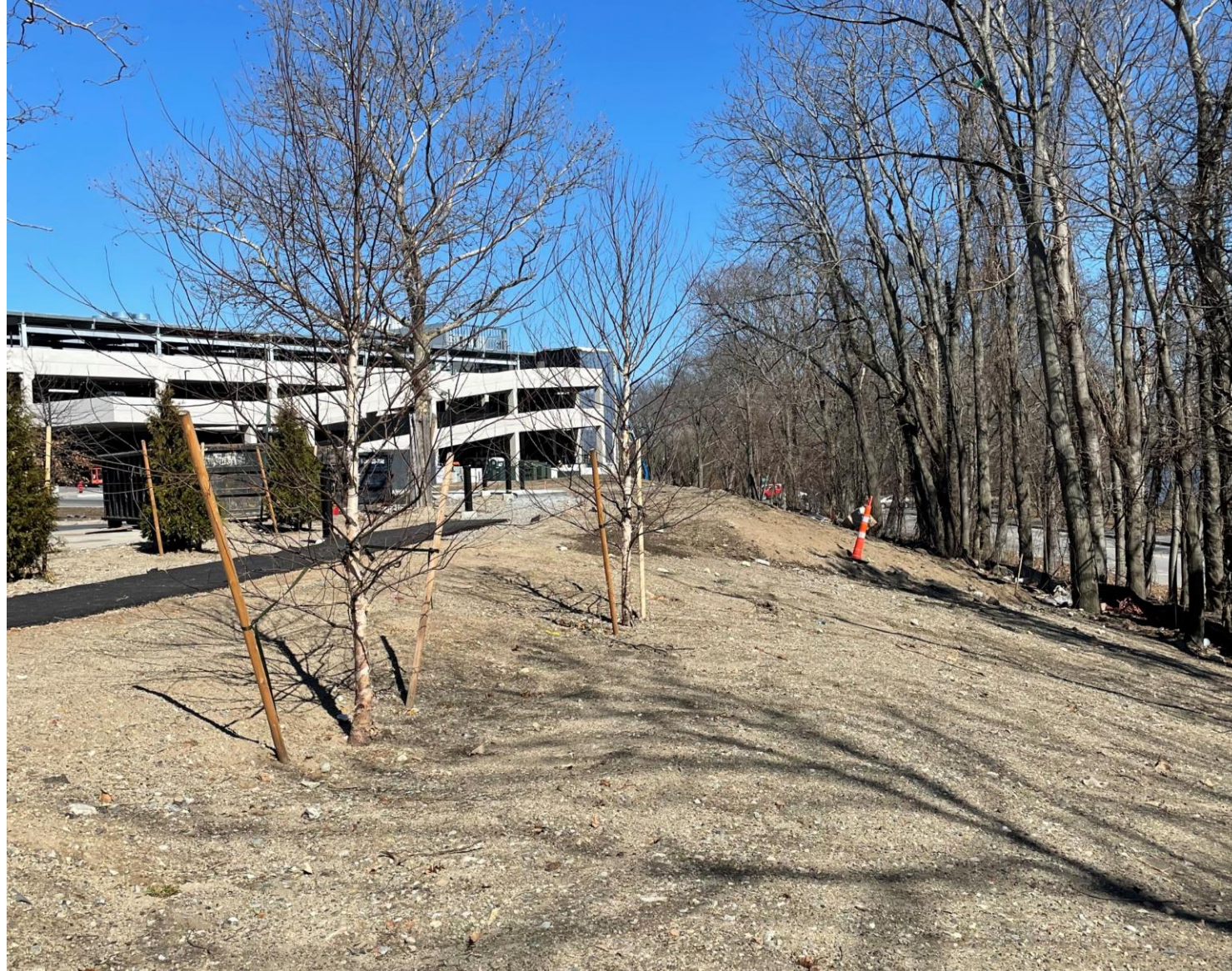
Landscape progress photo facing 500 Forge
