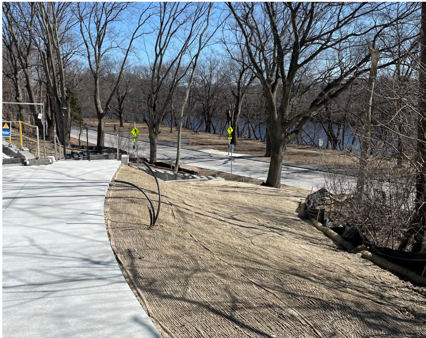
Pedestrian path to Greenough Boulevard
