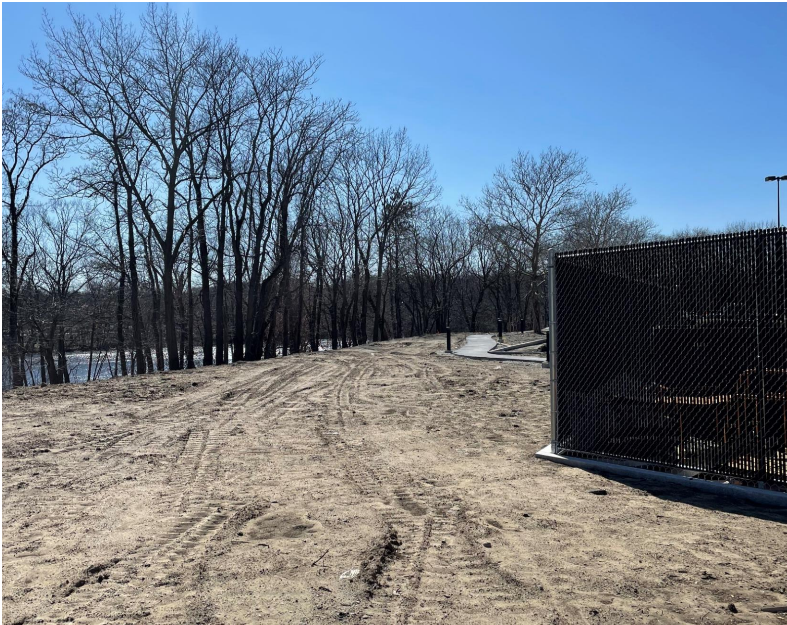
Rear of new Home Depot dumpster enclosure
