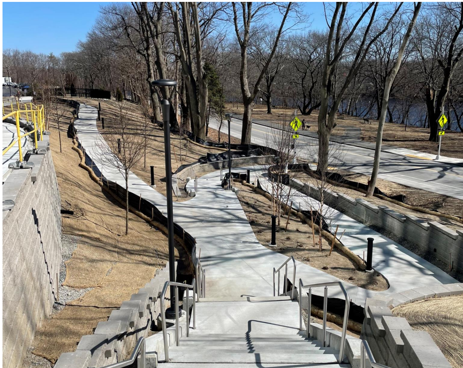
Stairway to Greenough Blvd.
