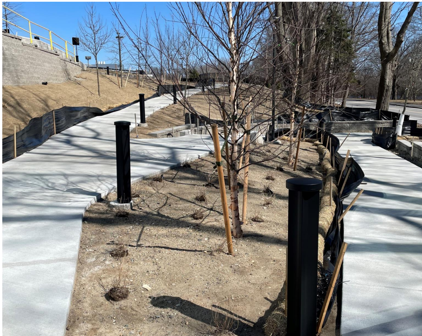
Switchback Ramp to Greenough Blvd.
