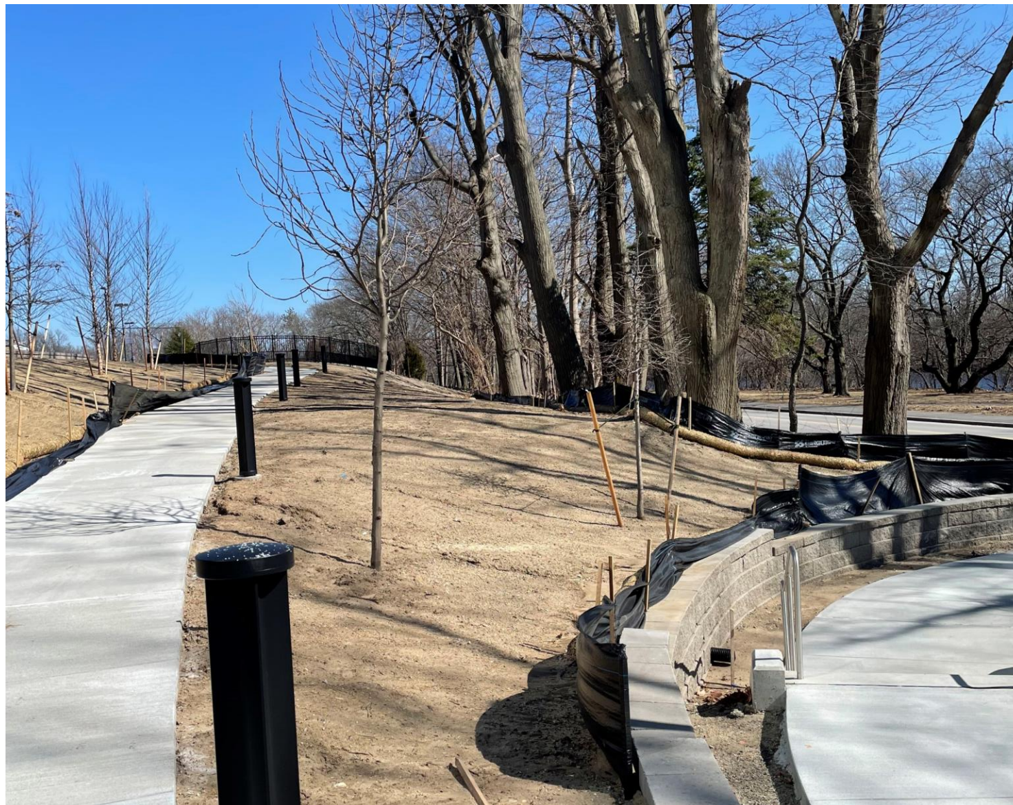
Retaining wall at Switchback Ramp
