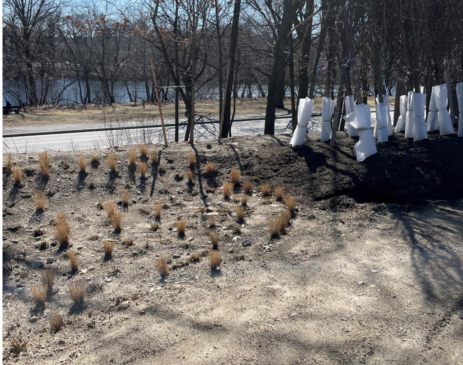
Landscape planting progress photo
