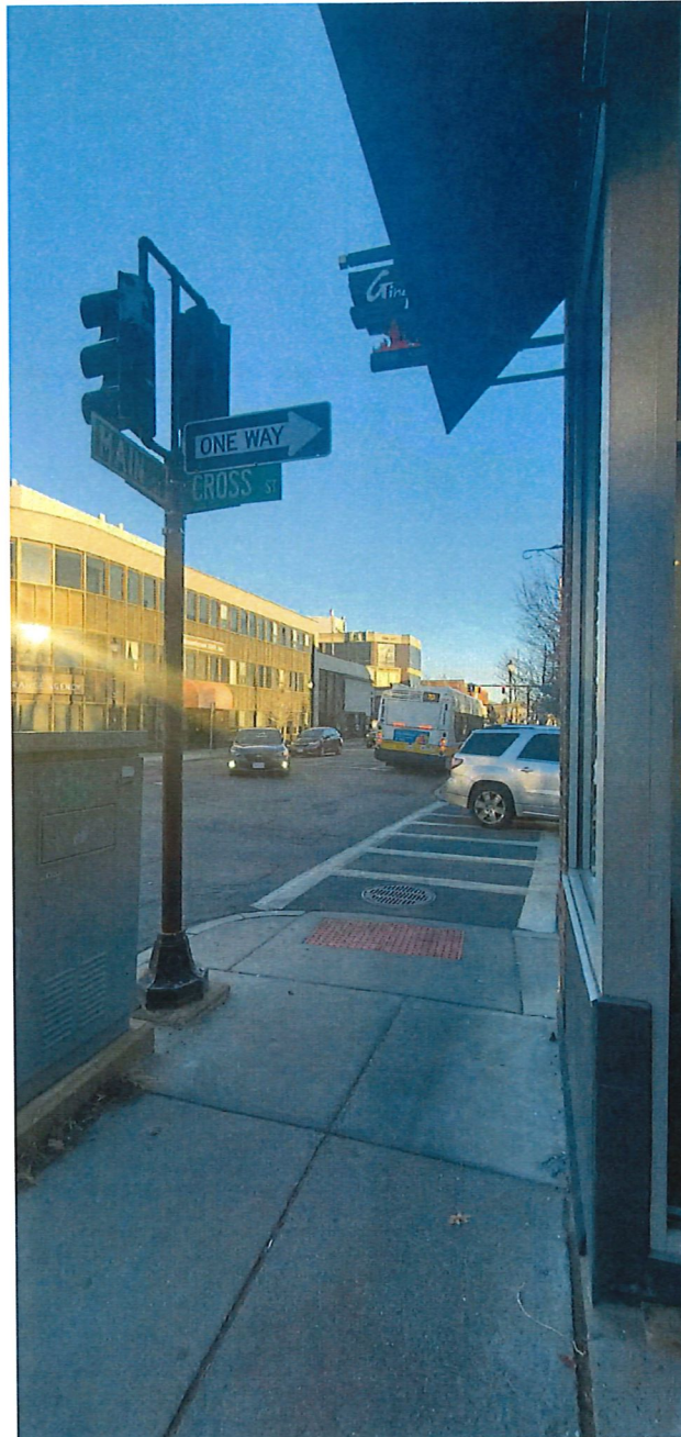
View of Existing Manhole and ADA Curb Ramp Where Service will be Installed from.
