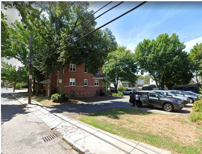
5. FROM MELENDY AVENUE - BUILDING 1
