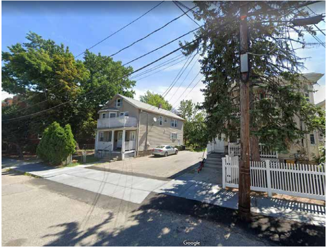
5. QUIMBY STREET - DRIVEWAY
