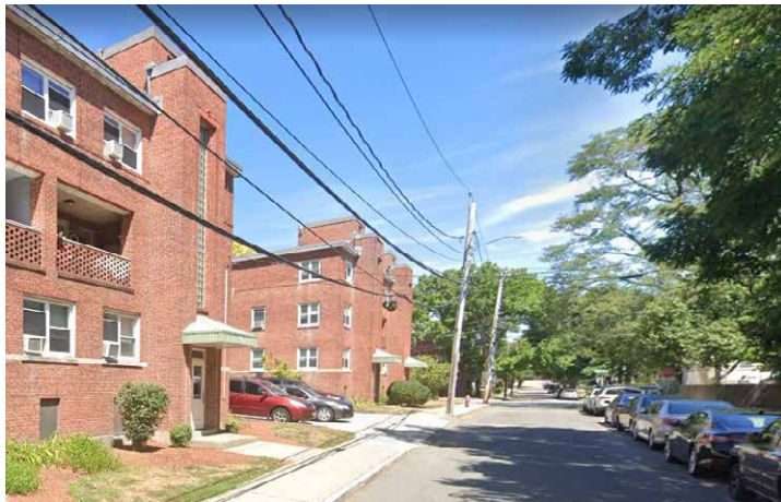
3. FROM MELENDY AVENUE - BUILDING 5-2
