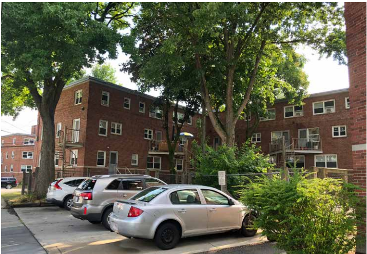
6. FROM QUIMBY STREET - BUILDING 2
