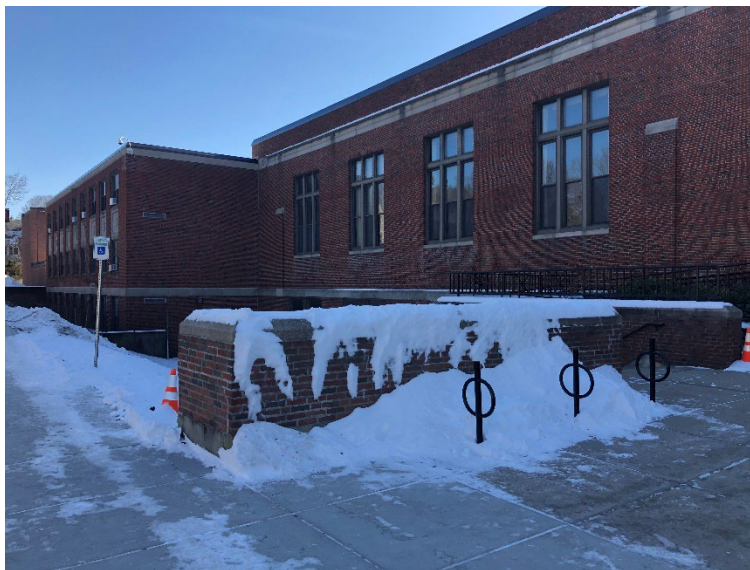
View east from Robbins Road
