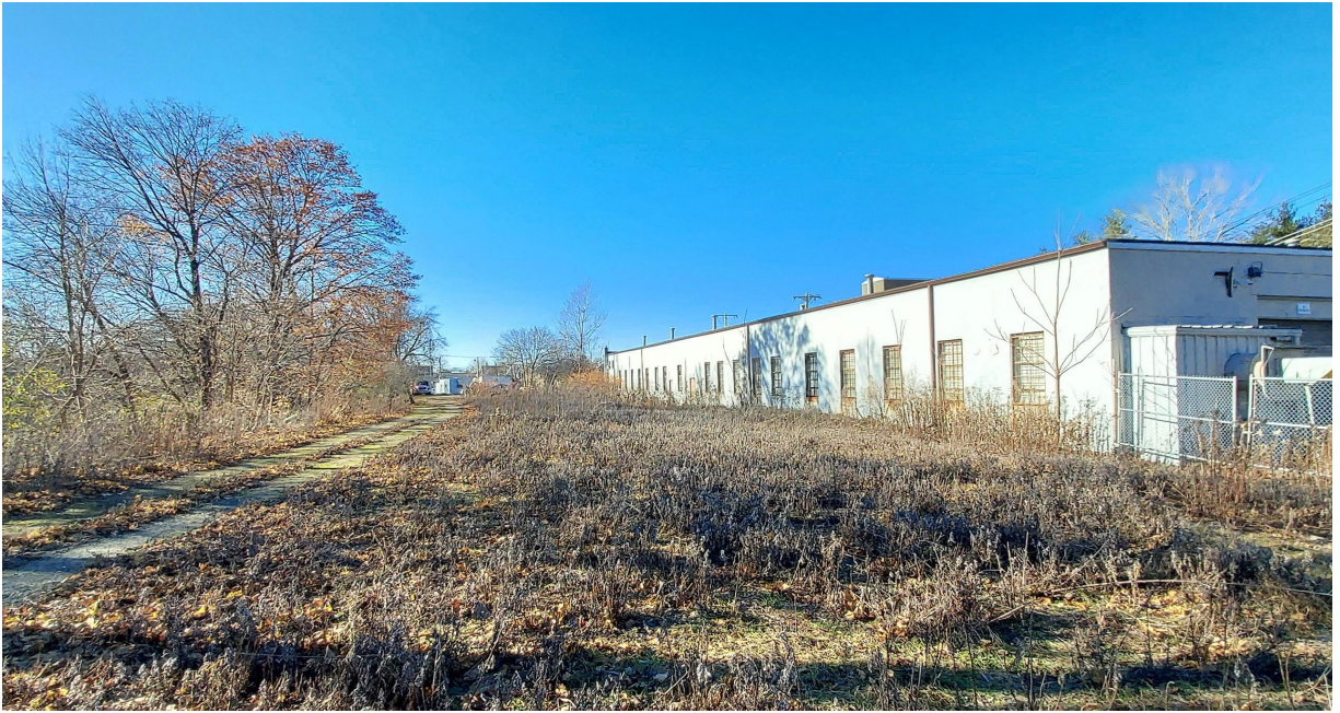
Photo #3: View the proposed Project area. Proposed work area consists of primarily herbaceous vegetation. This area is located within the 100-foot Buffer Zone and locally regulated 150-foot Buffer Zone. Sawins Pond is located south (left) of the Project area. Facing west.
