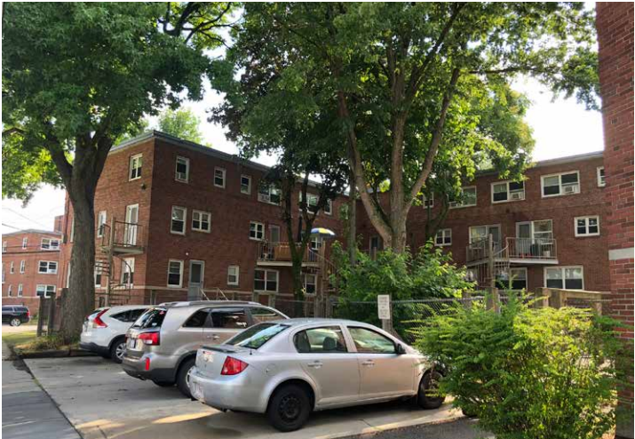
6. FROM QUIMBY STREET - BUILDING 2
