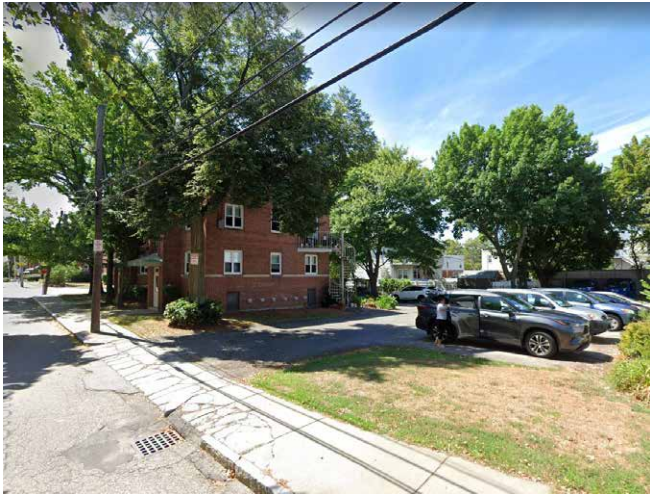
5. FROM MELENDY AVENUE - BUILDING 1
