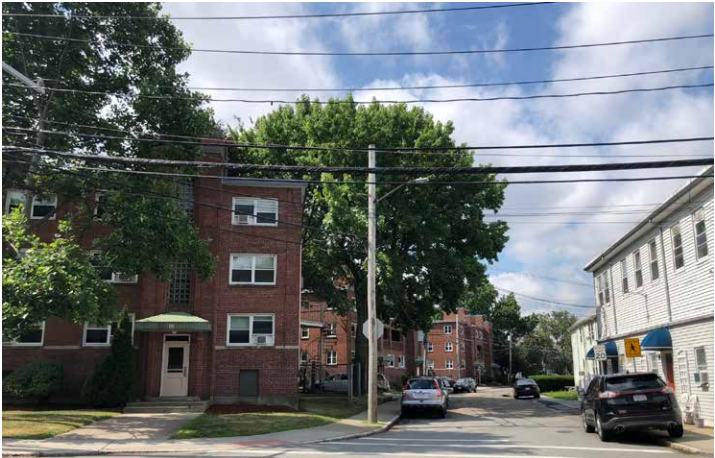
8. NICHOLS & QUIMBY STREET - BUILDING 2
