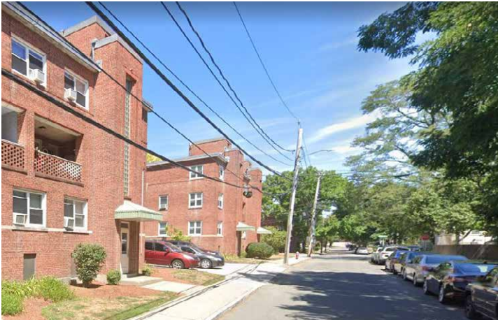
3. FROM MELENDY AVENUE - BUILDING 5-2
