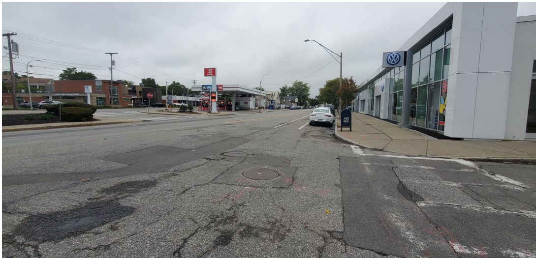
Photo 4: View of North Beacon Street facing East at Manhole #9899
