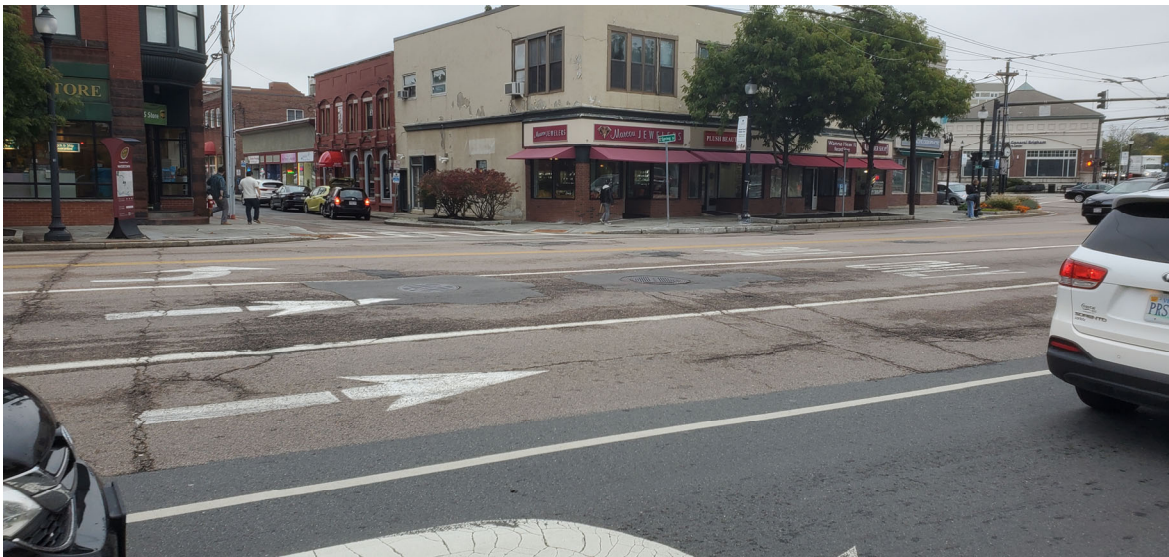
Photo 2: View of Manhole #3701 on Main Street and Spring Street
