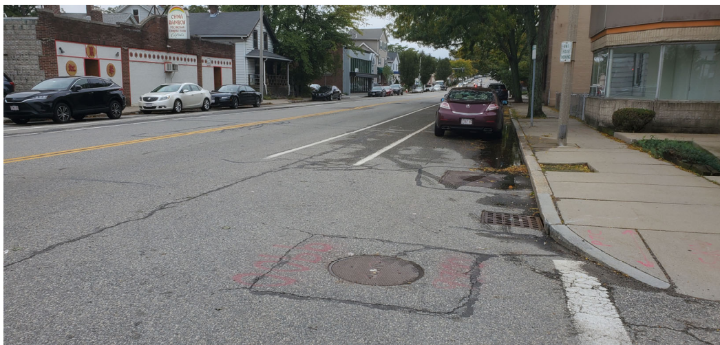
Photo 5: View of North Beacon Street facing East at Manhole #9900
