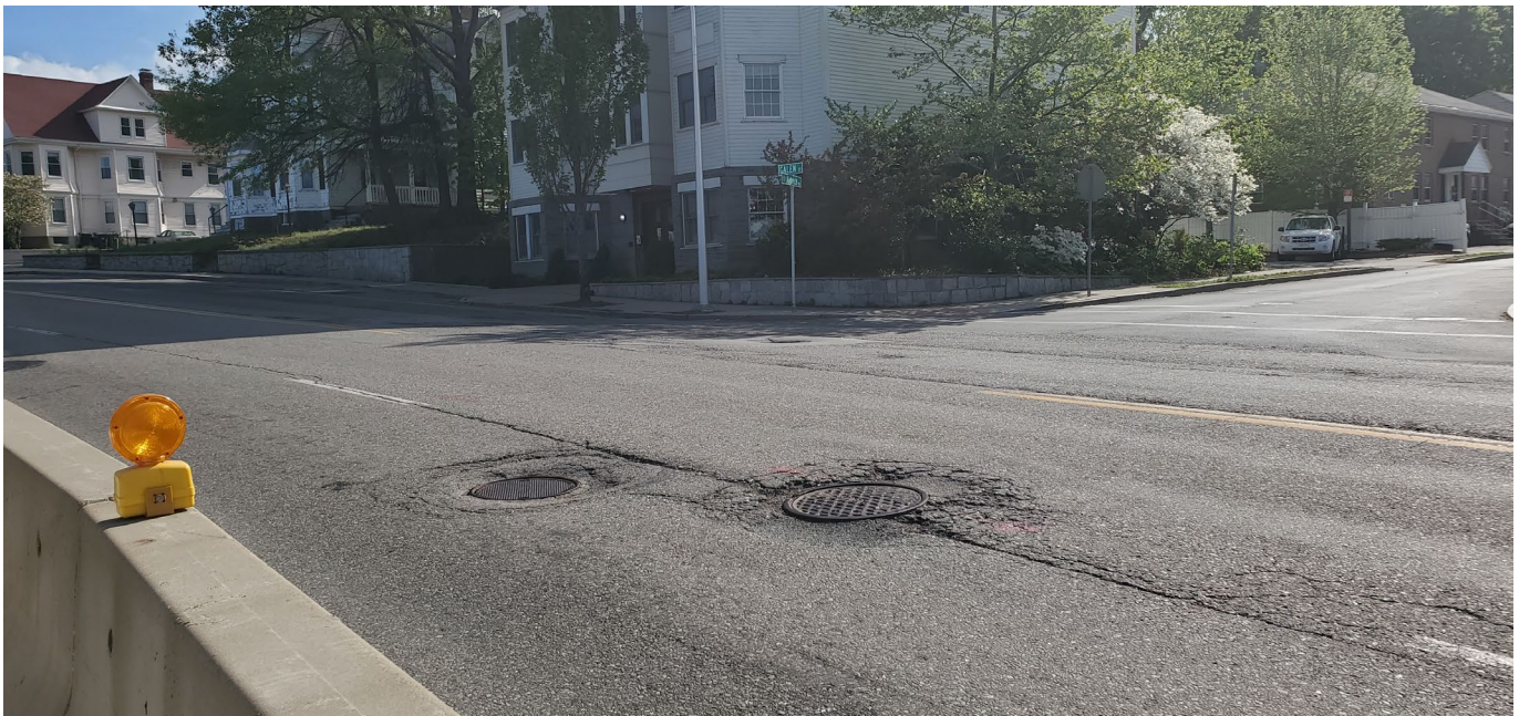
Photo 3: View of Galen Street facing South where the connection is proposed from manhole MH 16/205 to the 66 Galen Street Property.
