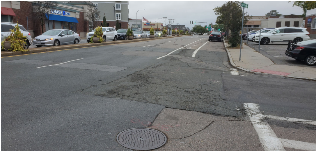
Photo 3: View of North Beacon Street facing East at location of Manhole #3700
