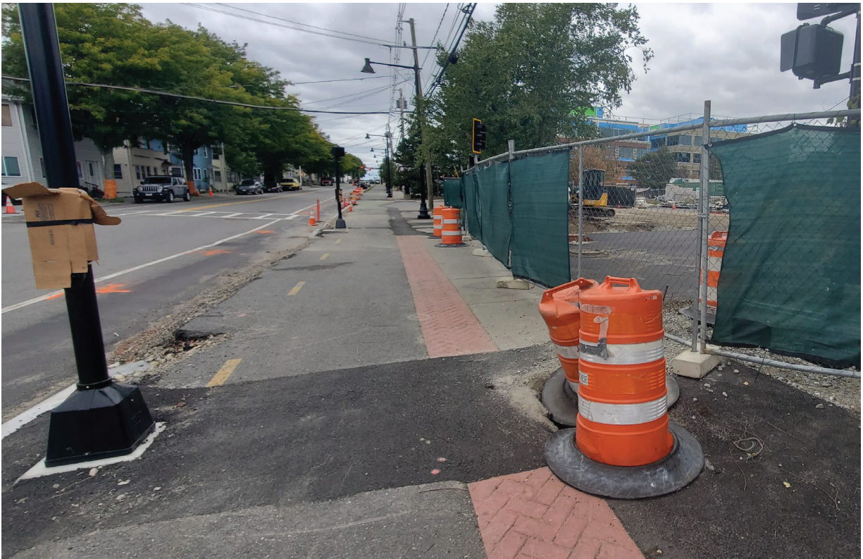
Photo 2: View of Arsenal Street facing West at location of proposed service connection (under construction barrels)
