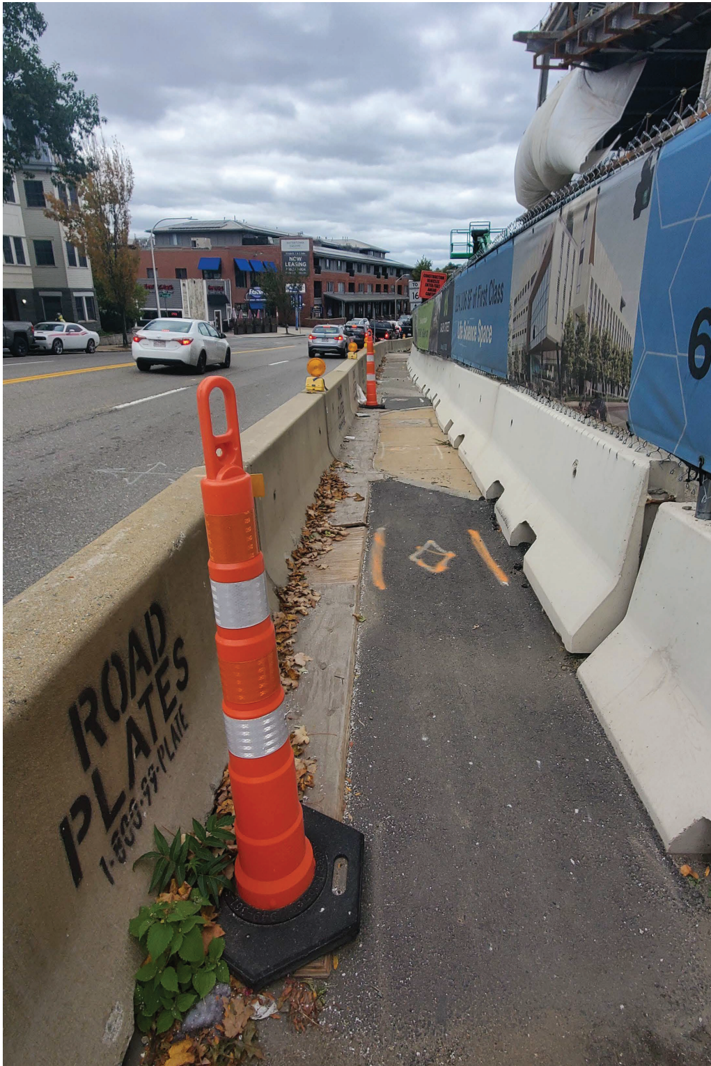
Photo 1: View of Galen Street facing North at location of proposed service connection
