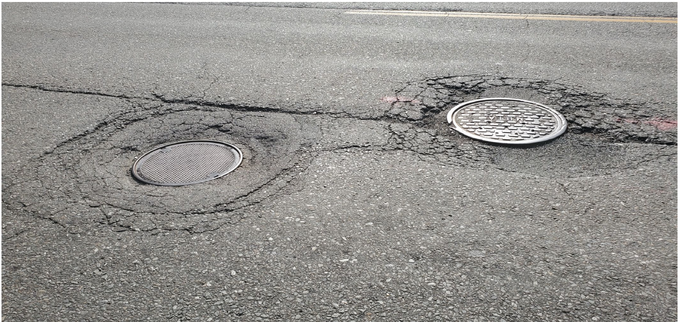
Photo 4: View of manhole MH 16/205.
