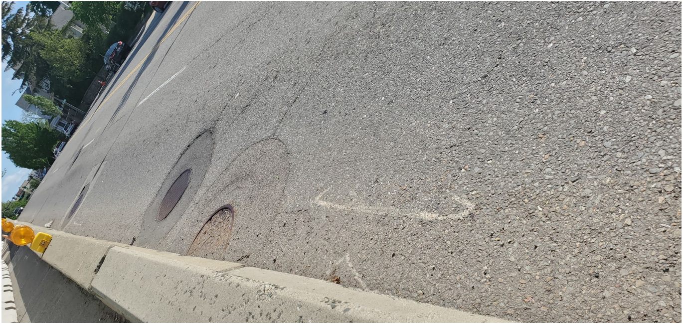
Photo 6: View of Galen Street facing South where manhole MH 16/205A is located.
