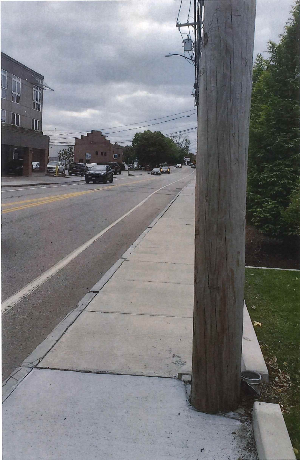
Photo 4: View of Pleasant Street facing West at location of utility pole #46
