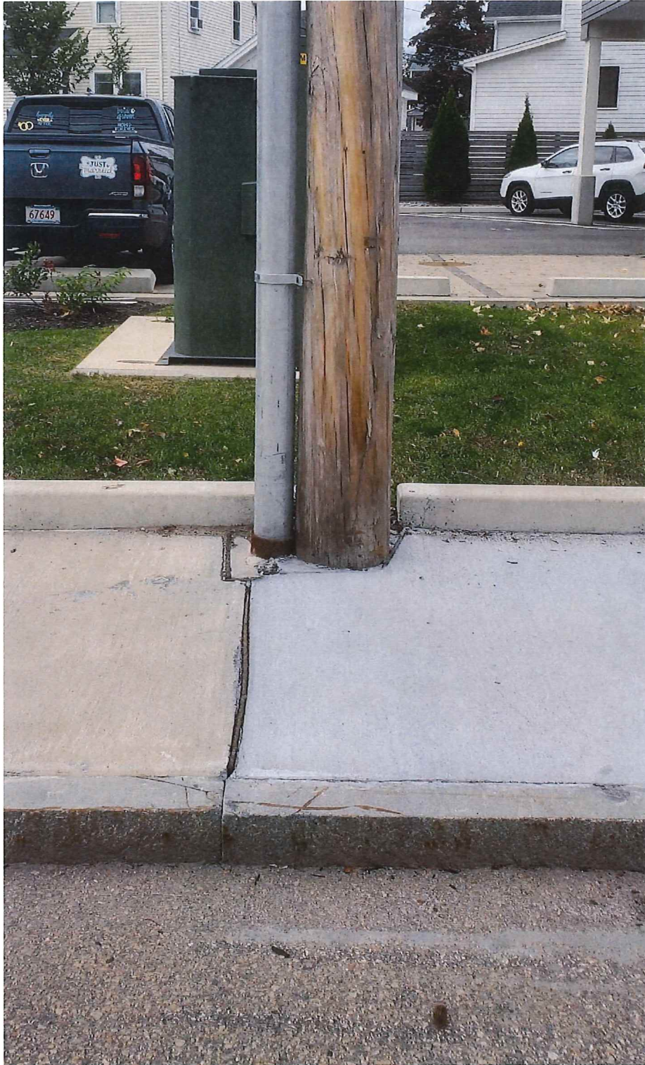
Photo 2: Pleasant Street view of utility pole #46
