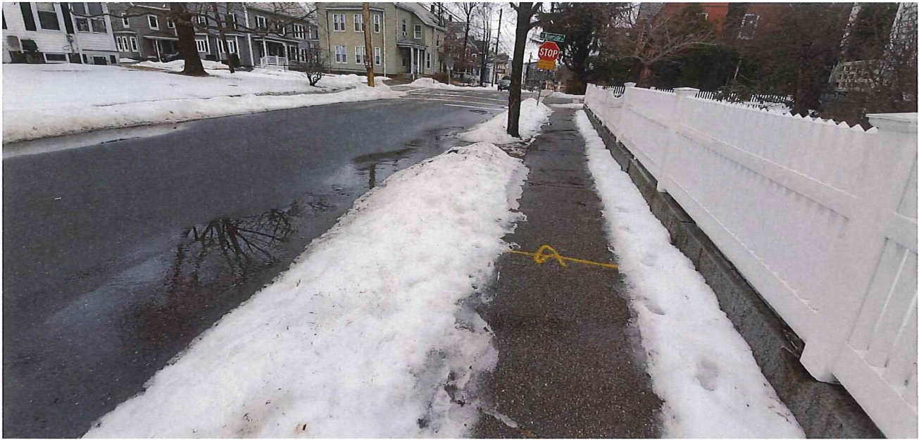
Photo 3: View of Irving Street facing Riverside Street where the road has recently been repaved.
