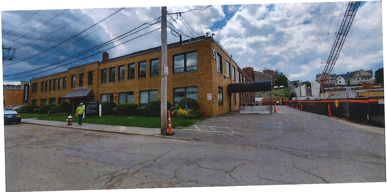
Photo 1: View of Utility Pole 142/6 and 51 Water Street.
