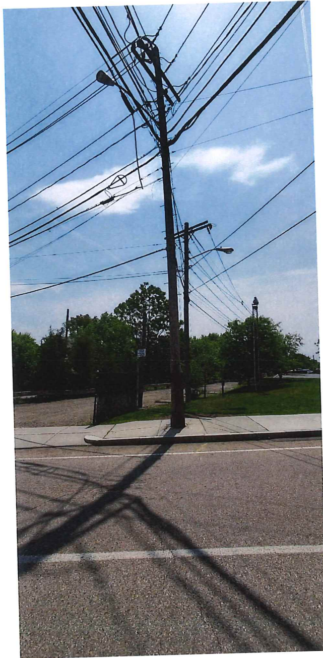
View of the proposed location of connection from utility pole #100/1 to the existing conduit located within the roadway.
