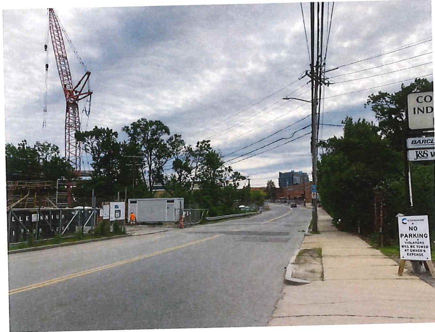
Photo 3: View of Coolidge Avenue facing Arsenal Street where the proposed conduit and manhole will be installed.
