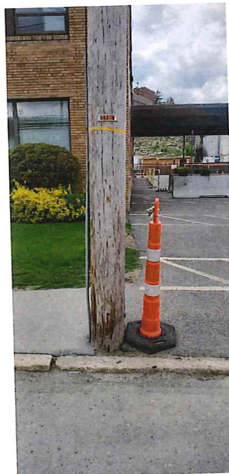
Photo 2: View of Utility Pole 142/6.
