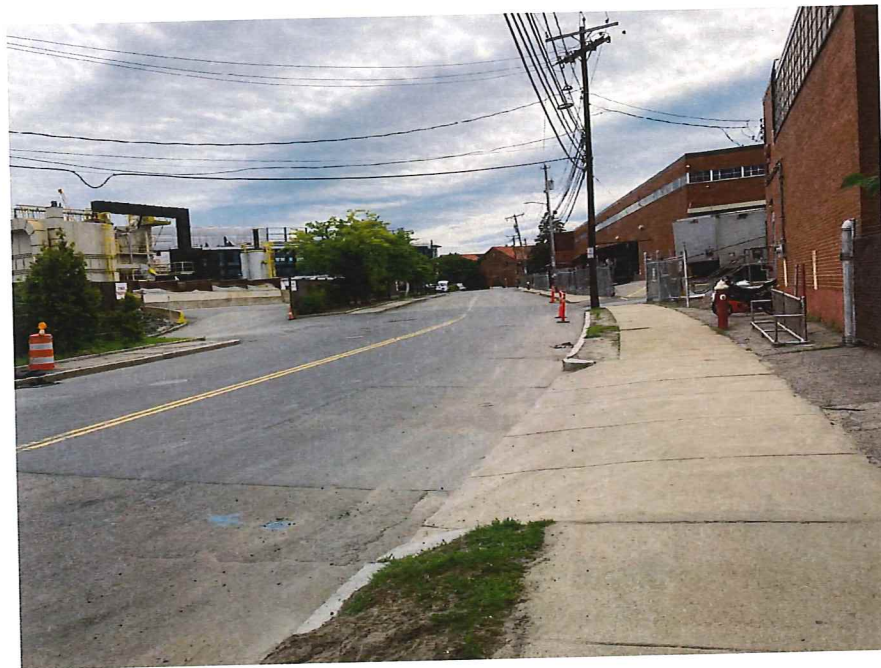
Photo 4: View of Coolidge Ave facing Arsenal Street where the proposed conduit and manhole will be installed.
