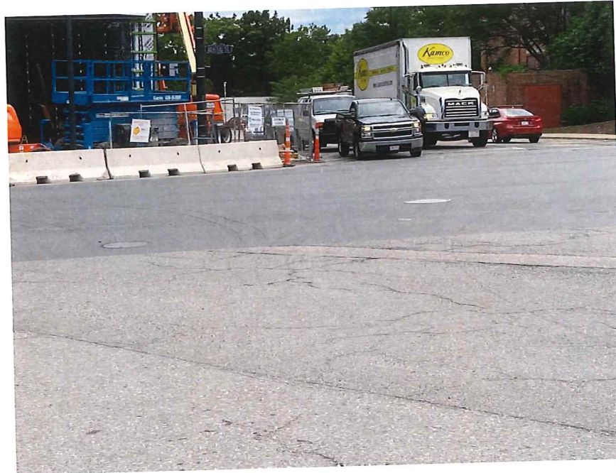
Photo 1: Location of connection to manhole MH15899 in Arsenal Street by Forge Road and Coolidge Avenue.
