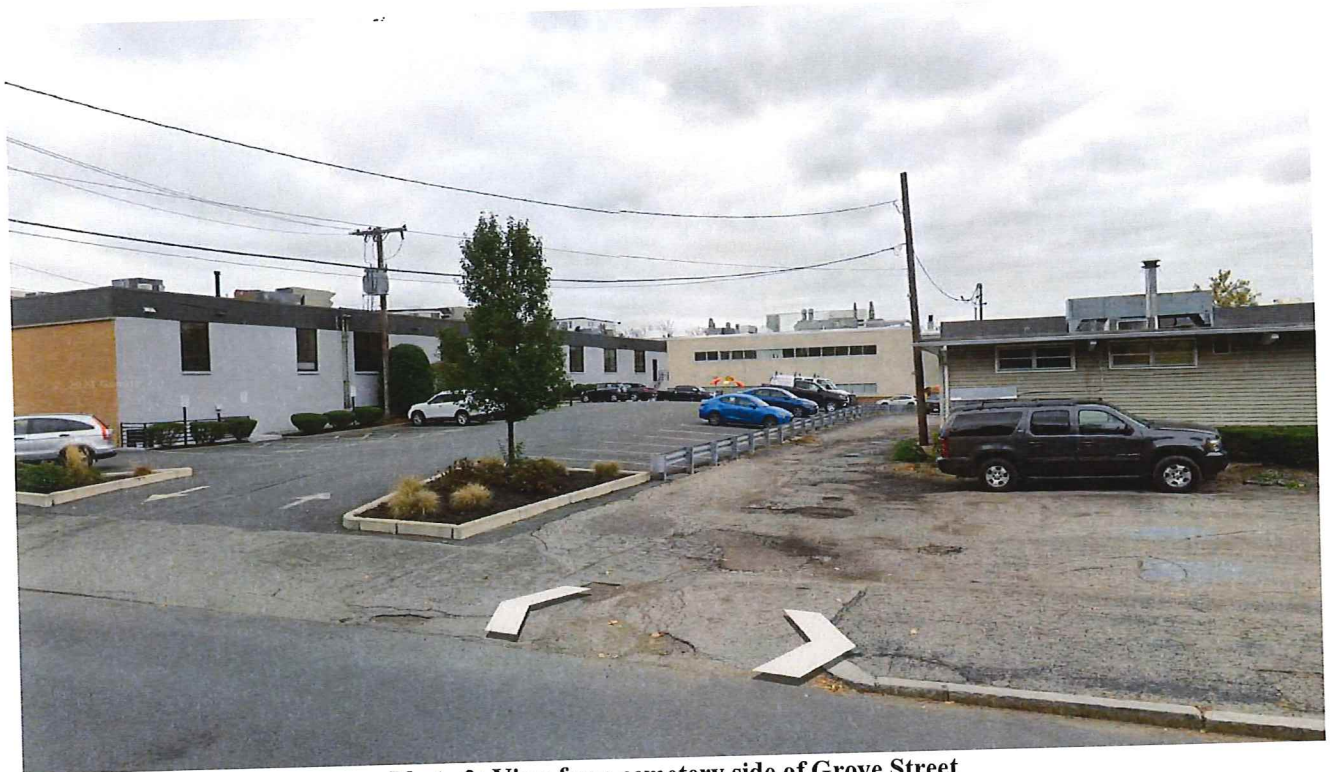
Photo 2: View from cemetery side of Grove Street
