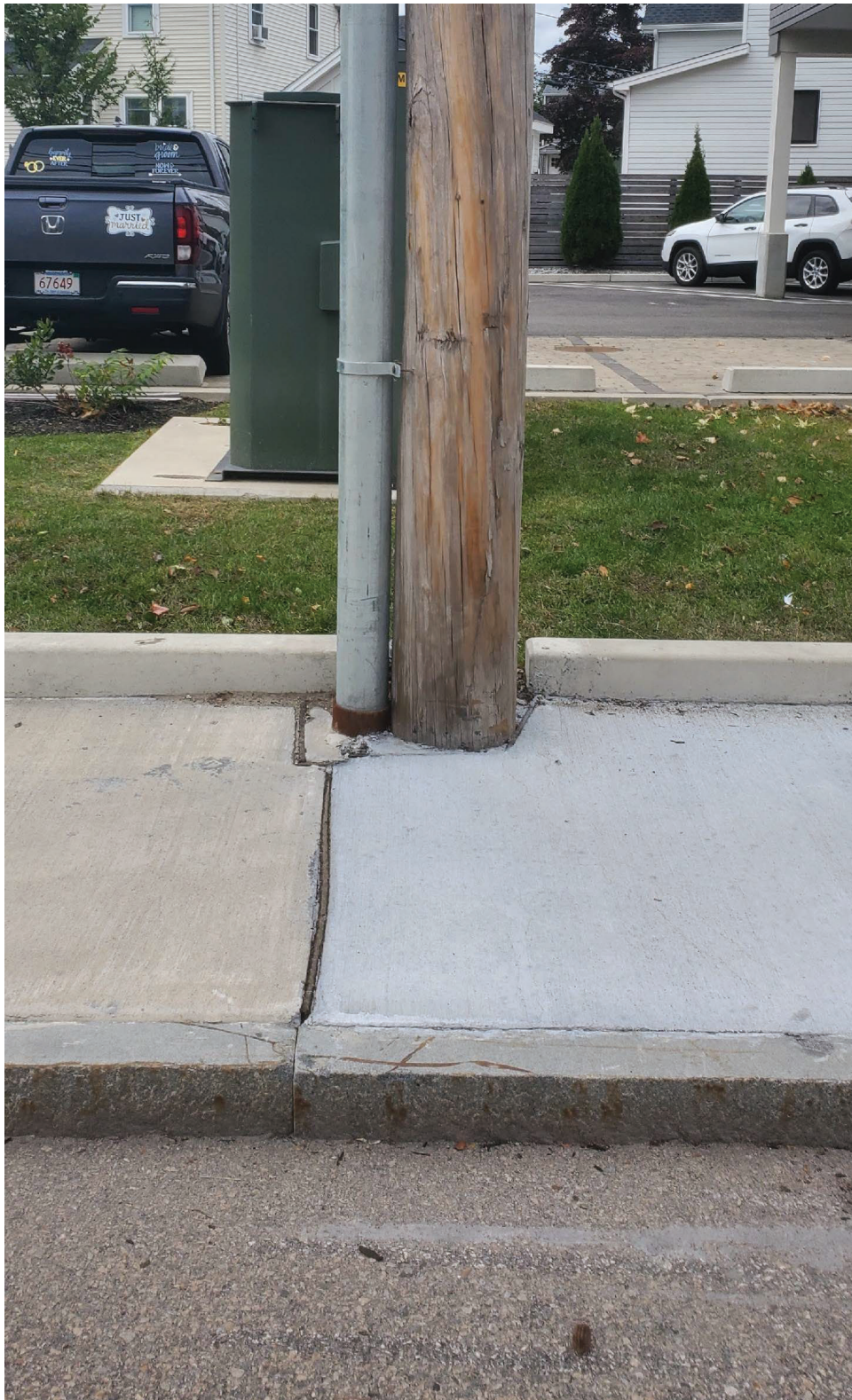
Photo 2: Pleasant Street view of utility pole #46
