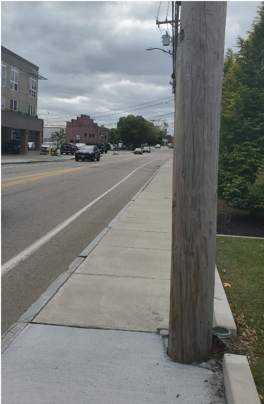
Photo 4: View of Pleasant Street facing West at location of utility pole #46
