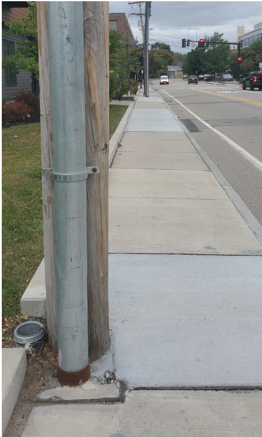
Photo 3: View of Pleasant Street facing East at location of utility pole #46
