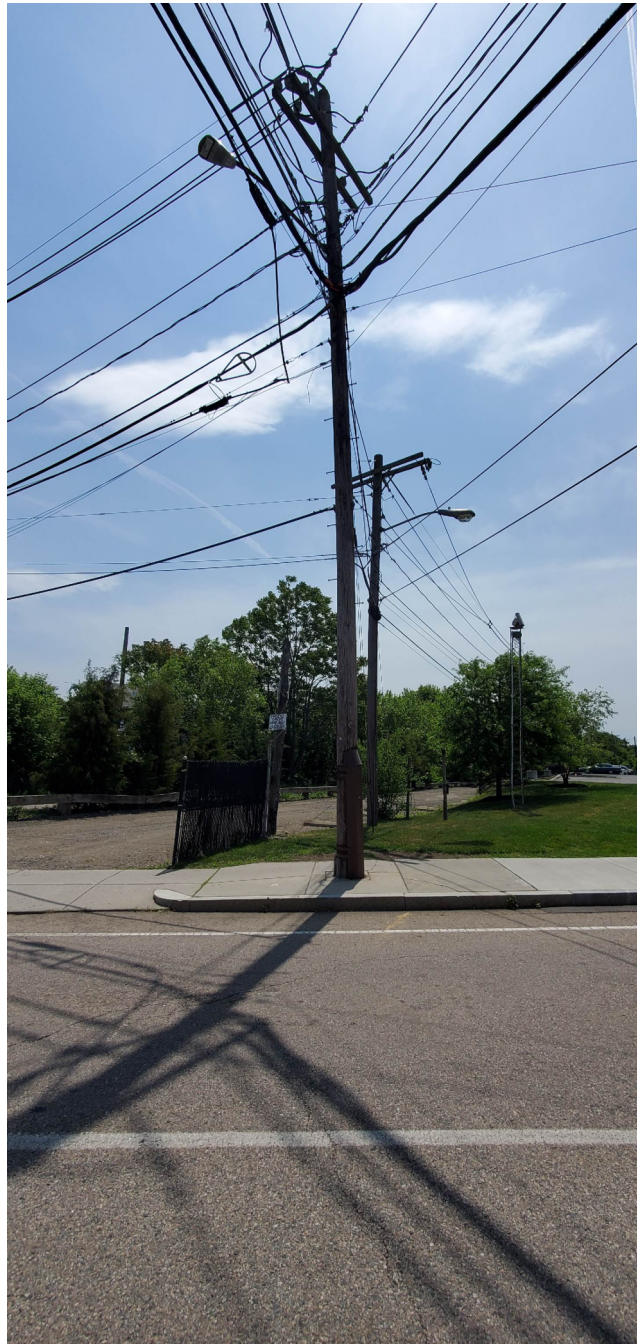
View of the proposed location of connection from utility pole #100/1 to the existing conduit located within the roadway.
