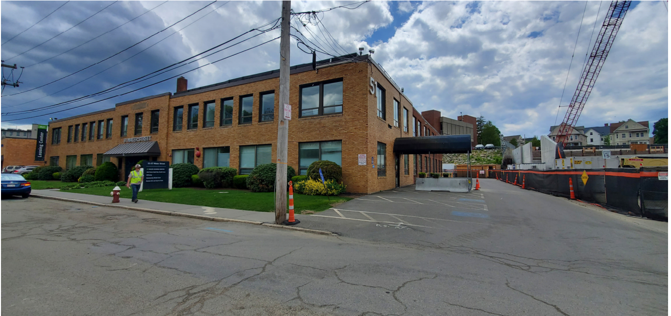
Photo 1: View of Utility Pole 142/6 and 51 Water Street.
