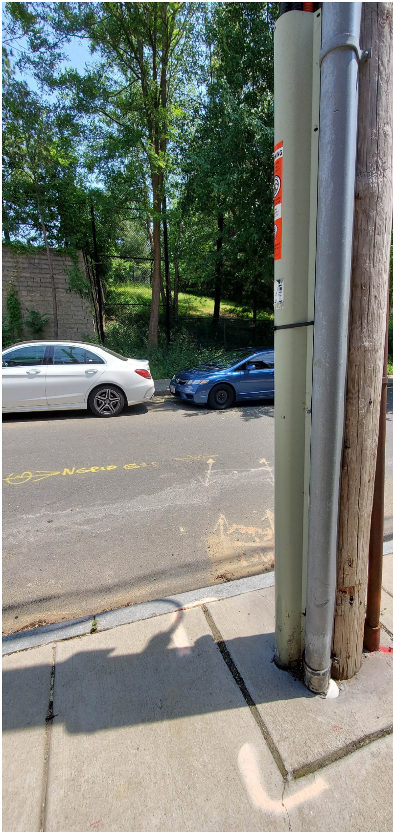
View of utility pole #11 and the proposed connection location facing the location of the existing data center located at 486 Arsenal Way.
