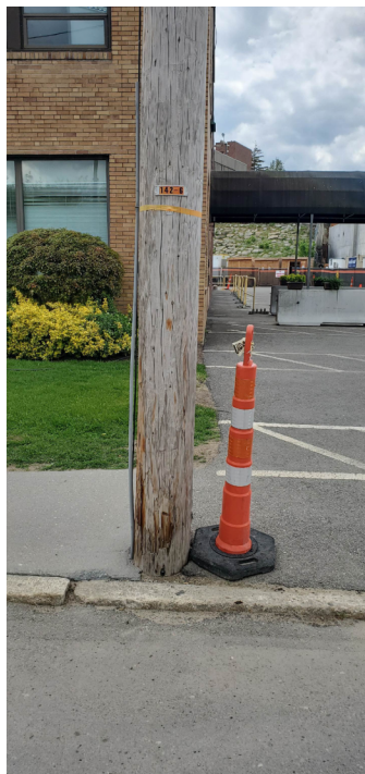
Photo 2: View of Utility Pole 142/6.
