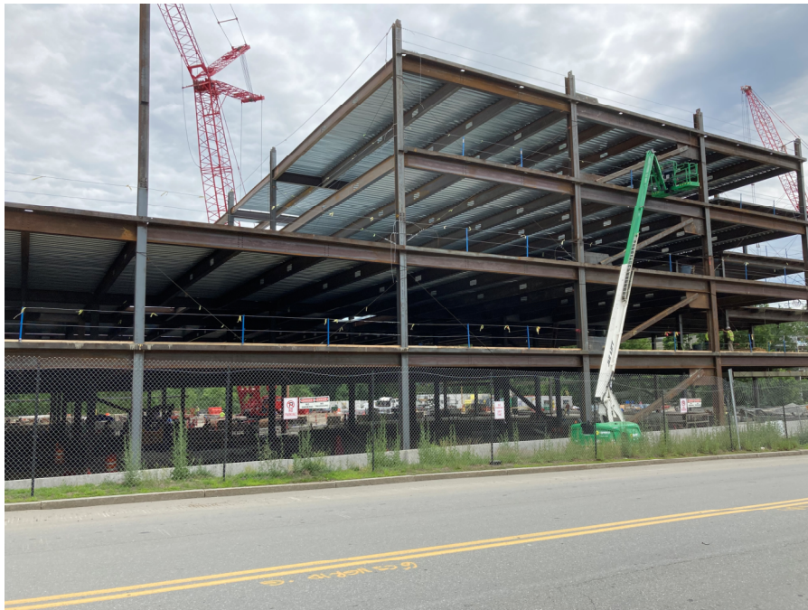
Photo 2: View of ongoing construction at the location where the proposed connection to 99 Coolidge Avenue.
