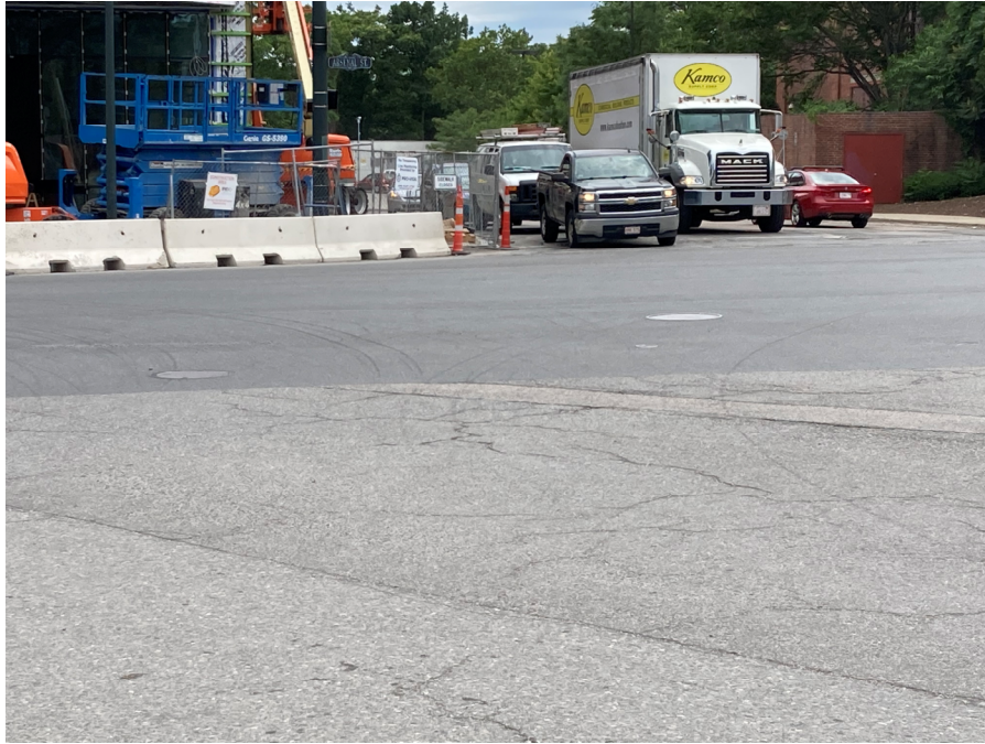
Photo 1: Location of connection to manhole MH15899 in Arsenal Street by Forge Road and Coolidge Avenue.
