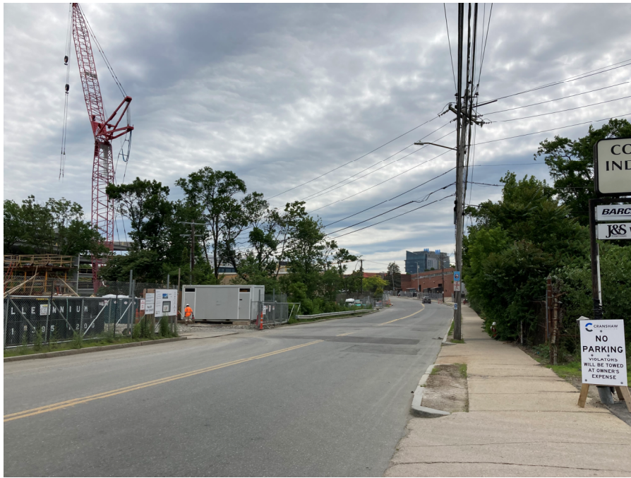
Photo 3: View of Coolidge Avenue facing Arsenal Street where the proposed conduit and manhole will be installed.
