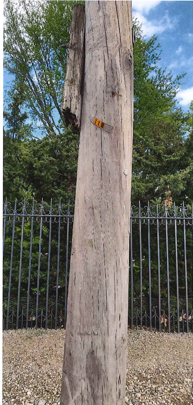
Photo 2: View of Utility Pole ID 63/18.
