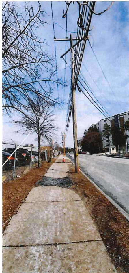
View of Utility Pole 32/11 and sidewalk facing east-northeast.
