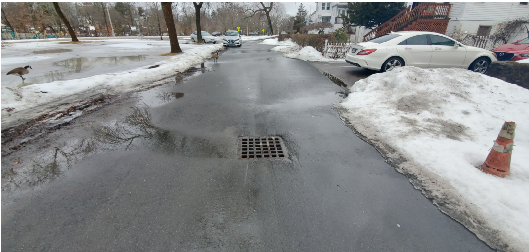
Photo 8: View of Private Way and catch basin closer to Irving Street.
