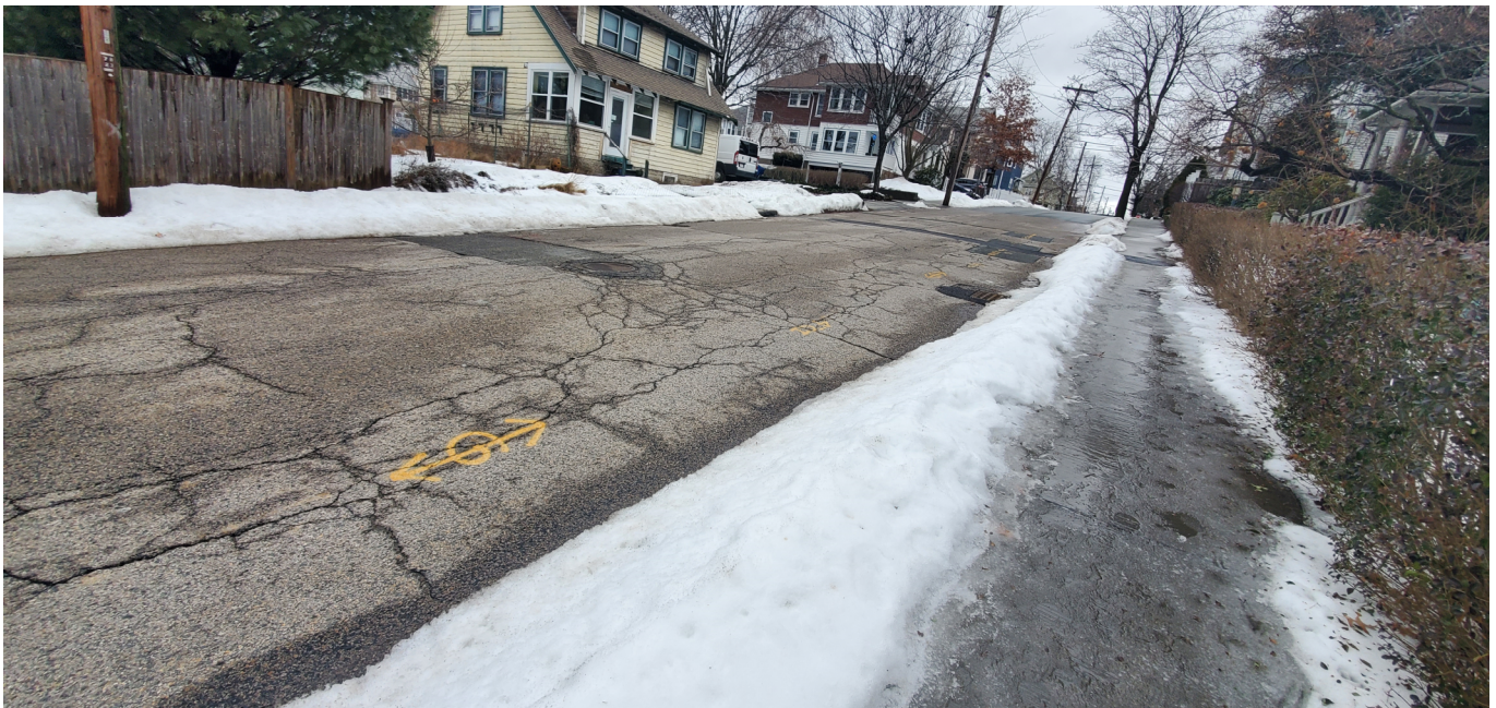
Photo 6: View of Irving Street facing Riverside Street closer to the Private Way where the proposed gas main will be relayed to provide service to the residences along the Private Way.
