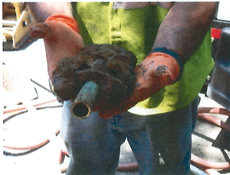
Quincy lead removal project
