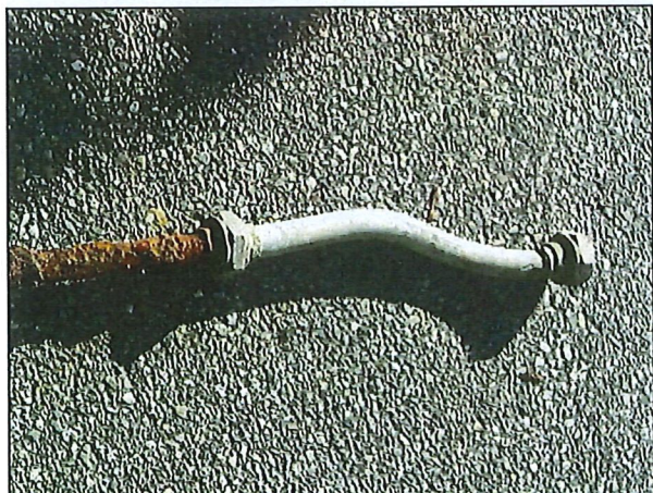
Photo of lead gooseneck connected to iron pipe (Source: Wikipedia)
