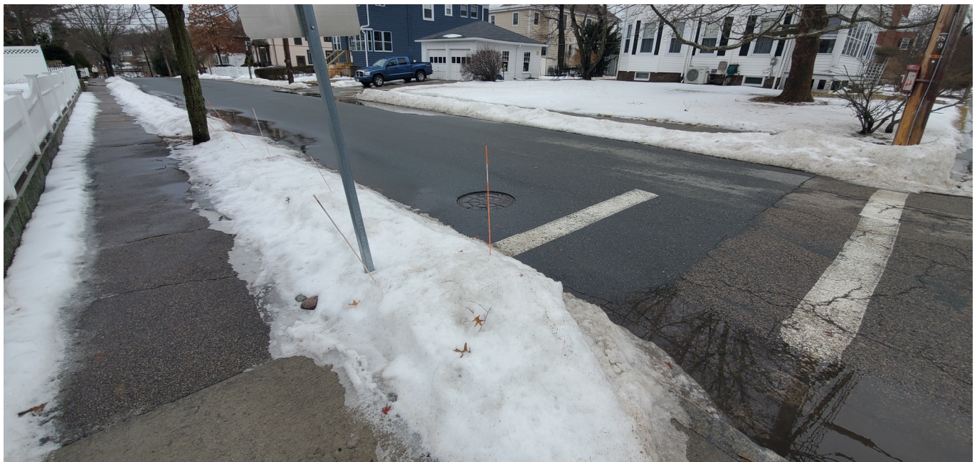
Photo 2: View of Irving Street where the road has recent been repaved.
