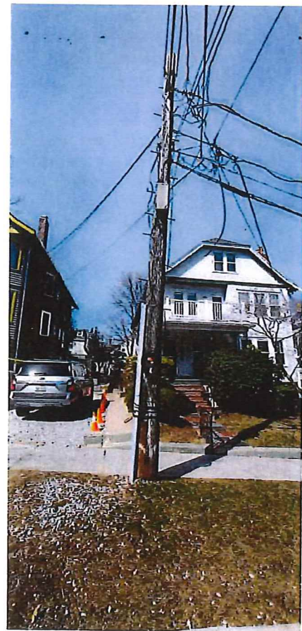
View of entire utility pole 178.
