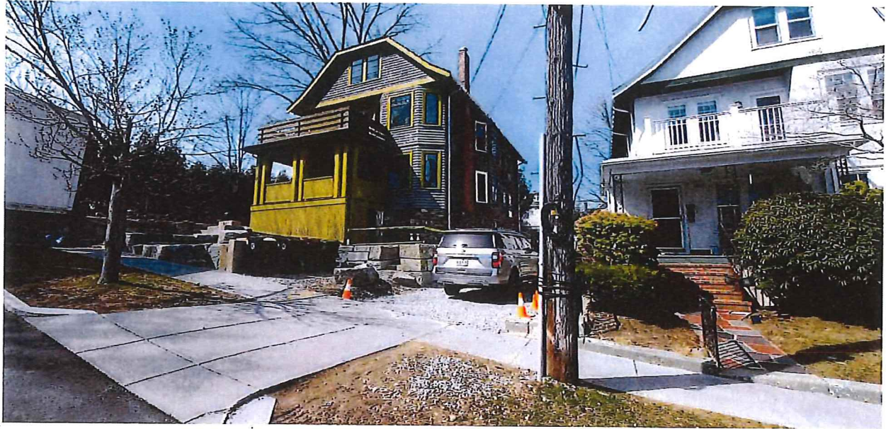
View of 23 Alden Road and utility pole 178 facing southwest where the service connection is proposed.
