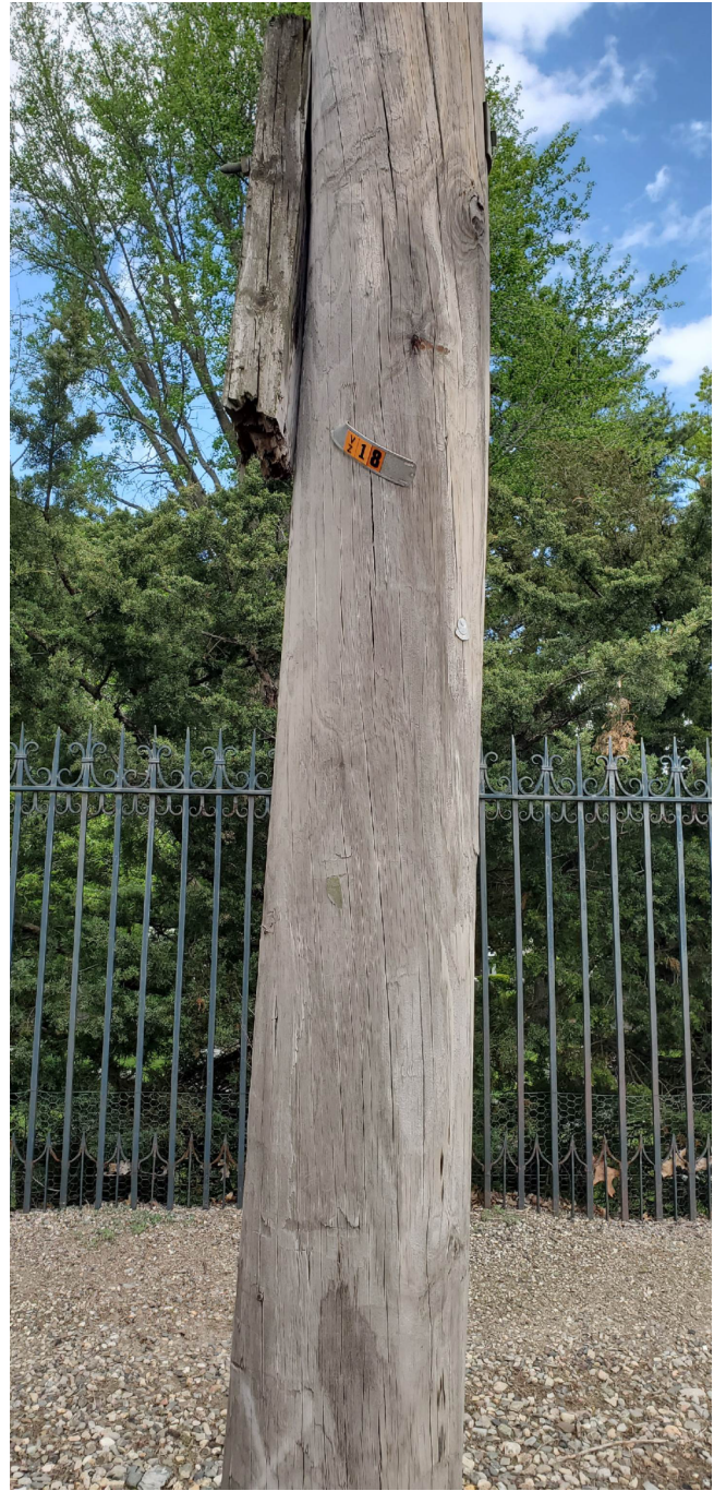
Photo 2: View of Utility Pole ID 63/18.
