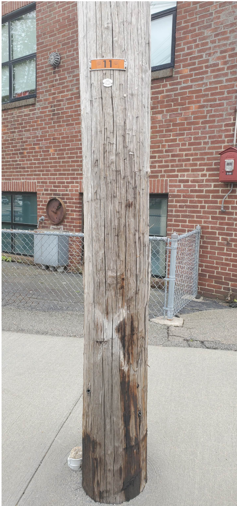
Photo 2: View of Utility Pole #194/11
