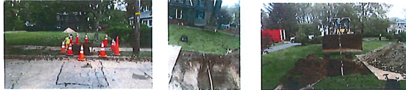
Long lead service line replacement in Newton
