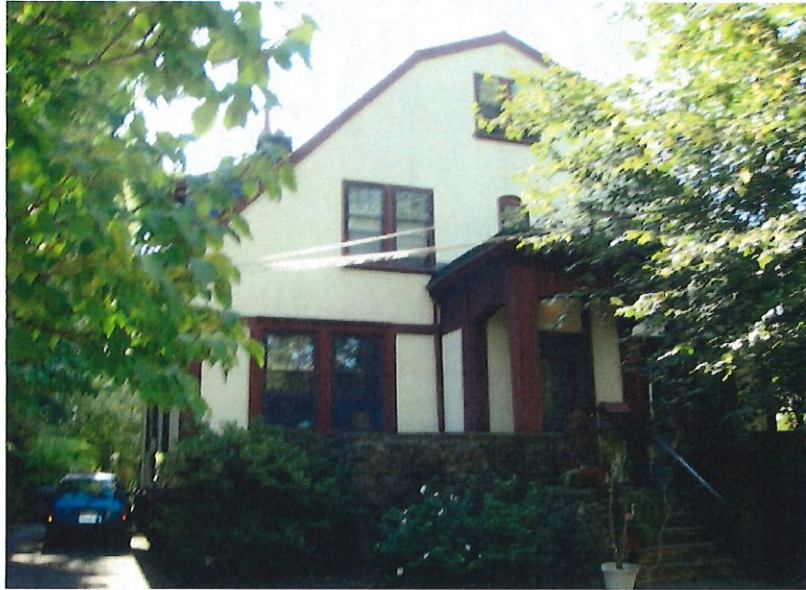
Before installation of new windows
