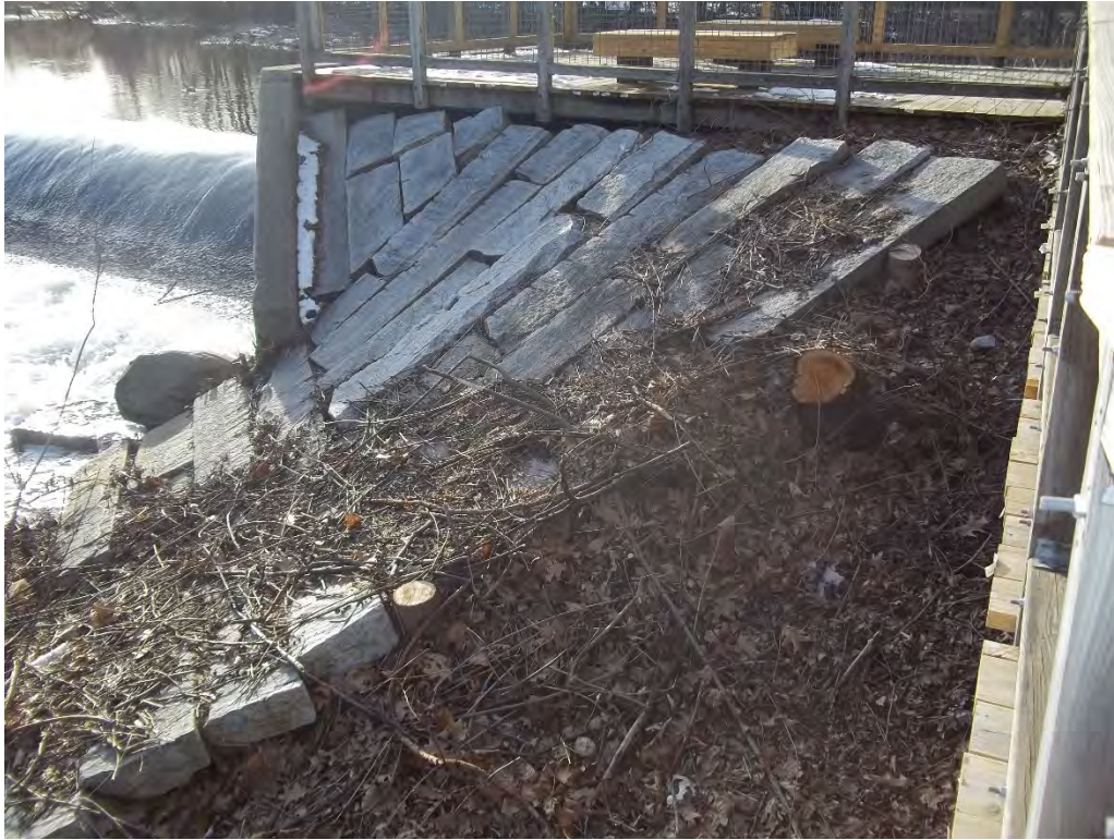
Photo 11. Downstream slope of left embankment.
