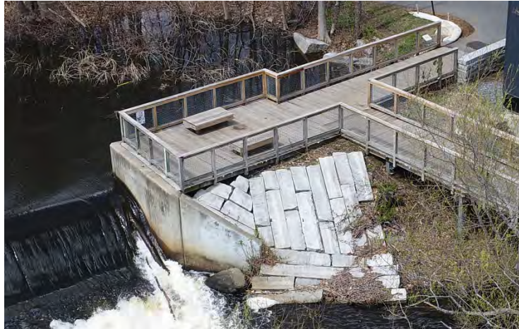
FIGURE 6-4 DCR Overlook No. 1 Near Sasaki Building at Eastern Abutment of Watertown Dam Near 64 Pleasant Street, Watertown, Massachusetts
