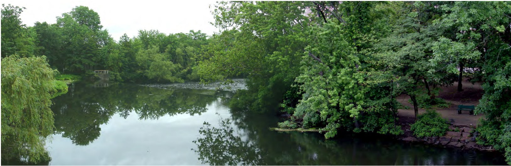
Photo 1 – Dam weir and right bank from upstream footbridge*
