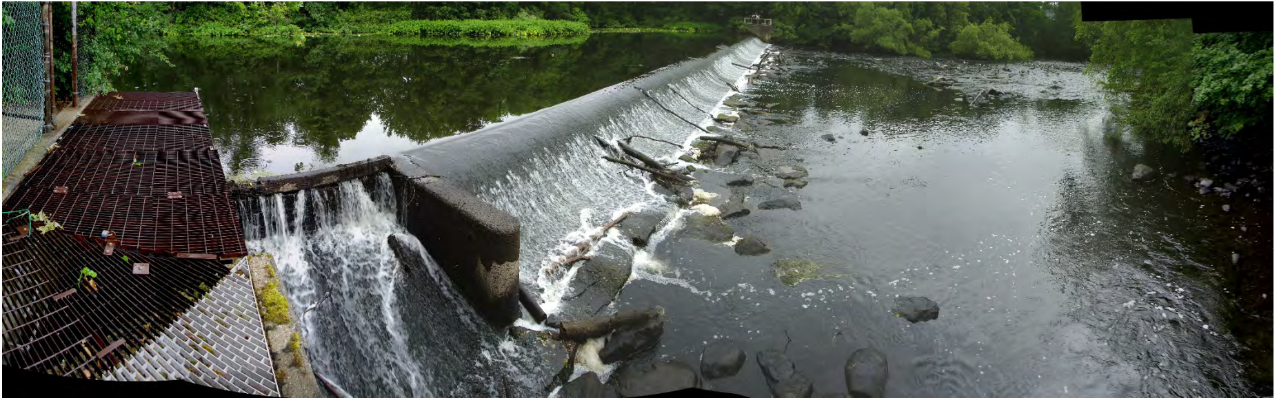
Photo 5 – Sluice / stop log gate and spillway weir / dam crest from right abutment fish ladder platform *
