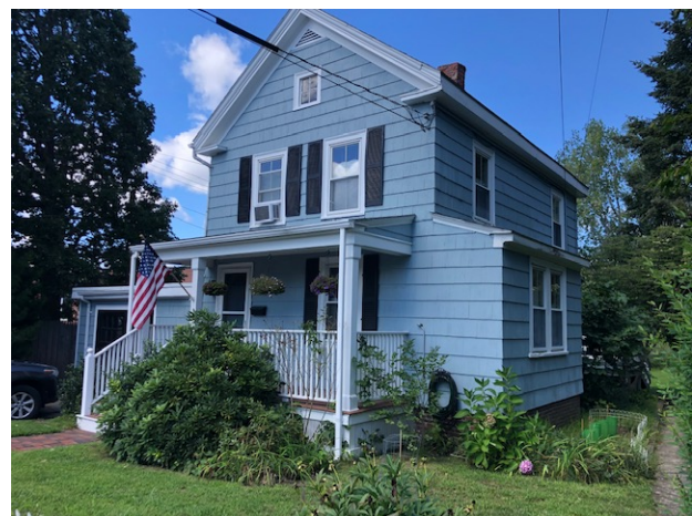
Northwesterly view of dwelling from California Street
