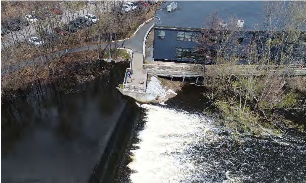
Photo No. 5: Aerial photo of river-left (northern) training wall, with a pedestrian walkway observation deck and former mill building. April 2018
