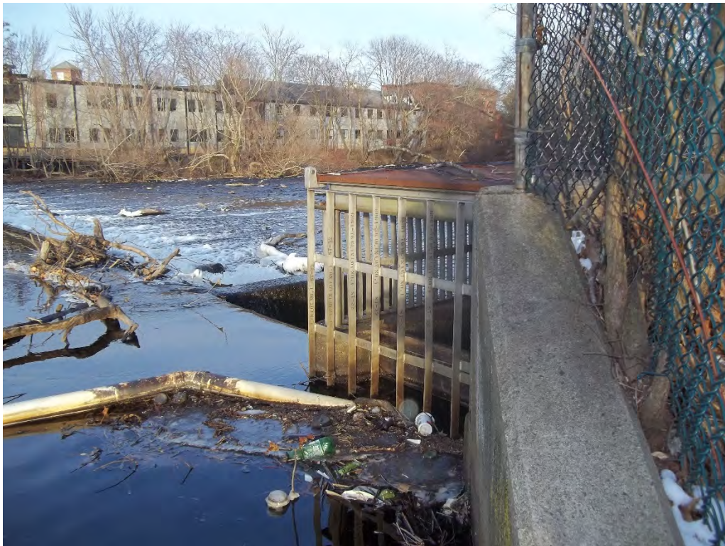
Photo 2. Fish ladder exit (upstream end) at right abutment.
