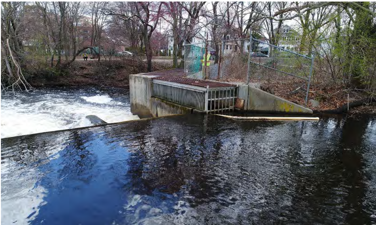
Photo No. 3: River-right (southern) training wall, concrete fish ladder looking at upstream end (fish exit). April 2018
