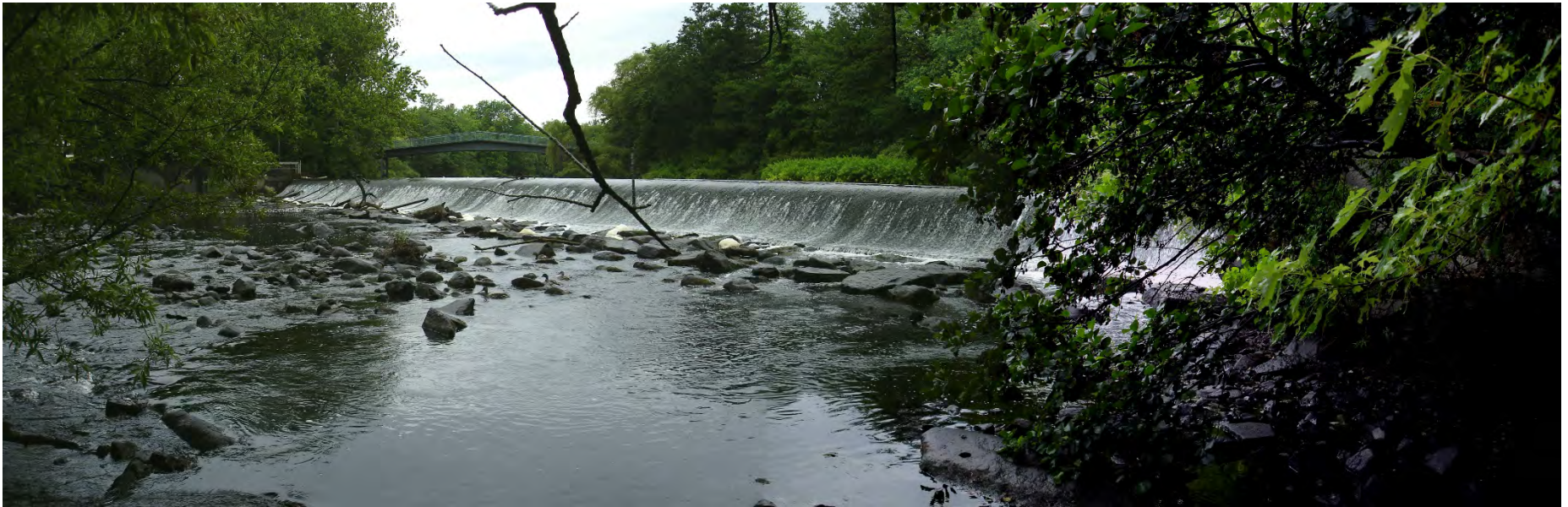
Photo 7 – Dam / spillway from downstream left riverbank*
