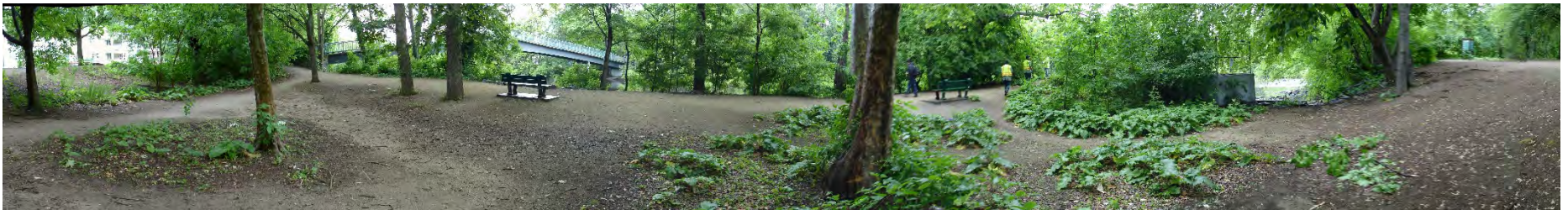
Photo 8 – Right abutment, looking toward the river*
