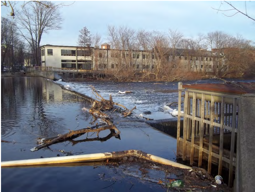
Photo 1. Dam / spillway weir and fish ladder exit from right abutment.
