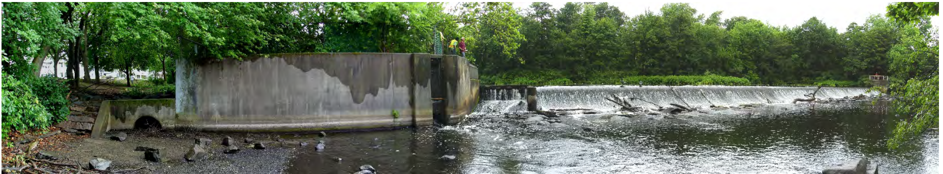
Photo 6 – Right abutment, fish ladder, sluice / stop log gate, and spillway / dam from downstream right riverbank*
