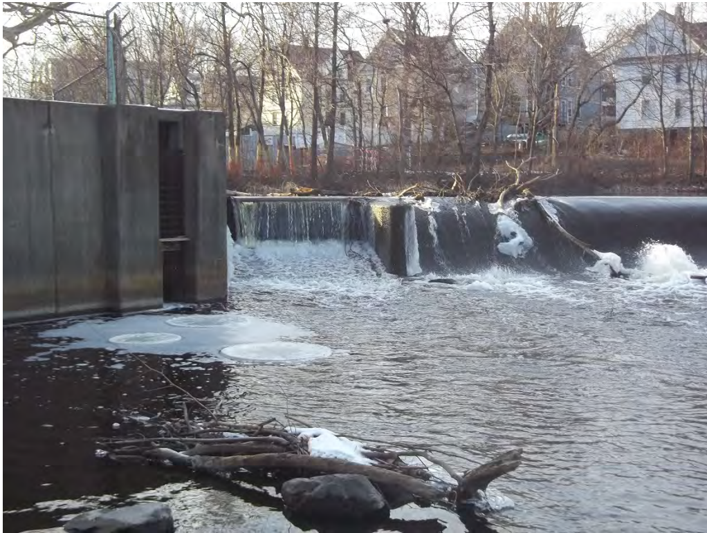
Photo 5. Fish ladder entrance and stop log bay on right side.
