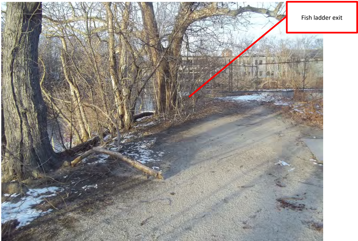
Photo 8. Upstream "levee" on right bank.
