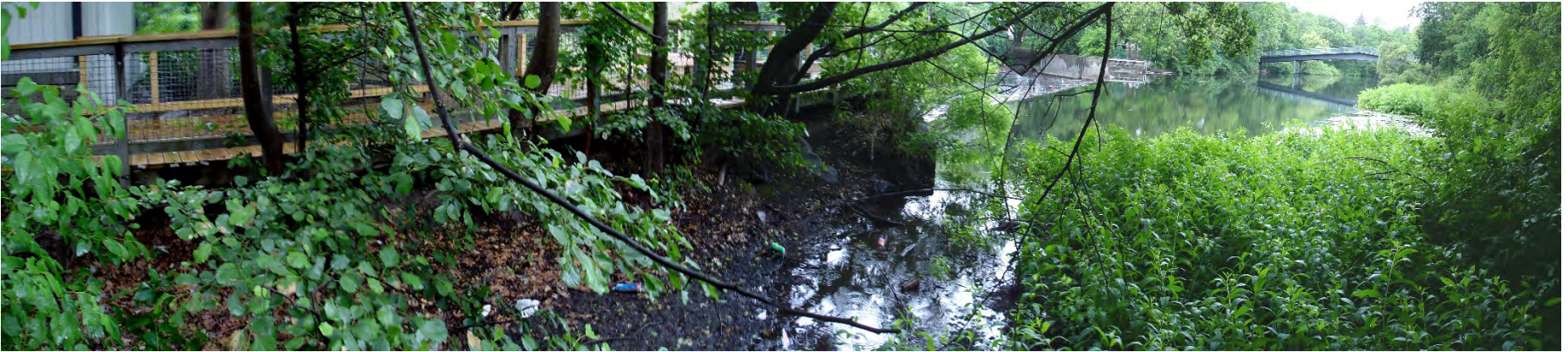
Photo 3 – Left abutment, spillway weir, and upstream channel from upstream left riverbank*
