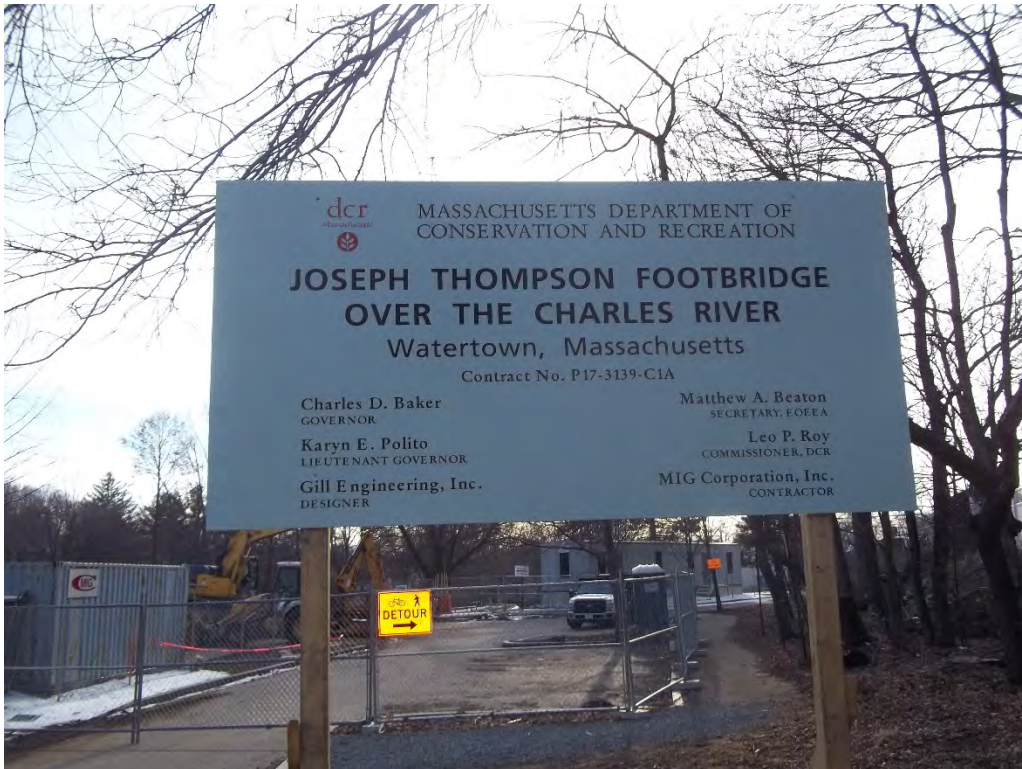
Photo 13. Construction sign for the upstream bridge replacement project.
