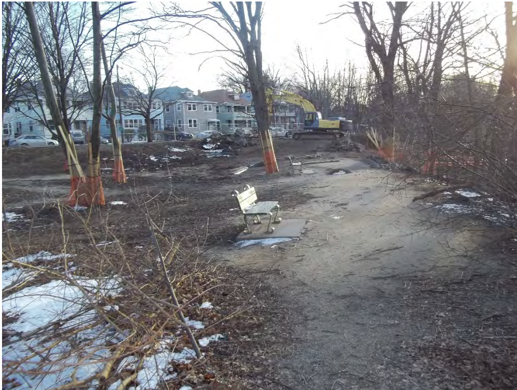
Photo 13. Right upstream embankment “levee” (note construction).
