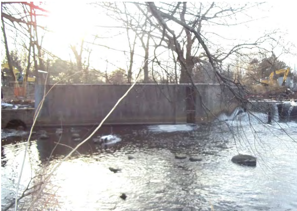
Photo 6. Downstream face of fish ladder structure and culvert discharge.
