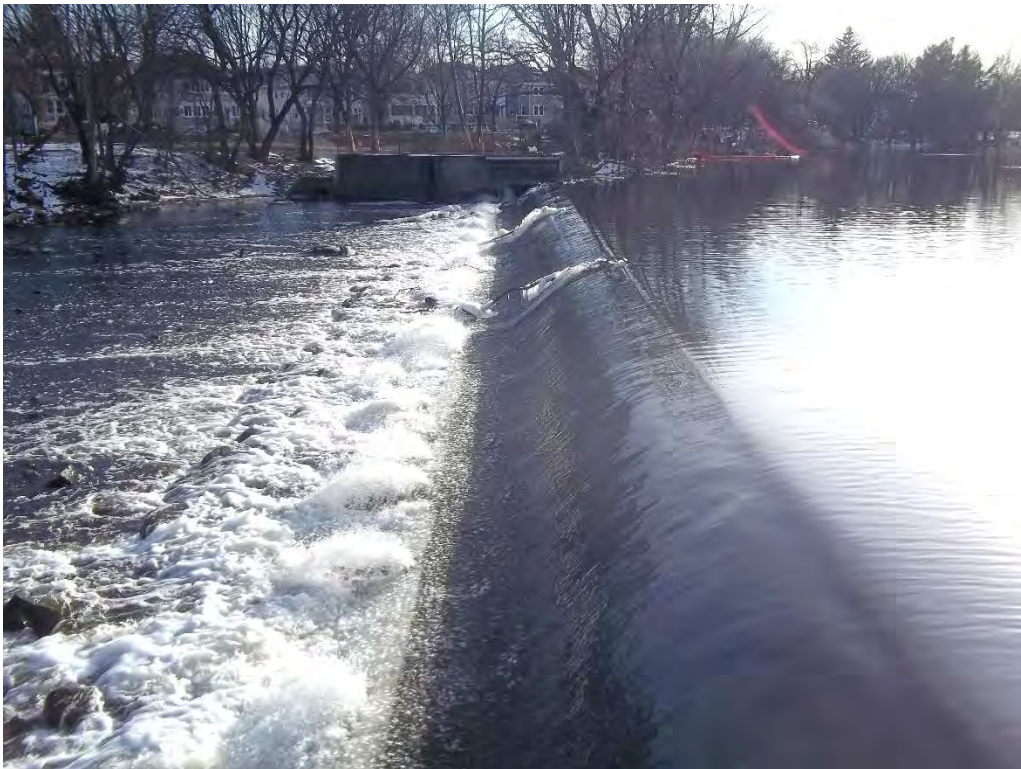
Photo 4. Spillway weir from platform on left embankment.
