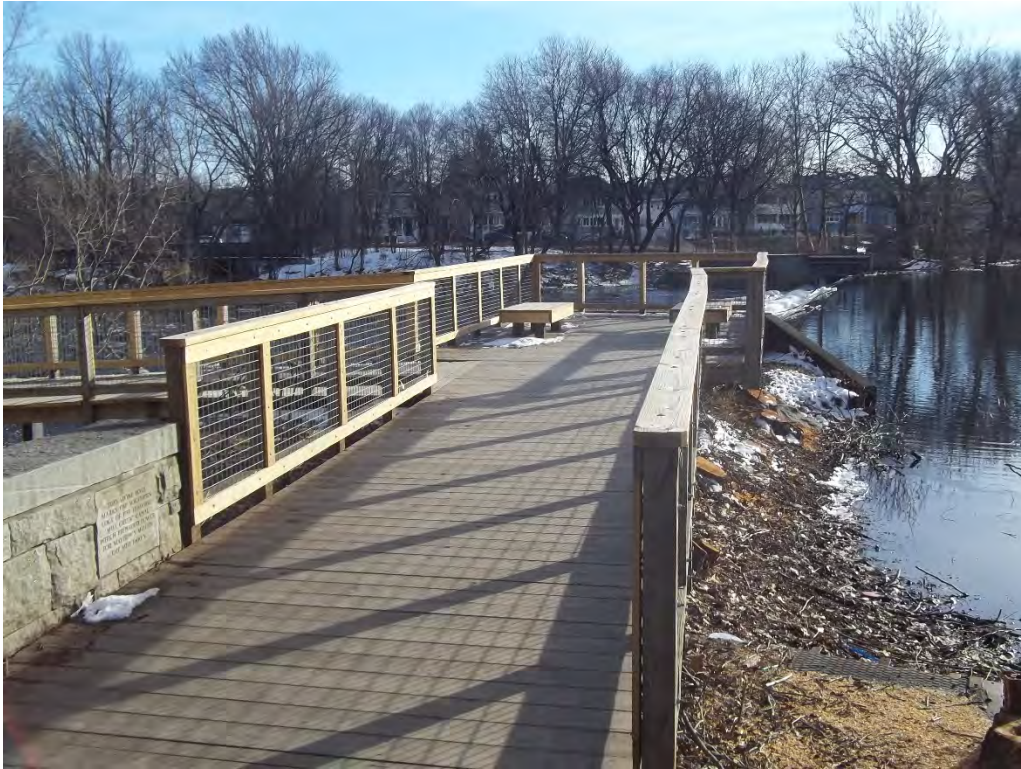
Photo 3. Overview of left embankment and u/s slope from abutment.
