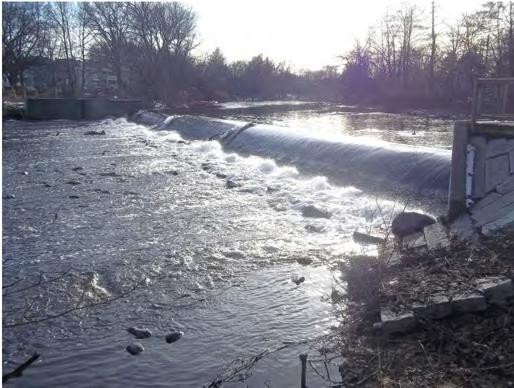
Photo 7. Dam / spillway weir from downstream left bank.
