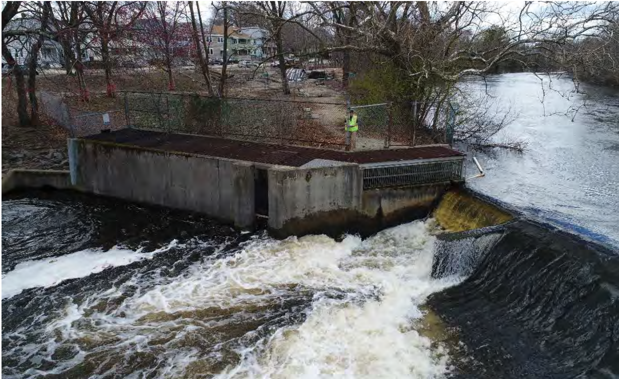
Photo No. 3: River-right (southern) training wall, concrete fish ladder looking at upstream end (fish exit). April 2018
