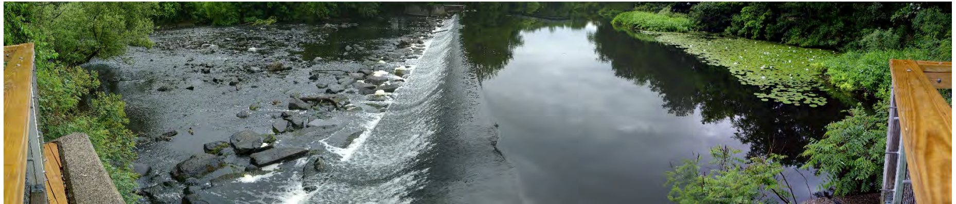
Photo 4 – Spillway weir / dam crest from left abutment walkway*
