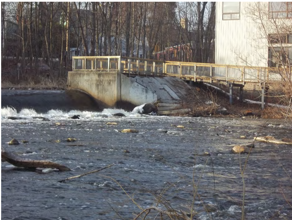
Photo 10. Downstream face of left embankment.
