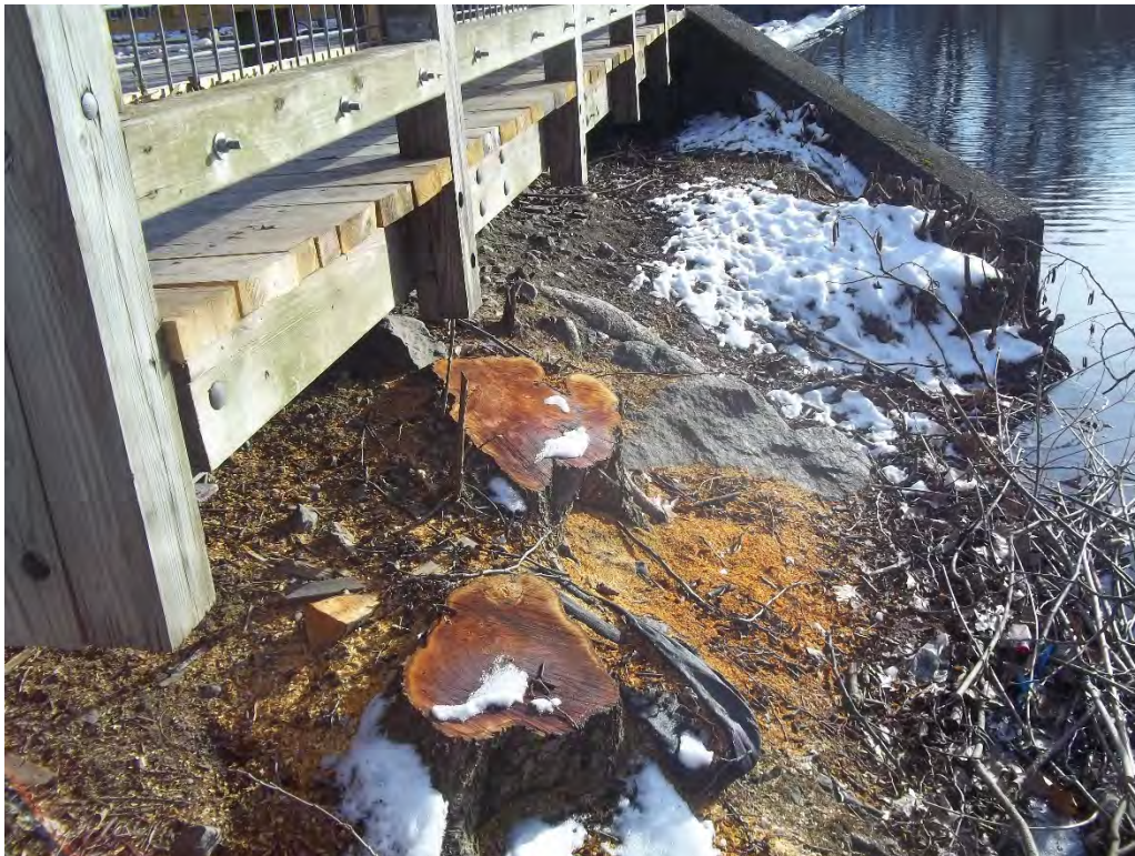
Photo 12. Upstream slope of left embankment / abutment (note stumps).
