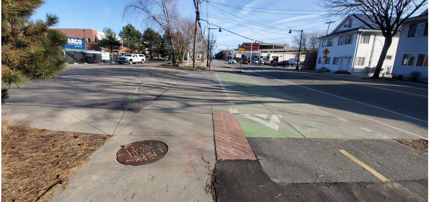
View of proposed connection point location, manhole MH10727, in the northern sidewalk on Arsenal Street facing East.
