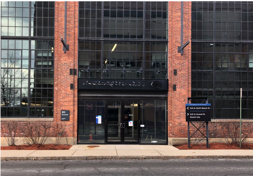
FLAG SIGN STRUCTURE AT 311
