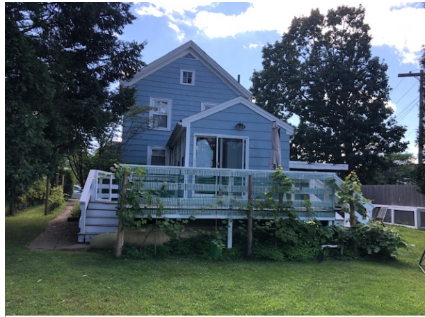
Southerly view of rear of dwelling
