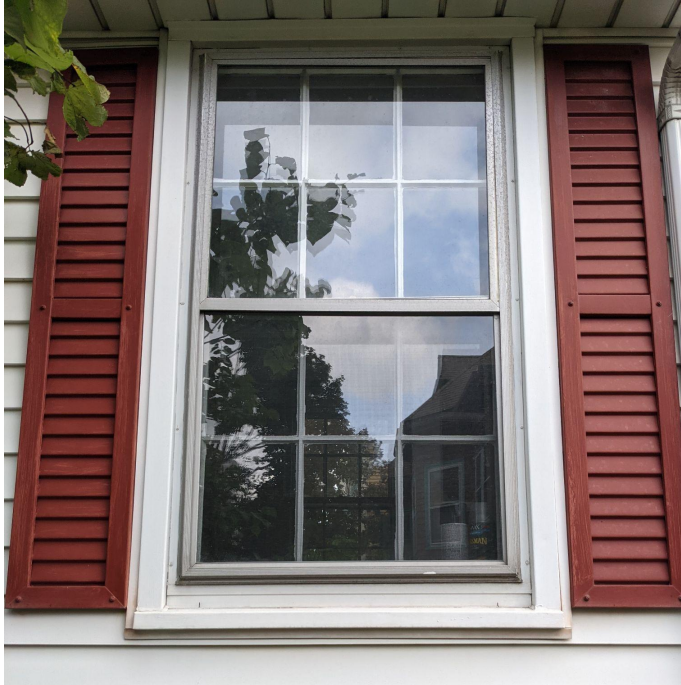
Existing Window 6-Light
