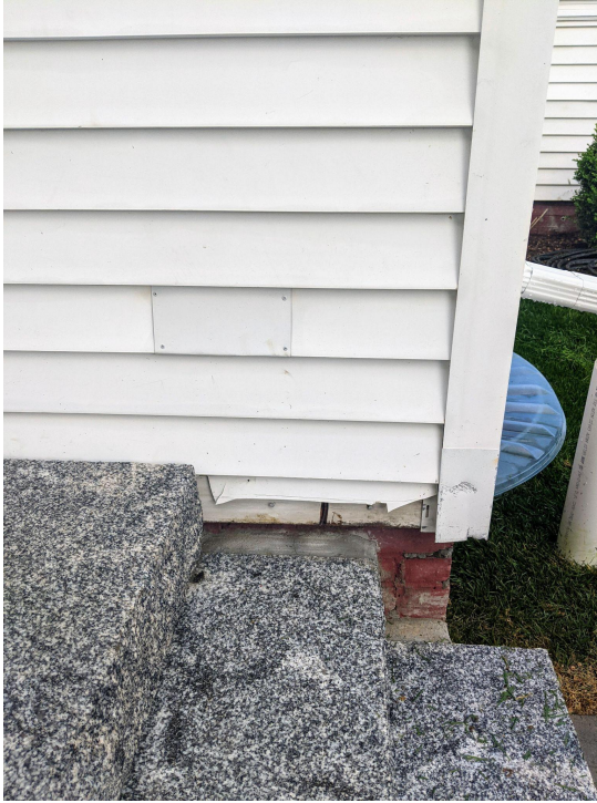
Photos of the current siding on the house.
