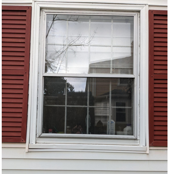
Existing Window 8-Light
