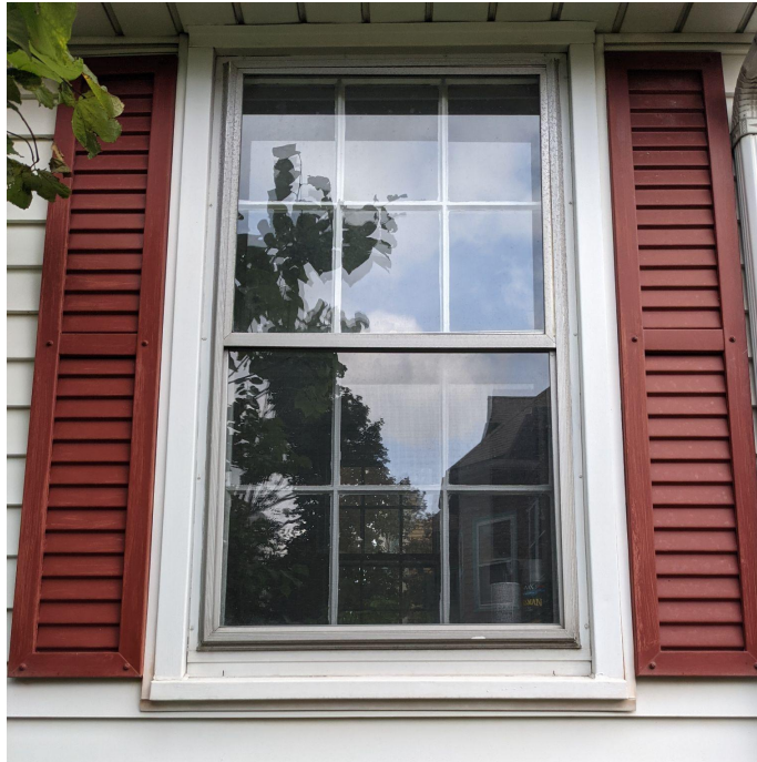
Existing Window 6-Light
