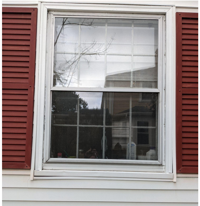
Existing Window 8-Light
