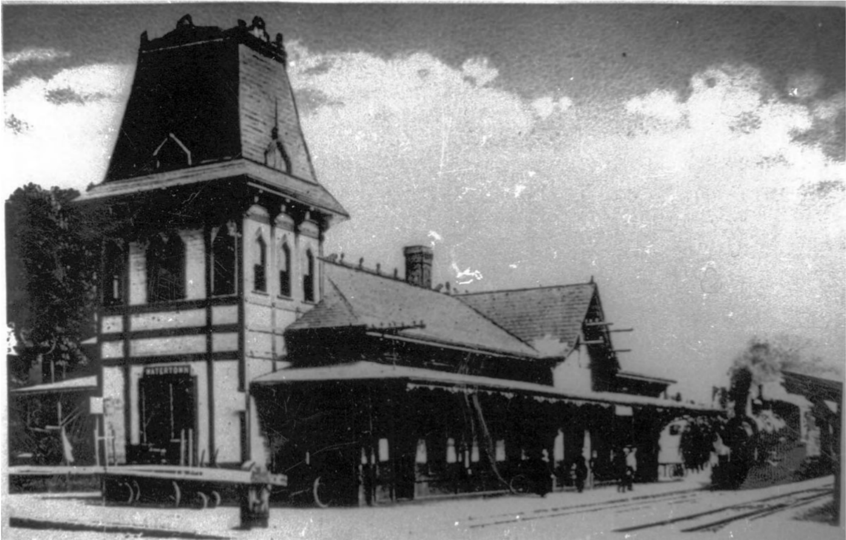
Figure 14: Watertown Station c.1890-1899
