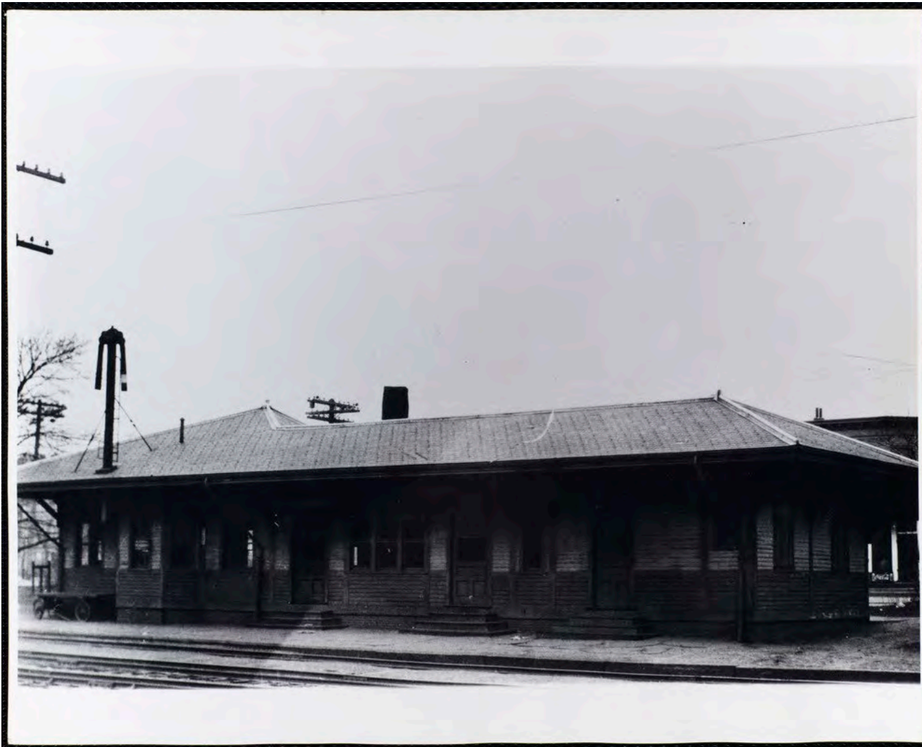
Figure 15: Watertown Station (c.1900-1960)
