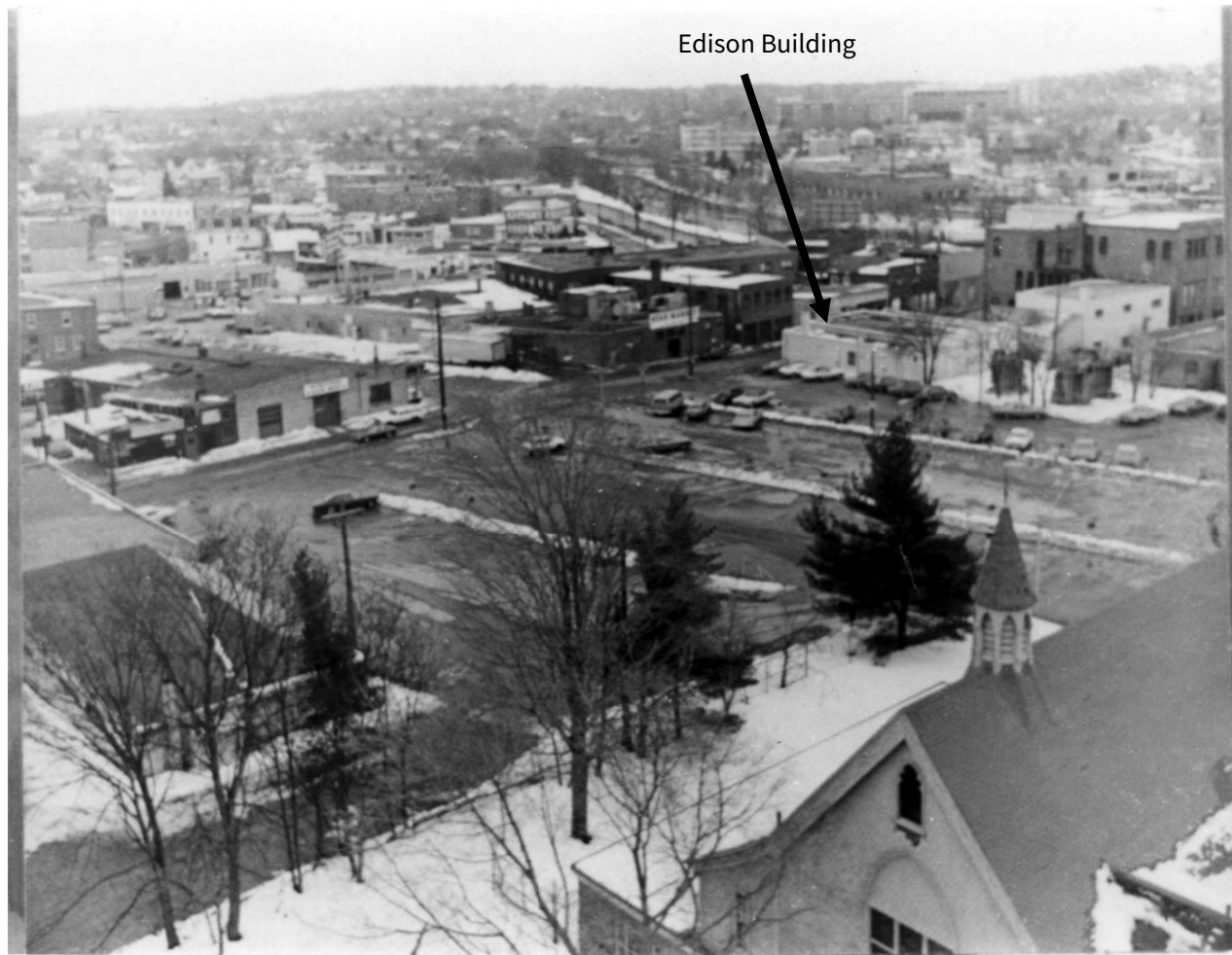
Figure 20: View of Parking Lots c.1975 29
