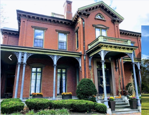
Commander's Mansion Building Exterior and Elevator Modernization
